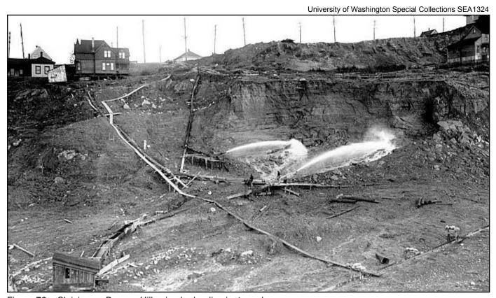
Figure 76 • Sluicing on Beacon Hill using hydraulic giants, n.d.
