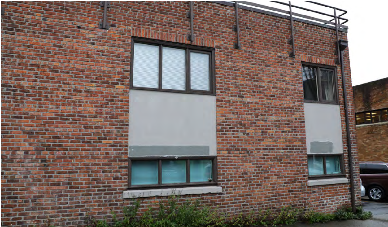
Figure 31. West facade showing the southwest portion.
