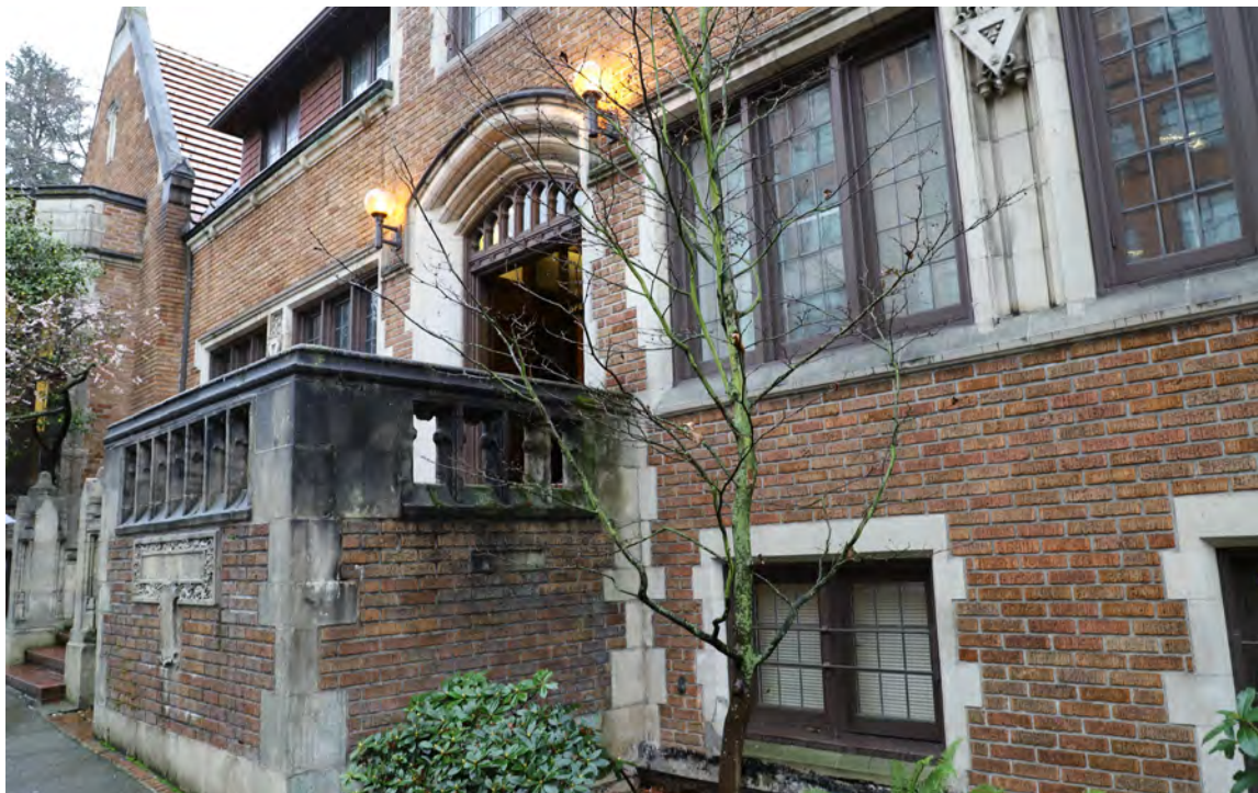
Figure 38. Main north entrance looking southeast.
