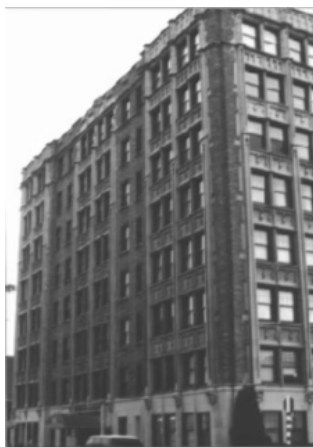
Figure 67. University Manor, 1305 NE 43rd St, designed by Earl Roberts, 1926.
