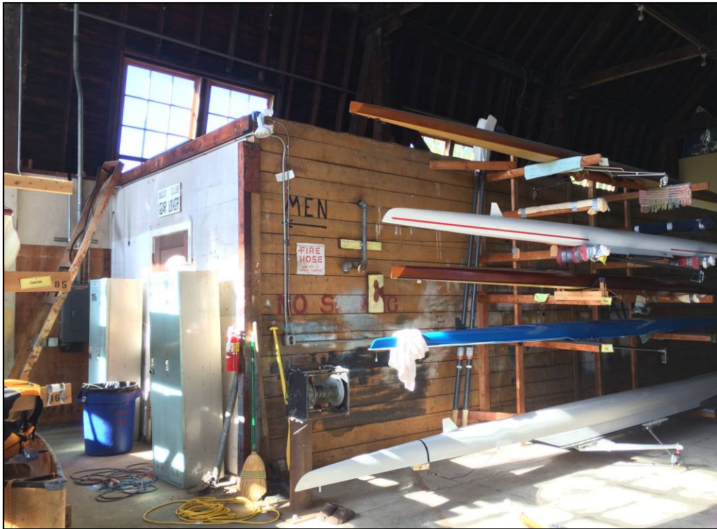
Figure 25. Interior view looking northwest, showing the partitioned area.
