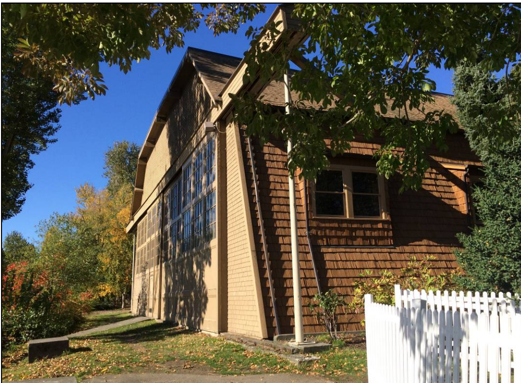
Figure 18. Looking west along the south façade and showing the southeast corner.
