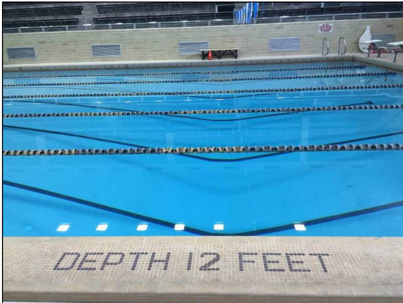
Figure 30. Above, a detail view of the pool tile work.
