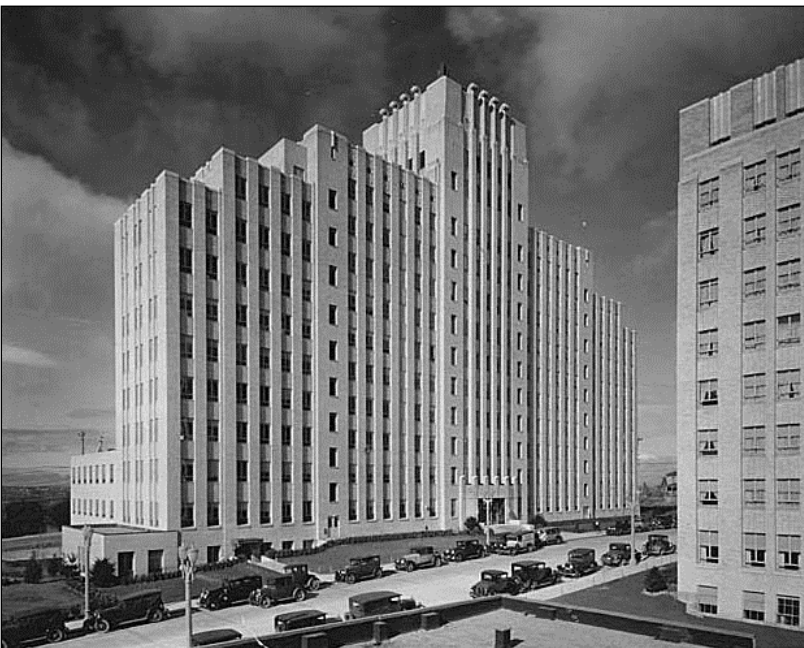
Figure 66. Below, Harborview Hospital on First Hill in 1931 (MOHAI, 1984)
