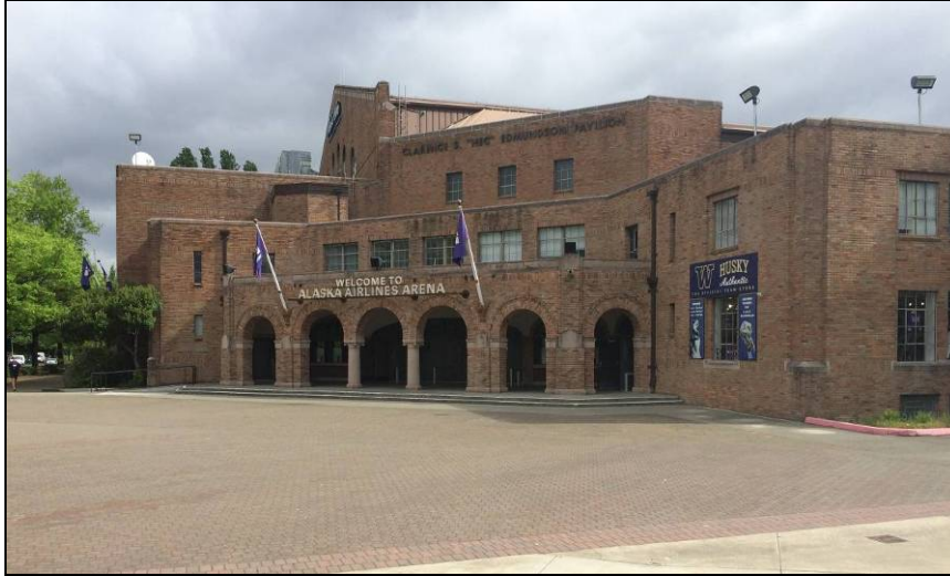
Figure 9. Above, looking northeast at the primary entry (ca 1928) and a portion of the west and south facades of the adjacent Hec Ed Pavilion.
