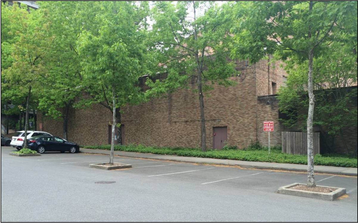
Figure 17. Above, looking southwest at the east facade. To the right, a portion of the abutting Grave Annex addition is visible.
