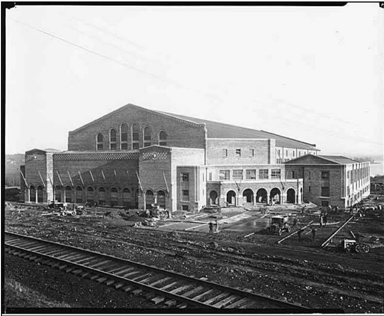
Figure 46. Above, a view of the Men's Athletic Building/Hec Edmundson Pavilion under construction in 1928 (MOHAI, Image No. 1983.10.1959.1). The view appears to include the rail line that became the Burke-Gilman Trail in the foreground.
