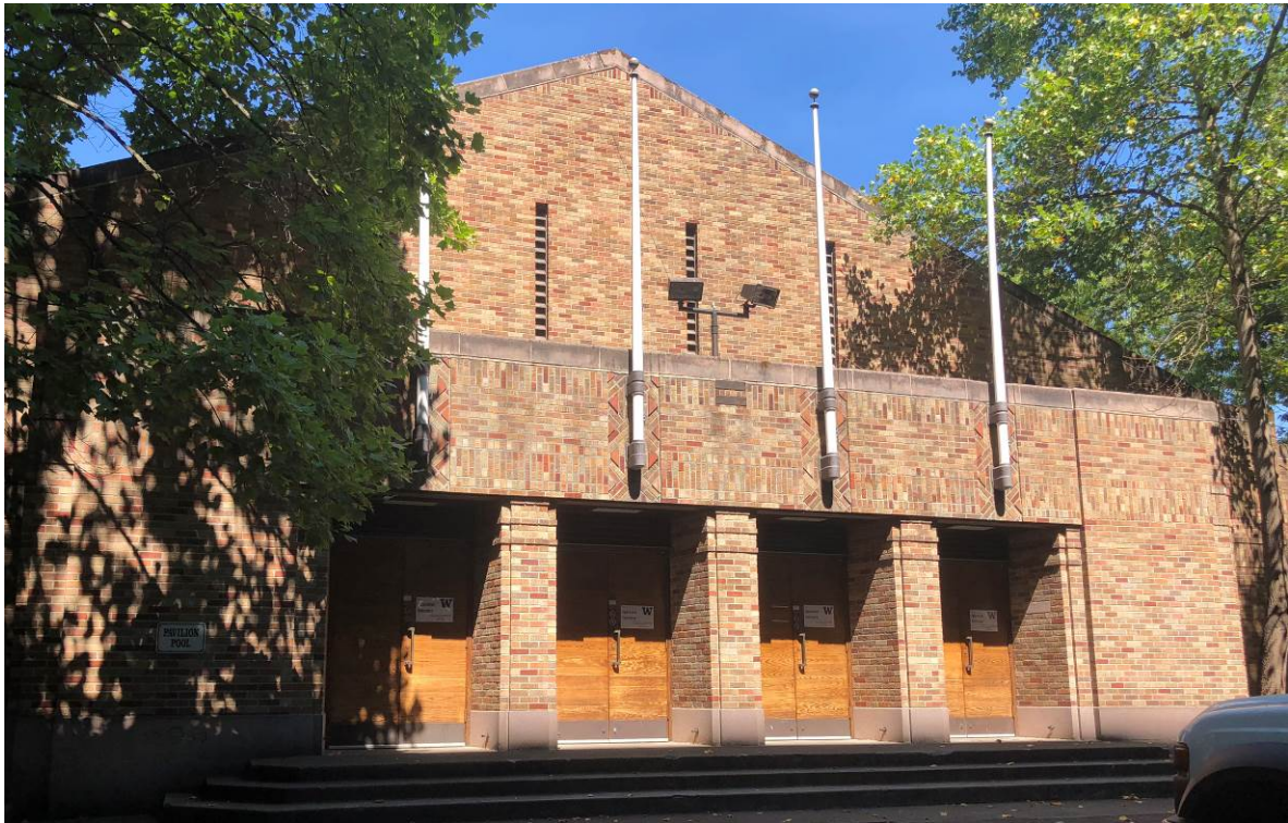
Figures 14 & 15. Above, looking southeast at the south façade entry and masonry patterns (August 8, 2018).
