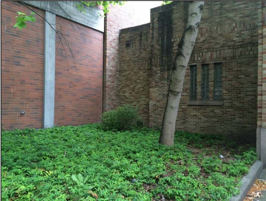
Figure 13. Detail view, looking northwest at portions of the Pavilion Pool south facade, the original Hec Ed Pavilion east facade and the ca. 1970 south storage addition east facade.
