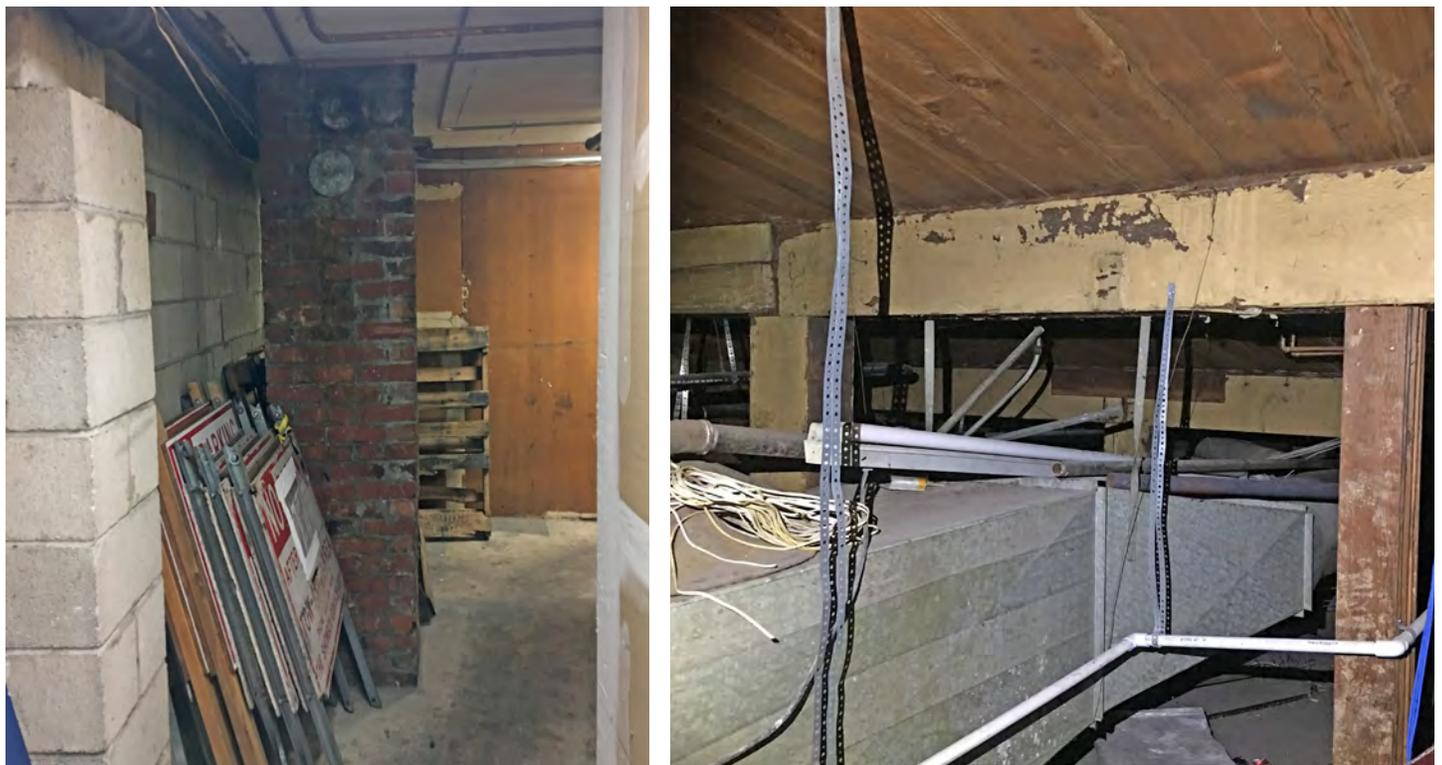
**Figure 57.** Service area, looking east along the rebuilt north facade. The brick chimney is original to the 1916 construction of the building (above left). A view looking west (above right) below the Showbox passageway showing the framing and ramp that are original to the 1939 remodel.
