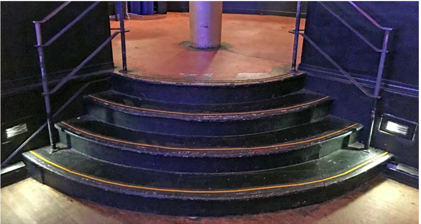
**Figure 40.** Showbox, detail of curved stairs and metal railings up from the dance floor to the terraced seating that are original to the 1939 remodel.
