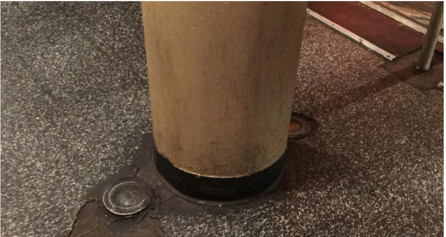
**Figure 38.** Showbox, detail of the floor lights original to the 1939 remodel that provided a light wash up the column.
