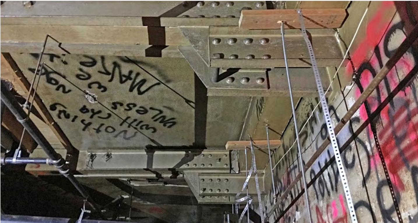
Figure 51. Showbox, fly loft showing the building framing and the graffiti within the space.
