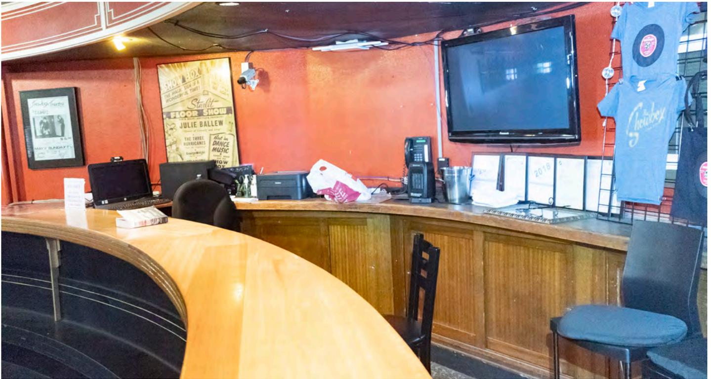
**Figure 27.** Showbox, looking north at the ticket window. The counter and back cabinets and overall opening are original to the 1939 remodel and 1940 modifications creating the Showbox. This space originally functioned as a bar for guests on their way to the performance volume.
