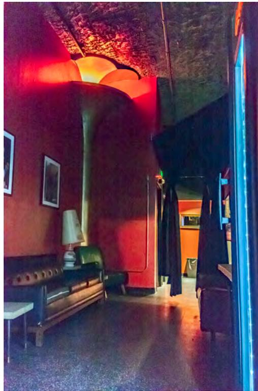
**Figure 46.** Showbox, outer green room looking south. Note how later partitions were abutted up to the column elements leaving them intact.
