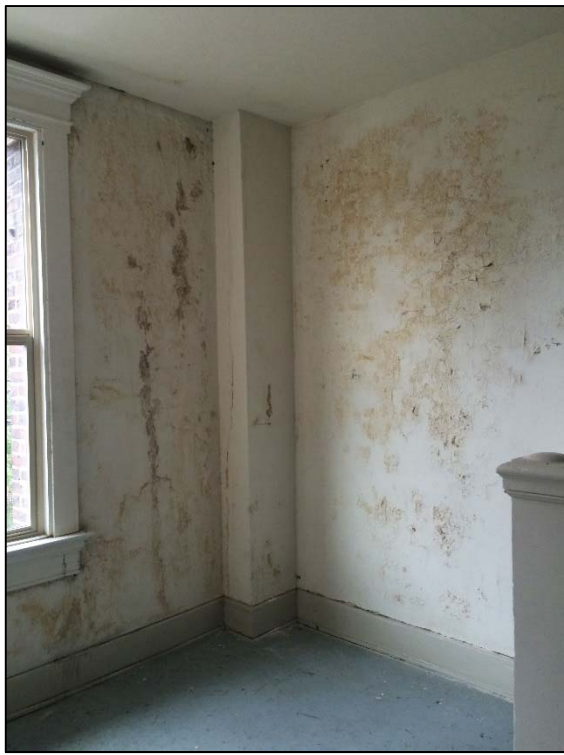
Figure 77. Above, the contemporary elevator lobby. Figures 78 & 79. Below left and right, west stair hall and adjacent water-damaged plaster at southwest corner. Note also partition, left, fitted against original window frame.
