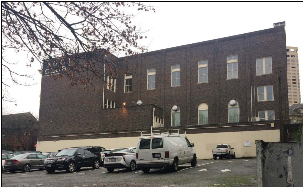
Figure 48. Below, looking southeast at the north facade and the setbacks along the north.
