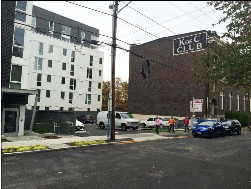
Figure 44. Above, looking east on Harvard at the west facade and a portion of the south facade.
