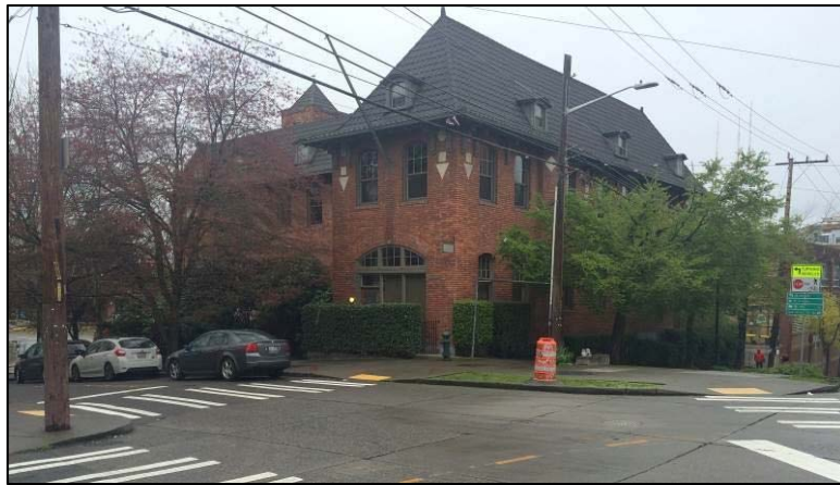
Figure 36. Above, looking northeast from the building at Fire Station 25.
