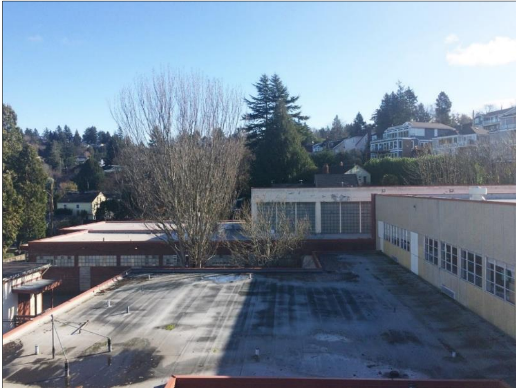
Figure 33. Above, looking east over the one-story section in the center of the school and a portion of the second story north façade, right. This portion of the school was built in 1966-1968. In the background there is the gym and fieldhouse sections, built in 1953-1954.
