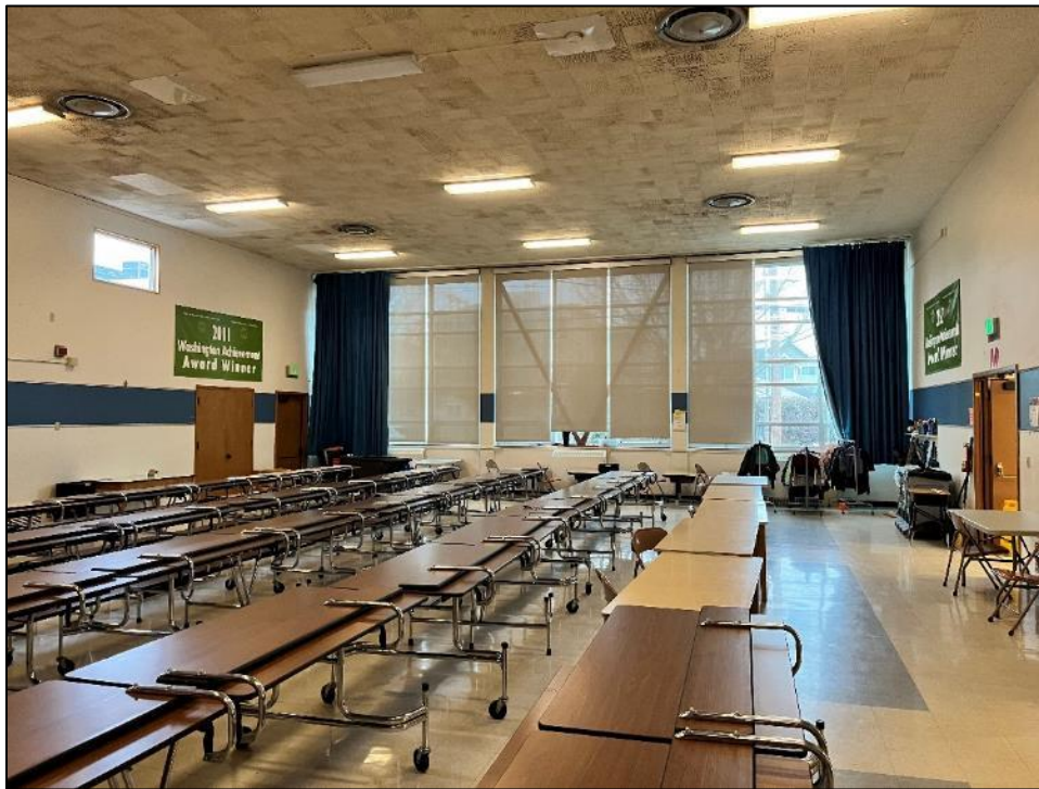
Figure 49. Above looking southwest at the west perimeter wall of the lunchroom. The X-bracing inside the west wall is an additive element from a seismic upgrade project.
