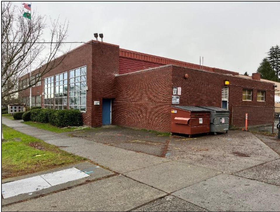
Figure 19. Above, looking northeast at the kitchen extension, driveway, and portion of the parking/service area on the back (south side) of the school site.
