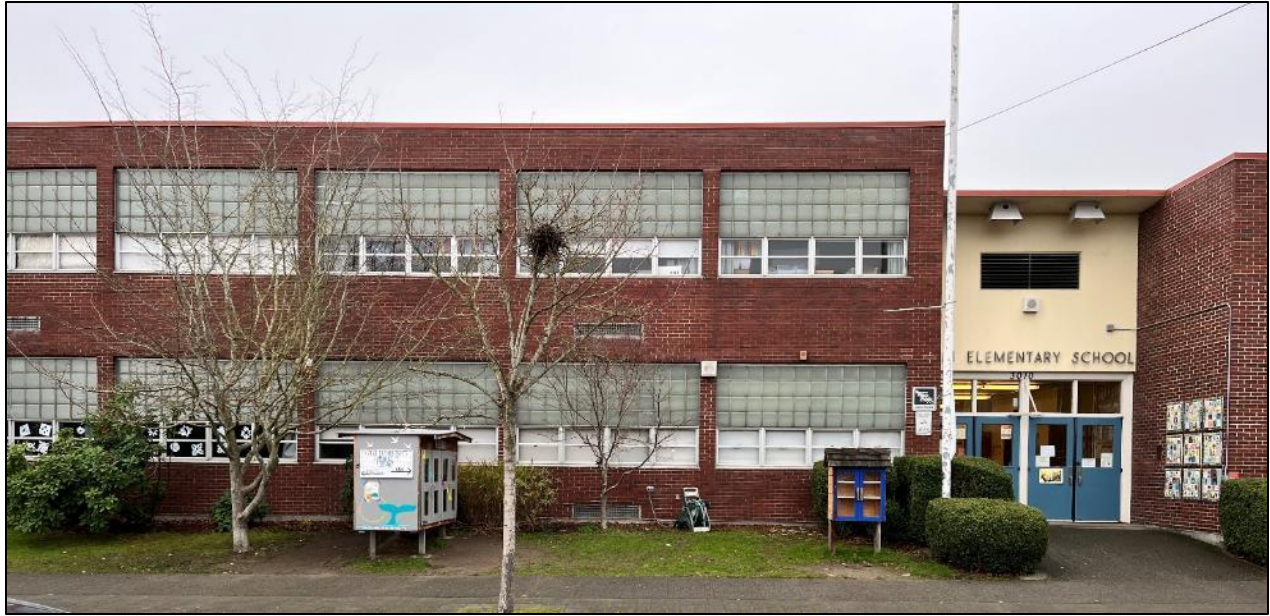
Figures 21, 22 & 23. Looking east at a portion of the west façade with the recessed main entry off 59 th Avenue SW, and detail views of the entry doors and decorative wall tiles.
