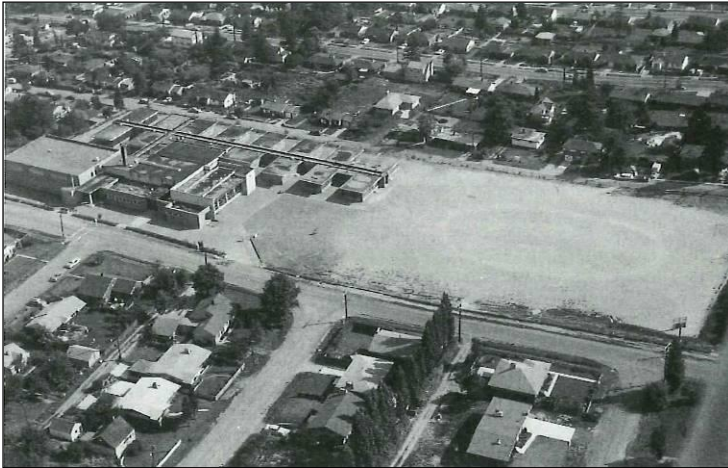
Figures 95A & 95B. Arbor Heights Elementary, 3701 SW 104 th Street (1949, George W. Stoddard), Demolished & Replaced
