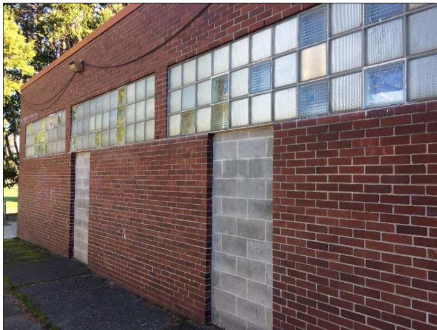
Figure 38. Below, looking east along the west façade of the Fieldhouse section, showing infilled openings in the brick veneer wall.
