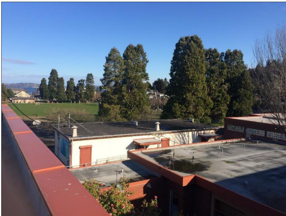
Figure 29. Left, view looking northeast from the roof of Unit A at lower roofs roof and open courtyard.
