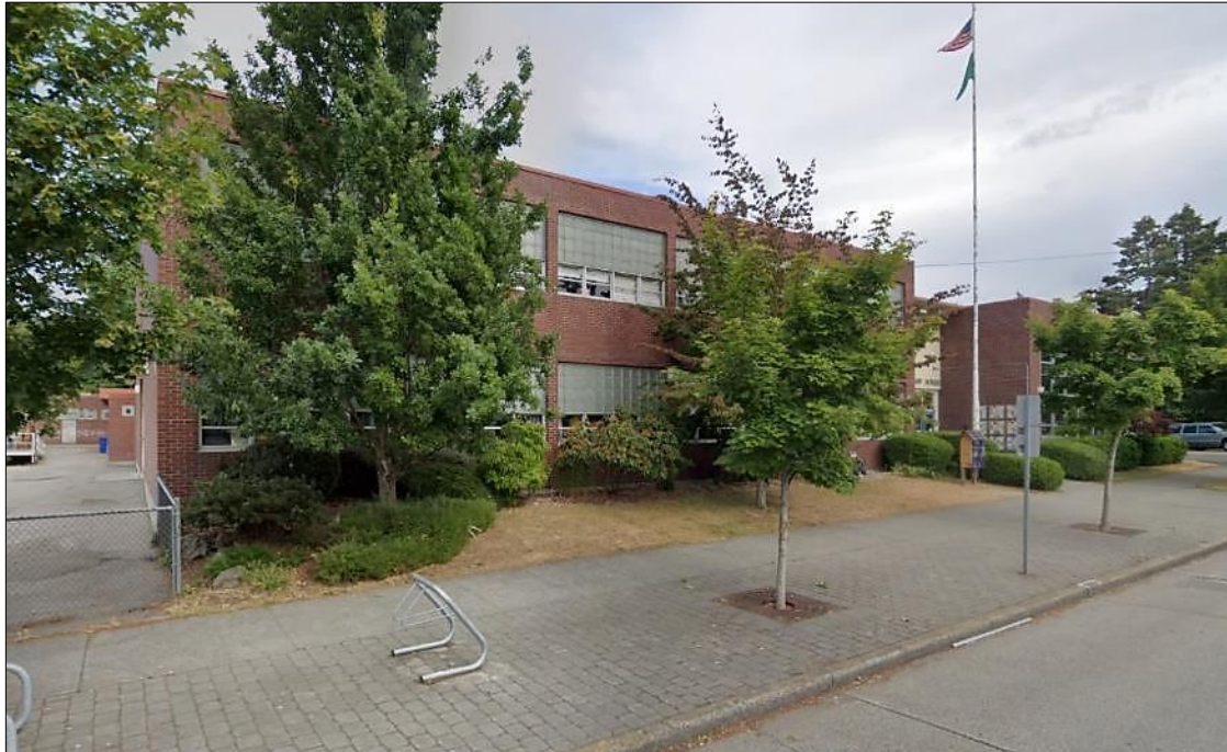
Figures 24 & 25. Above and below, looking southeast at the west façade along 59 th Avenue SW, above in summer showing the landscape in the front yard setback (GoogleEarth), and below, during winter months. These show the large openings filled with glass block and operable aluminum sash, which are typical on the east and west facades of Unit A that illuminate classrooms and offices.
