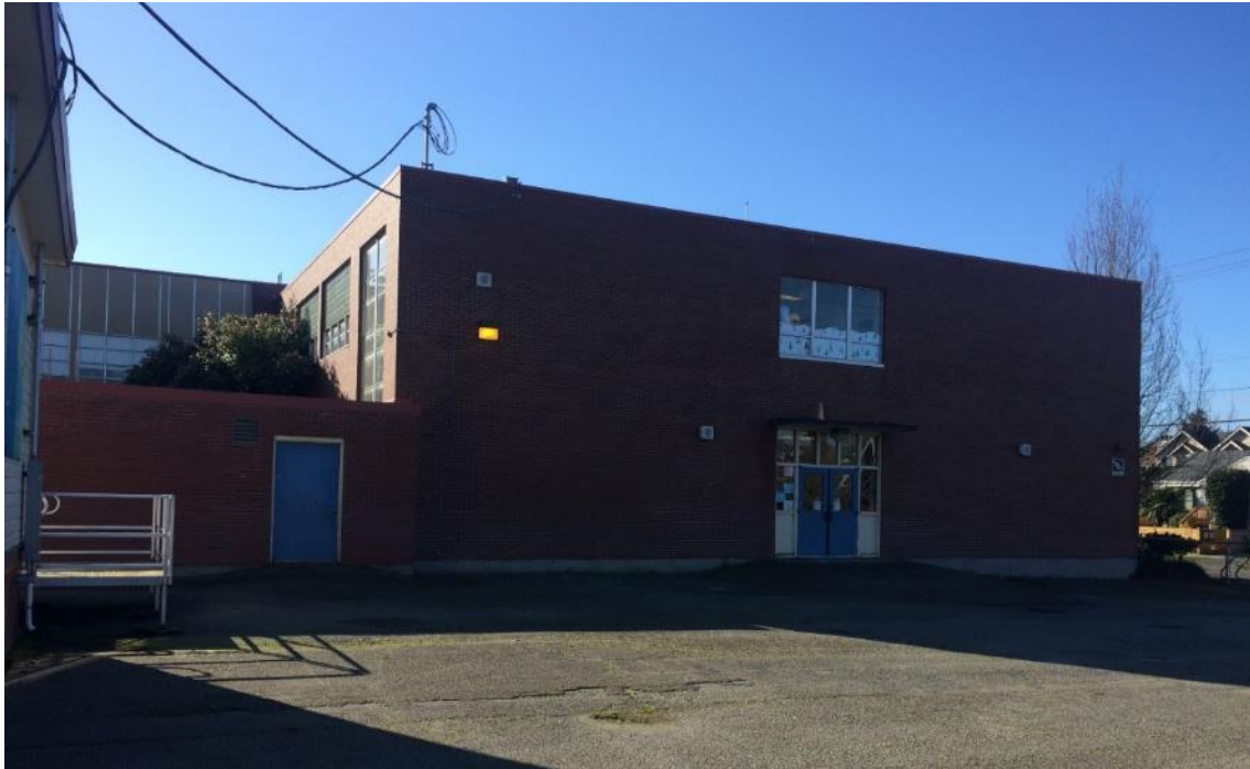
Figure 28. Above, looking south and the north end façade of Unit A, the two-story classroom wing. The enclosed courtyard space is to the east of it
