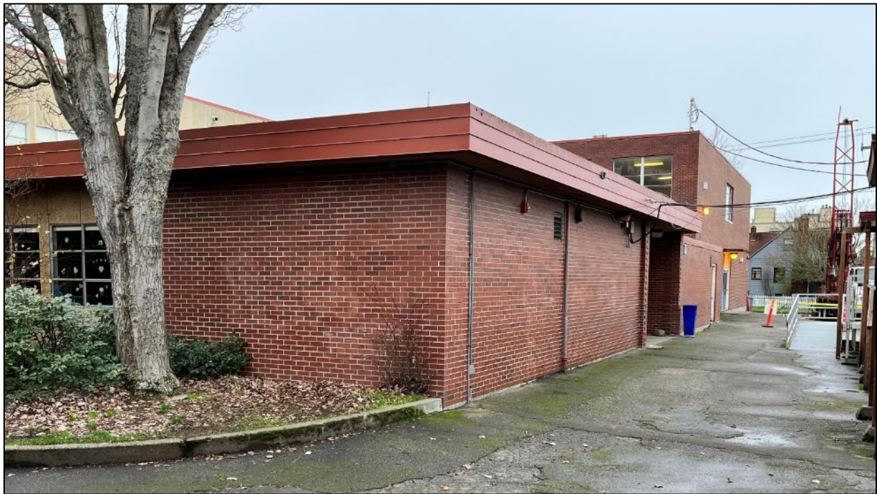
Figure 30. Above, looking west along the north façade of Unit B, the center section of the school, built in 1966-1968. Unit A, in the background, is from 1953-1954.
