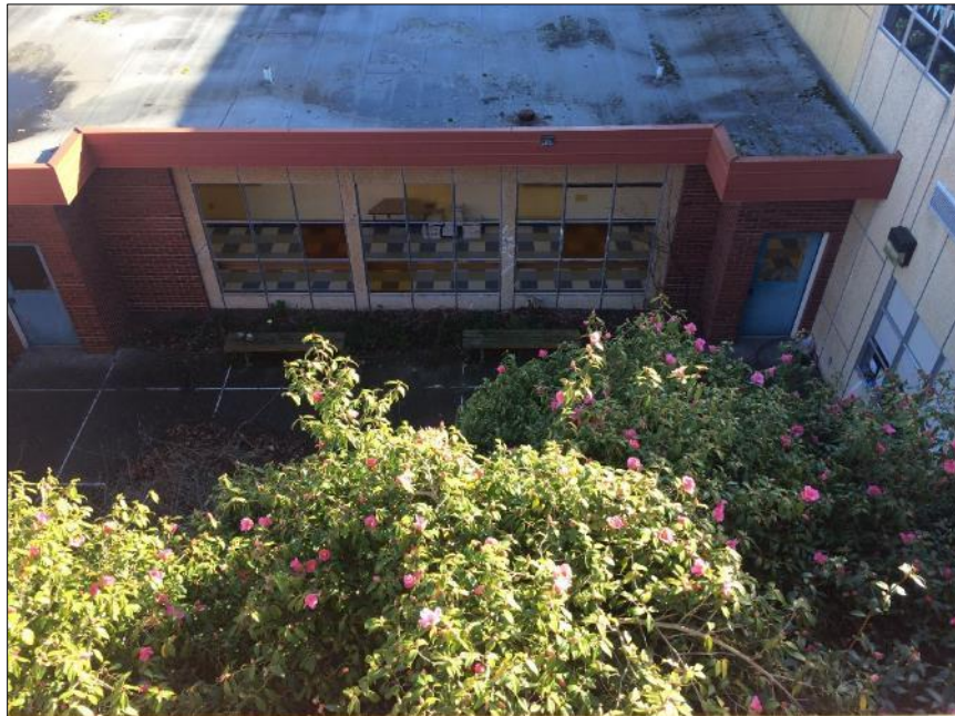
Figure 34. Below, looking east and down from the roof into the outdoor classroom inside the north perimeter wall.
