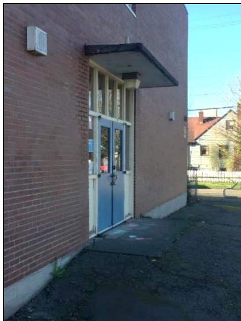
Figures 31 & 32. Below, detail views of doors in the north façades.
