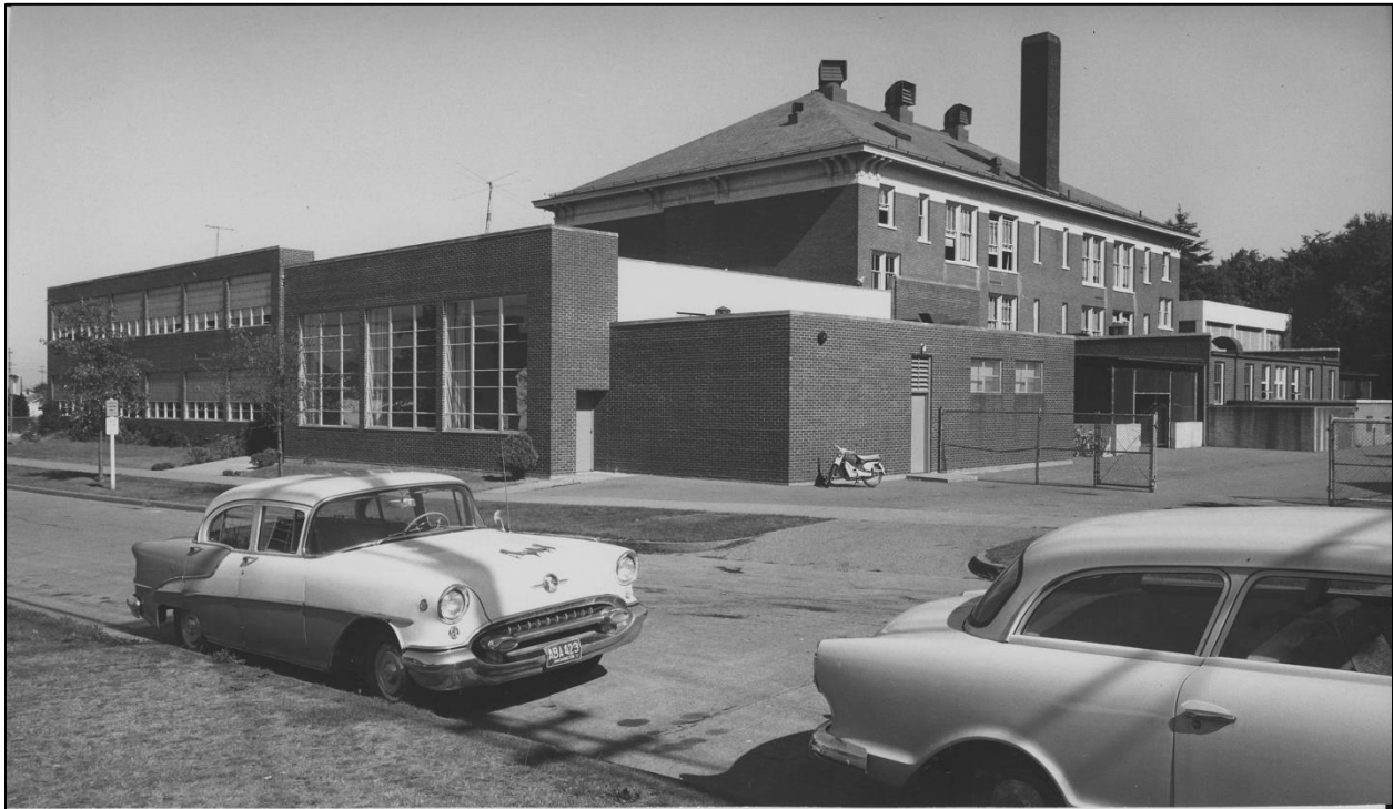
Figure 75. Below, looking northeast across 59 th Avenue SW at the primary west façade and secondary south façade of the 1953-1953 addition with the 1913 school building behind it (SPS).
