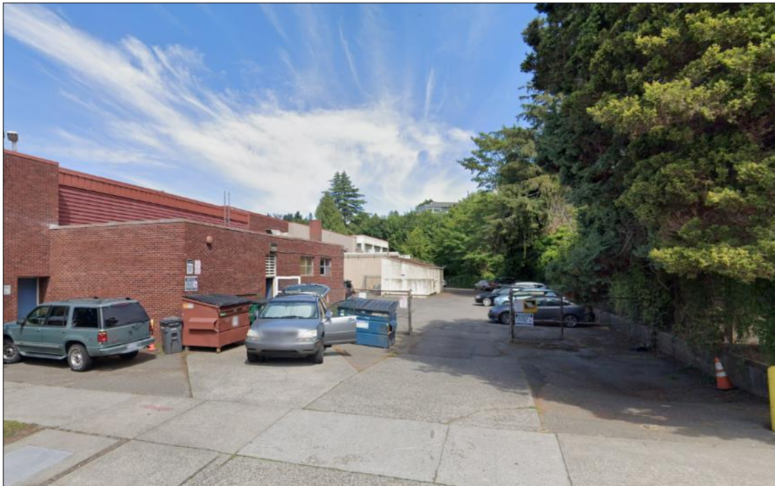
Figures 44. Above, looking east into the parking lot and service area on the south side of the site. The light colored building masses are portions of the single-story boiler/mechanical room and the taller gymnasium. Note the steep grade change to the south and southeast (right).
