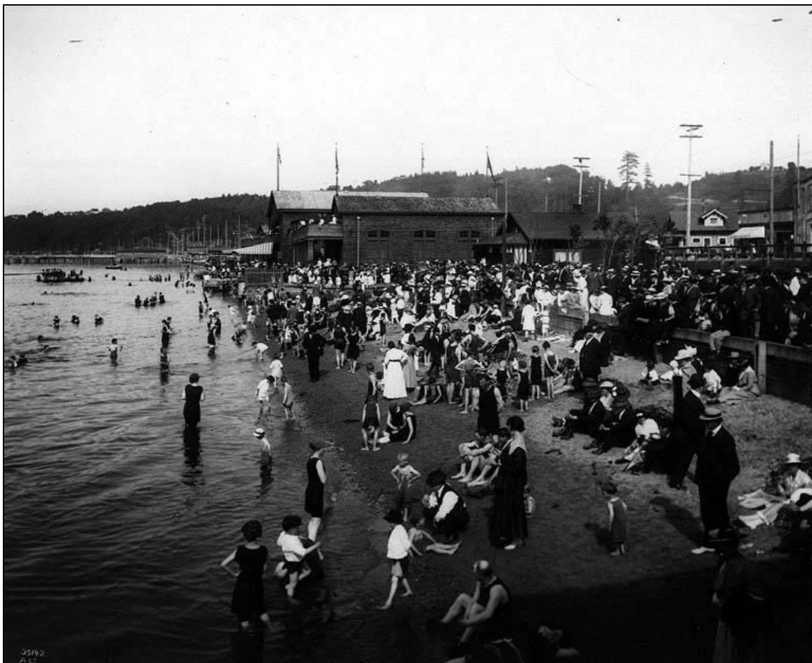
Figure 65. Above, the Alki Bathing Beach in 1930 (Asahel Curtis, photographer, UWLSC UR1330).
