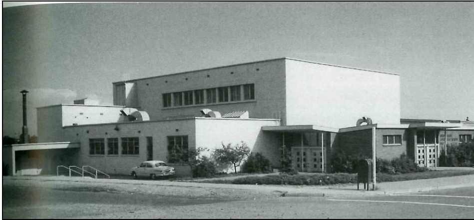
Figures 97A & 97B. D. T. Denny Middle School, 8402 SW 30 th Avenue (1952, Mallis and DeHart), Demolished & Replaced
