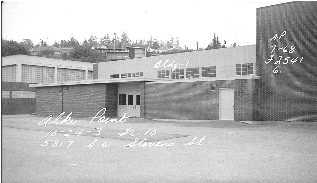
Figure 84. Above, looking southeast at the central part of building's new addition (Unit C) and partial north and east facades in the July 1968. Portions of the 1953-1954 gym are in the background.
