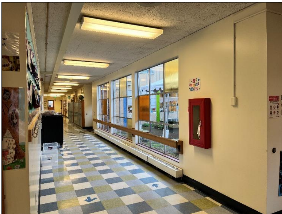
Figure 57. Below, looking southwest along the glazed corridor wall into the outdoor classroom / courtyard.
