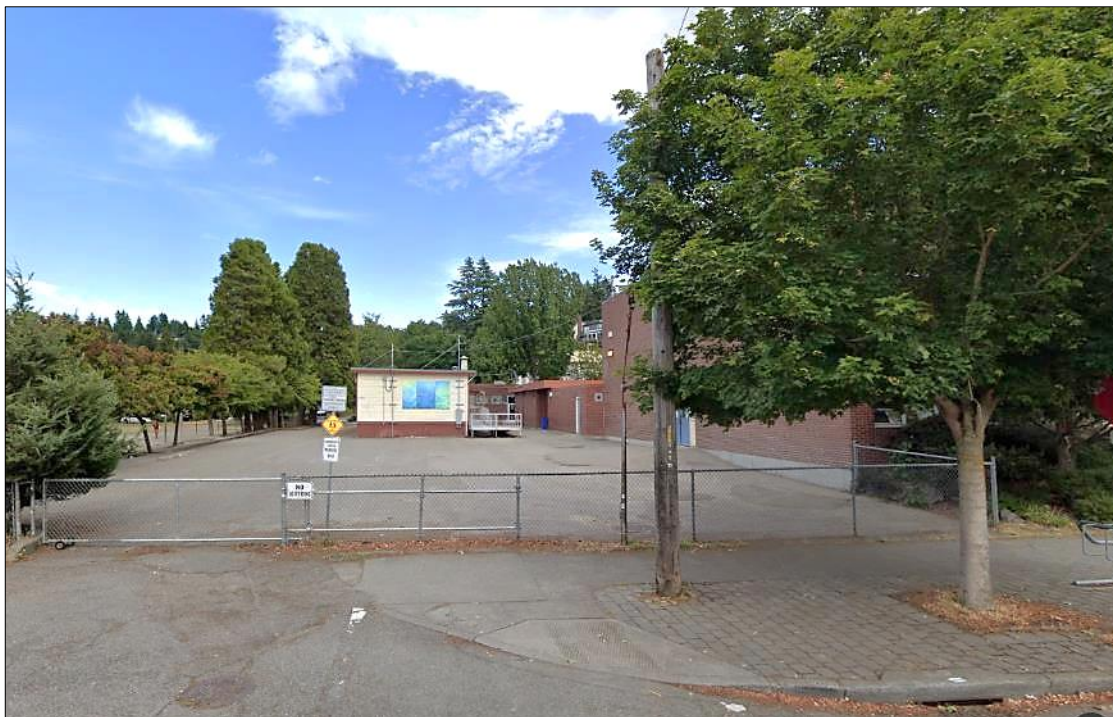
Figure 27. Below, looking east from 59 th Avenue SW at the hardscape play area directly north of the school, and the temporary portable classroom building.
