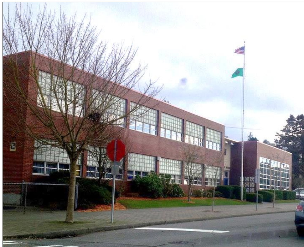
Figures 24 & 25. Above and below, looking southeast at the west façade along 59 th Avenue SW, above in summer showing the landscape in the front yard setback (GoogleEarth), and below, during winter months. These show the large openings filled with glass block and operable aluminum sash, which are typical on the east and west facades of Unit A that illuminate classrooms and offices.
