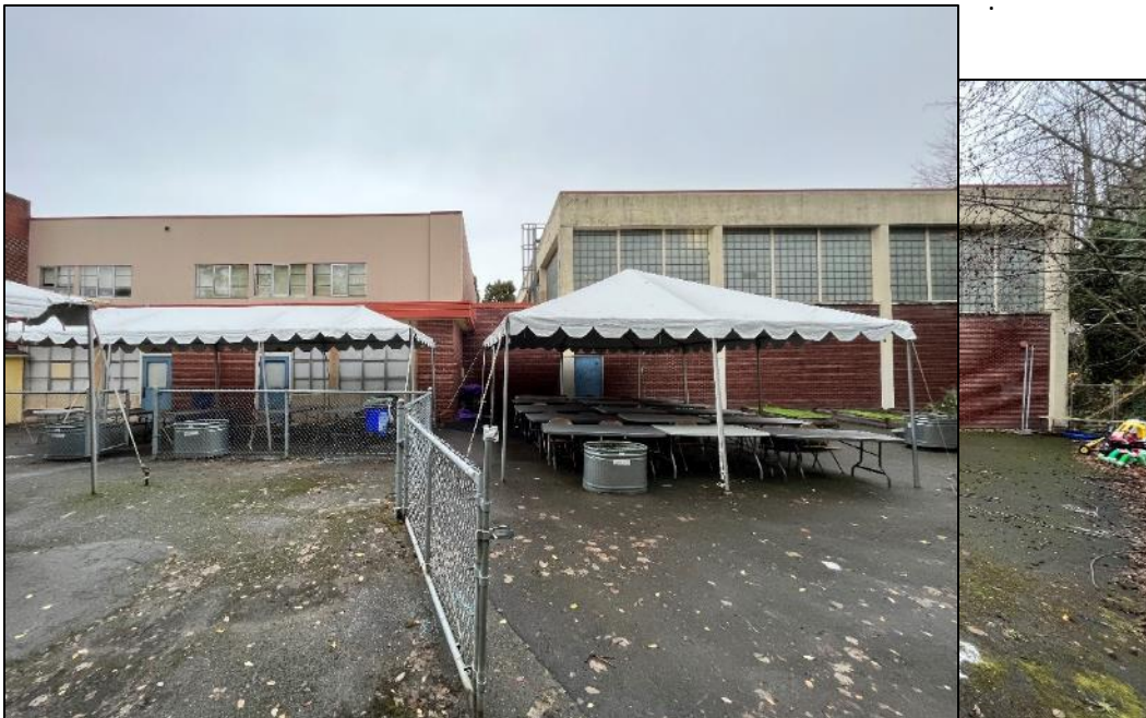
Figure 45. Below, a composite photo view looking south across a paved lot at the gym (right) and portion of the two-story classroom section in the center of the assembly (left)
