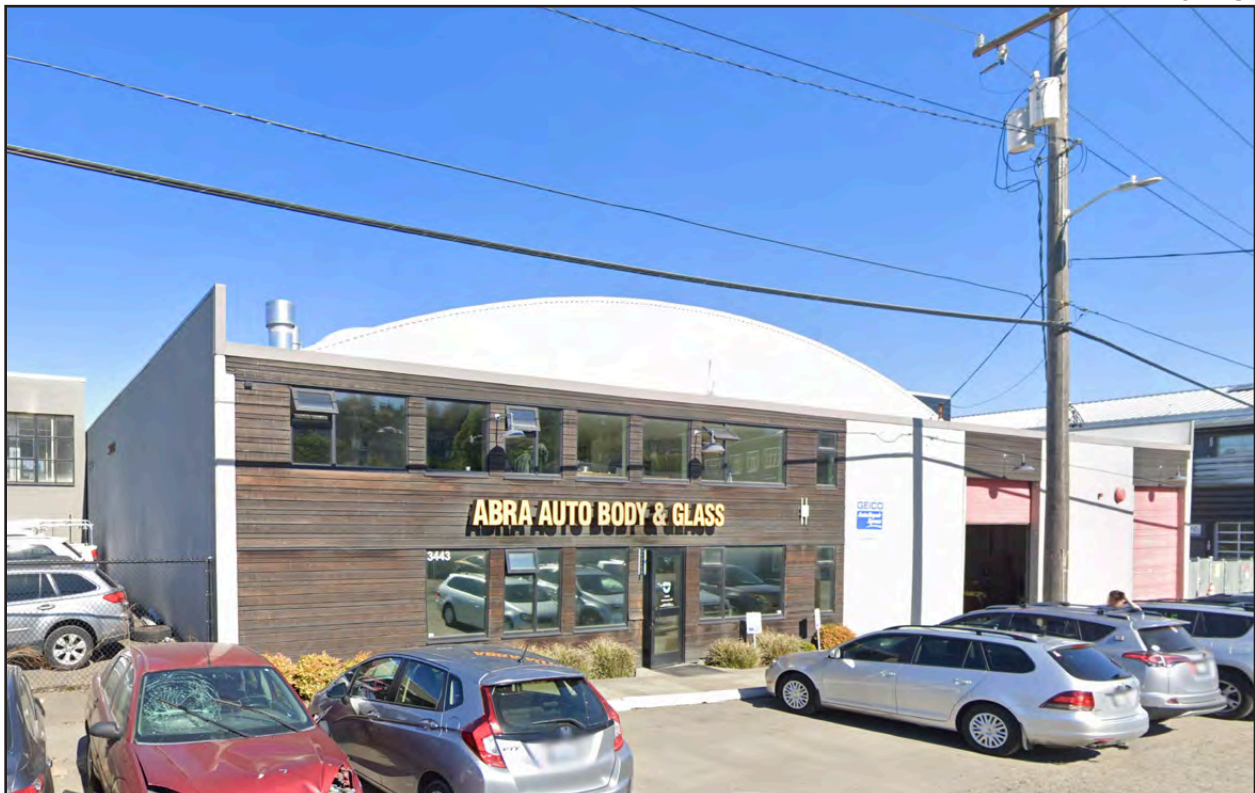
Figure 105 • Shifton Plywood Co. 2021 (1958, extant)
