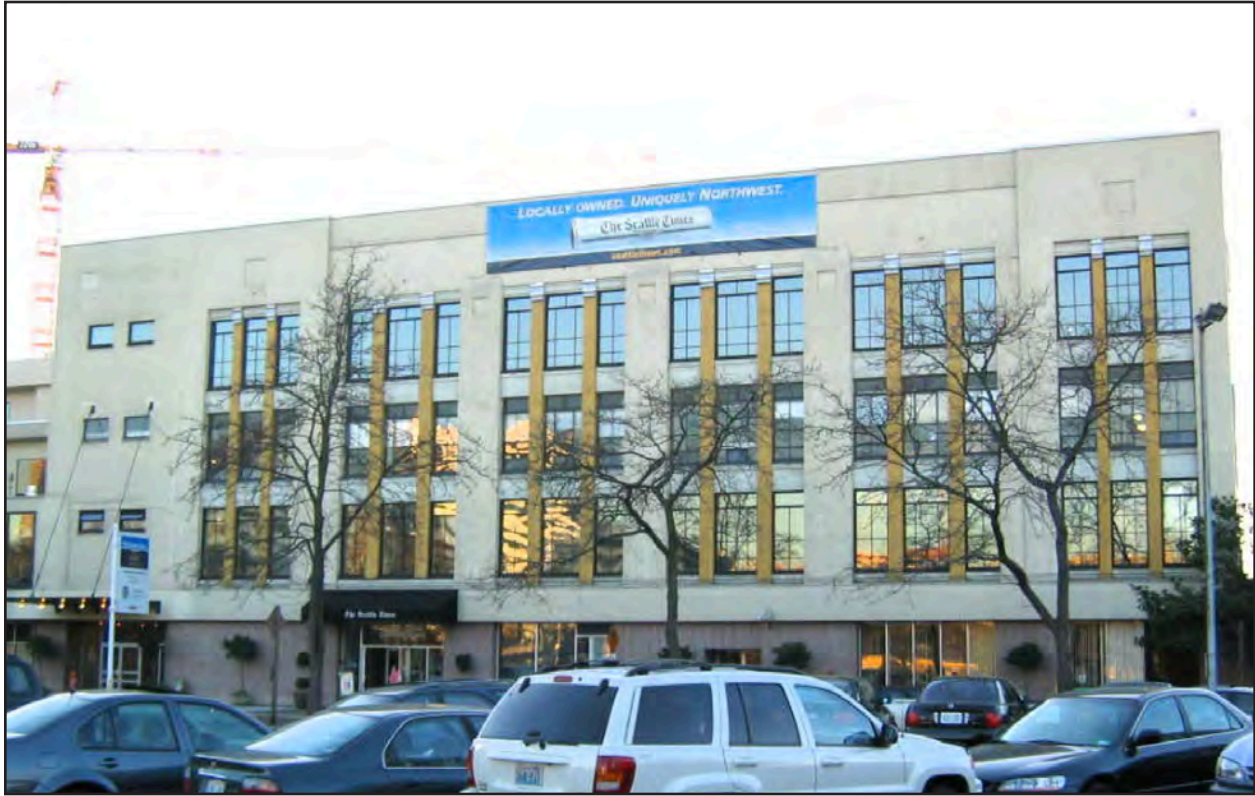
Figure 85 • Peck and Hills Furniture Company & Baxley Dress Manufacturing Company, 1000 Denny Way (1929, Albert C. Martin, extant)
