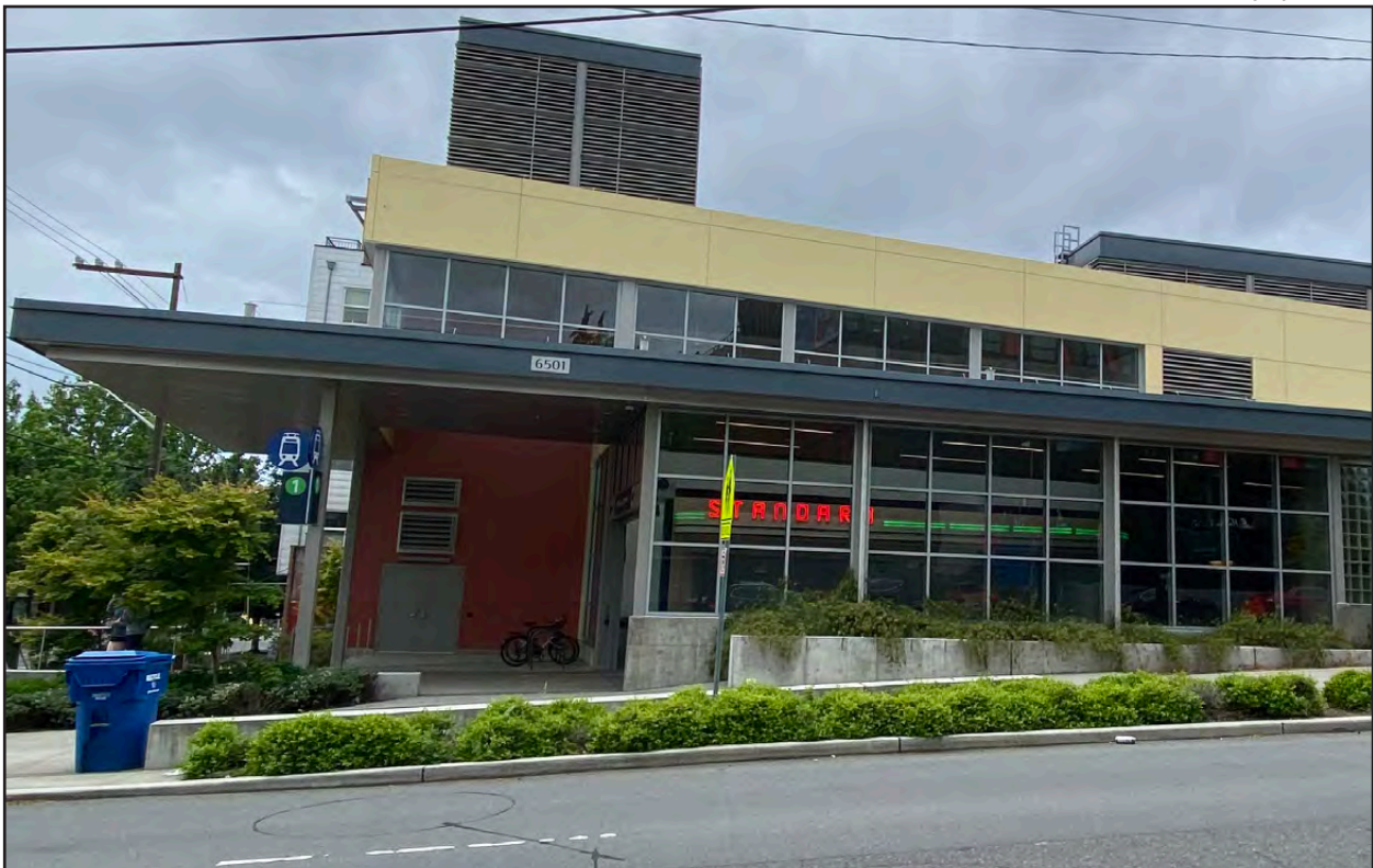
Figure 82 • Standard Radio façade reinstalled at Roosevelt light rail station
