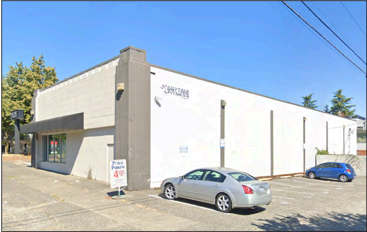
Figure 45 • 2222 California Ave SW, North Admiral neighborhood (1942, extant)
