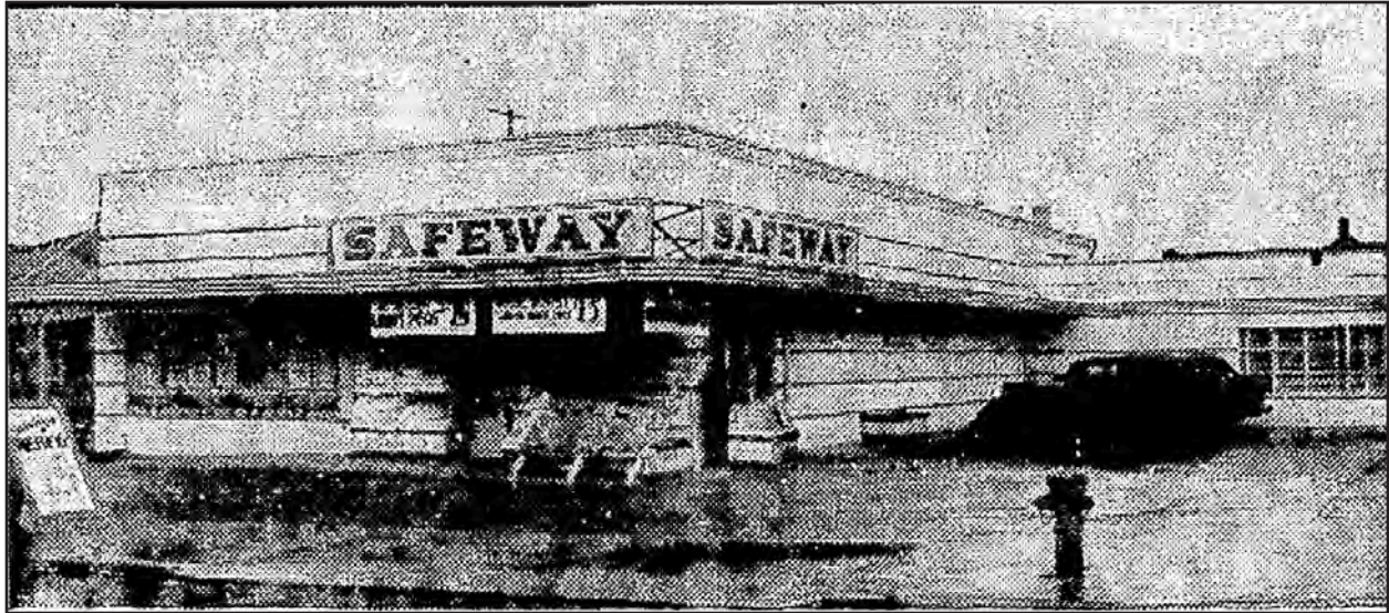
Figure 39 • Seattle Safeway at 6th Ave W and W McGraw St, Seattle (demolished), 1939
