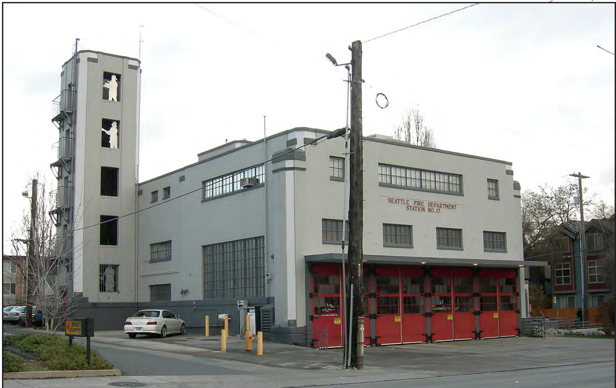
Figure 70 • Fire station #17, 101 NE 50th St (1930, architect unknown, City of Seattle Landmark)
