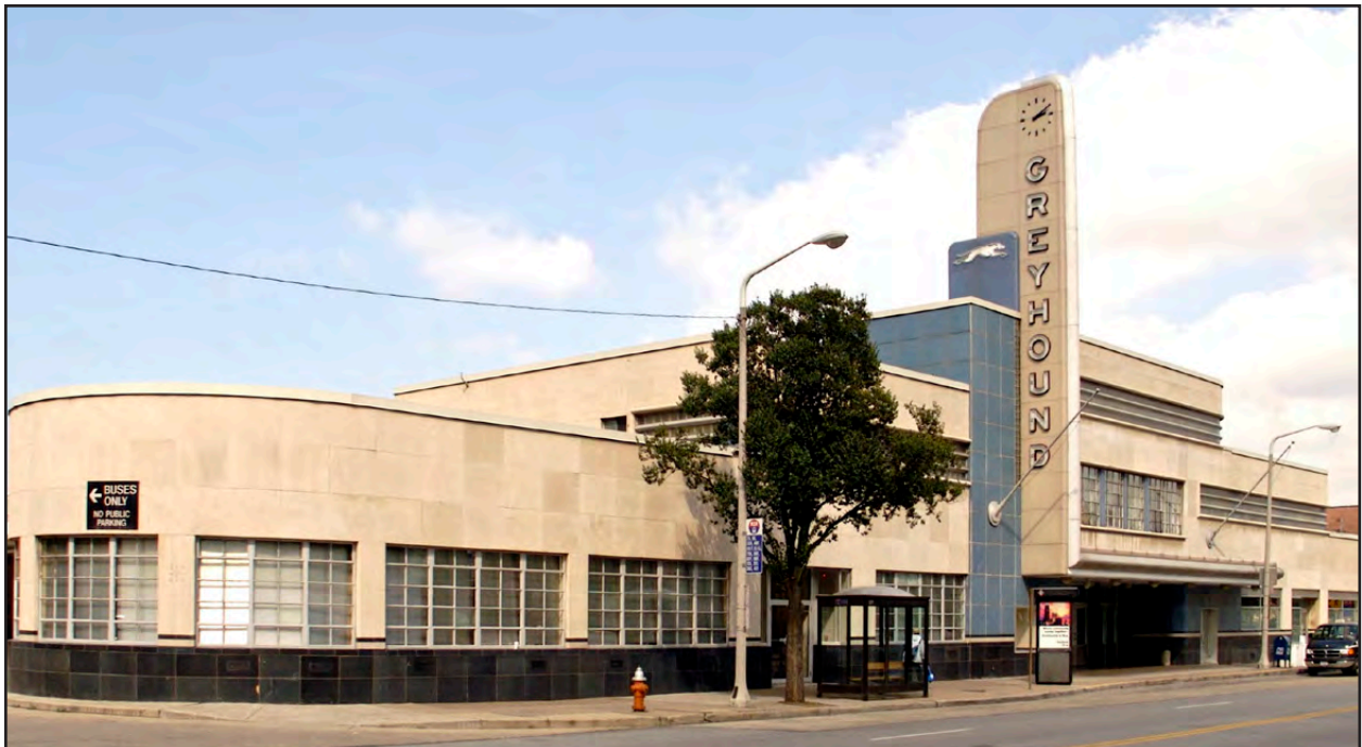
Figure 58 • Greyhound Bus Terminal, Cleveland, OH (1948, William Strudwick Arrasmith, National Register)
