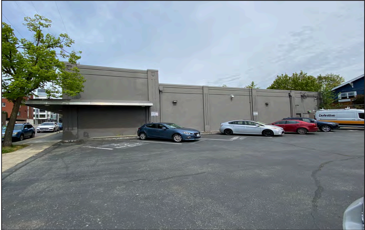
Figure 12 • 6206 Roosevelt Way NE, southern facade
