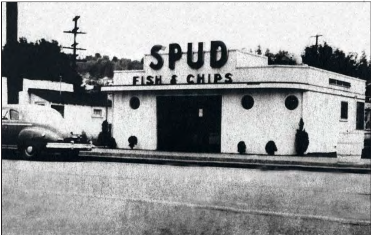
Figure 68 • SPUD Fish 'n' Chips (Alki Location, now demolished)
