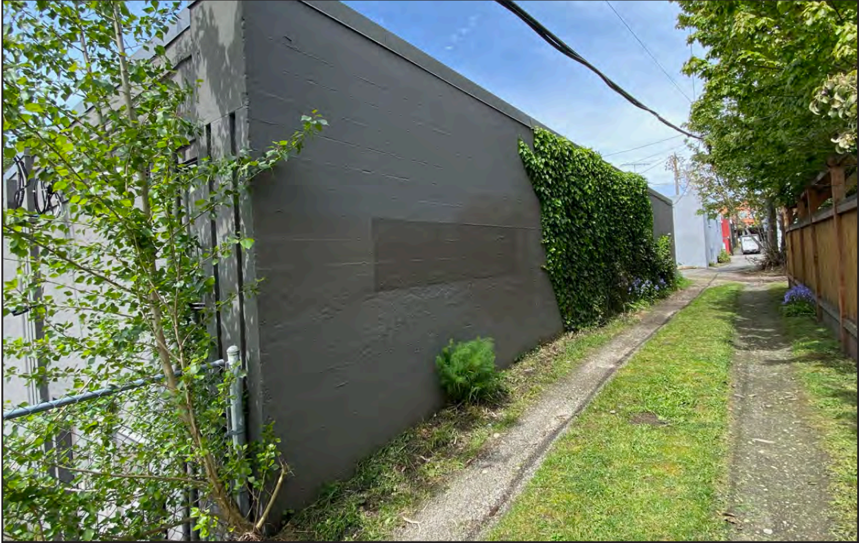
Figure 14 • 6206 Roosevelt Way NE, eastern facade
