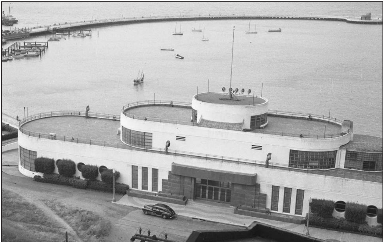
Figure 64 • San Francisco Bathers' Building (1936, William A. Mooser II, National Register, now National Maritime Museum)
