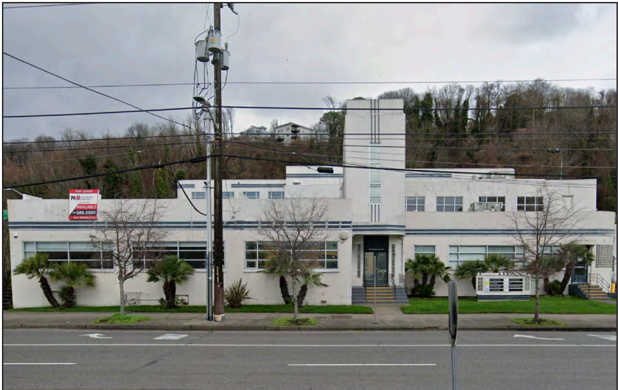
Figure 90 • Western Pacific Chemical Company building, 1430-1436 Elliot Ave (1940, extant)
