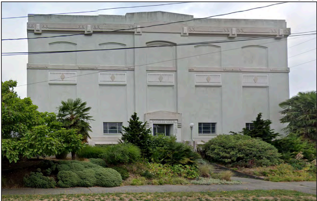
Figure 80 • North Rectifier Substation, 814 NE 75th Street NE (1954)
