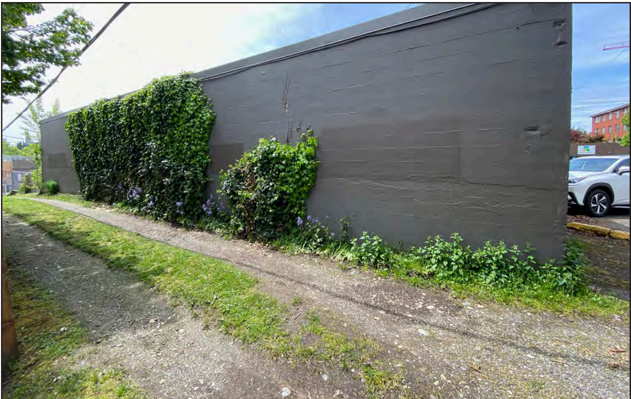
Figure 15 • 6206 Roosevelt Way NE, eastern facade
