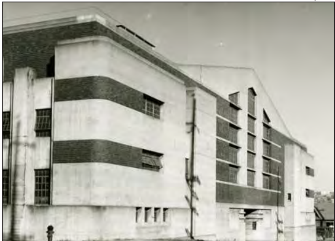
Figure 74 • Seattle Center House, 305 Harrison Street (1939, Naramore & Young, City of Seattle Landmark)
