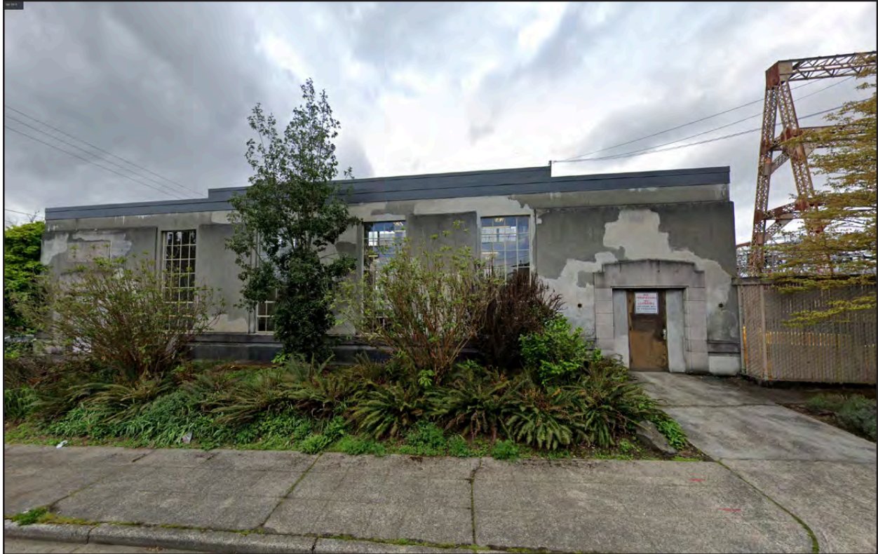
Figure 79 • North Distribution Substation/North Substation Machine Shop, 814 NE 75th Street NE (1930)
