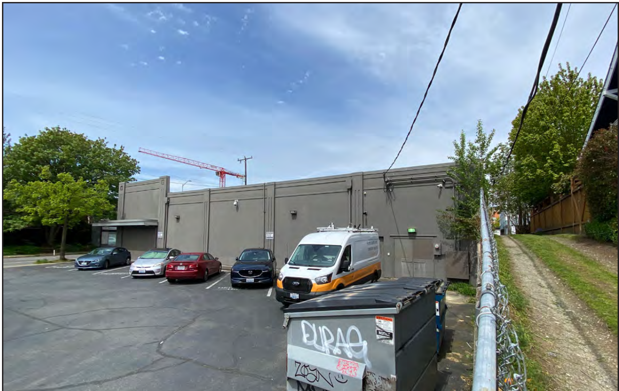
Figure 13 • 6206 Roosevelt Way NE, southern facade
