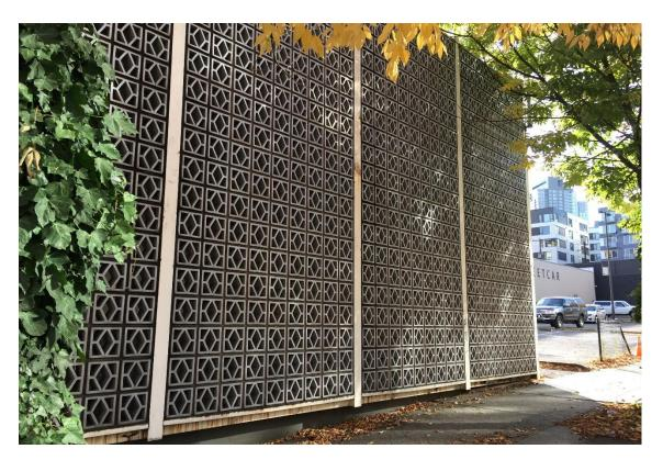
FIGURE 9: WEST ELEVATION, DETAIL SHOWING TERRACOTTA TILE SOLAR SCREEN (2017)
