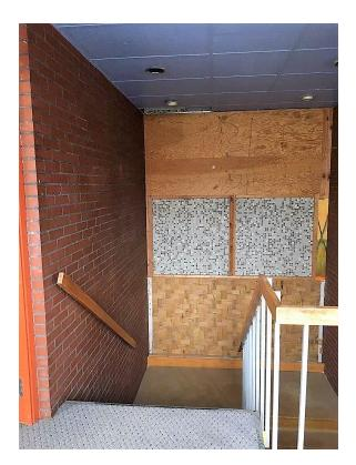
FIGURE 35: INTERIOR, FIRST FLOOR - ORIGINAL MOSAIC TILE PARTIALLY COVERED (2018)
