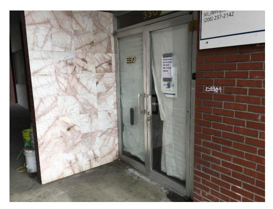
FIGURE 25: WEST ELEVATION, DETAIL SHOWING ORIGINAL ENTRY DOORS (TILE HALF WALL LIKELY NOT ORIGINAL) (2018)
