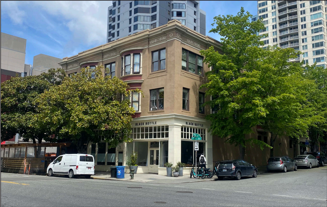
Figure 48 • 2600-2604 First Avenue, former Pacific Hospital Building (Henry Dozier, 1904)
