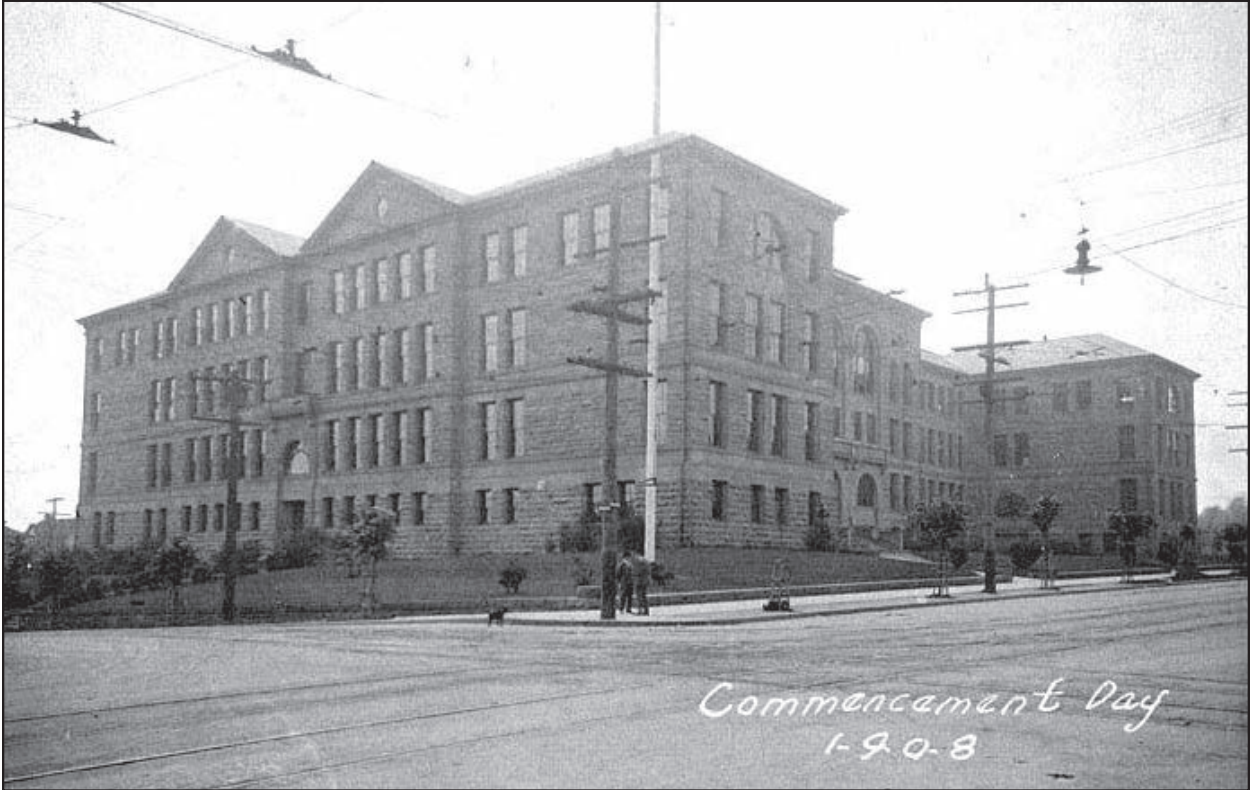
Figure 29 • Broadway High School (1902, Boone & Corner, demolished), 1908
