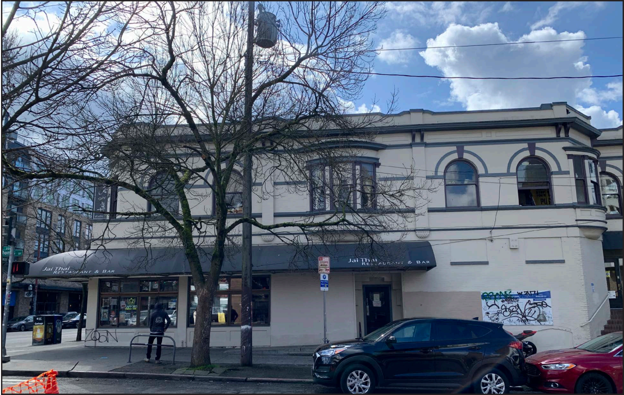
Figure 15 • 229 Broadway E, Northern façade
