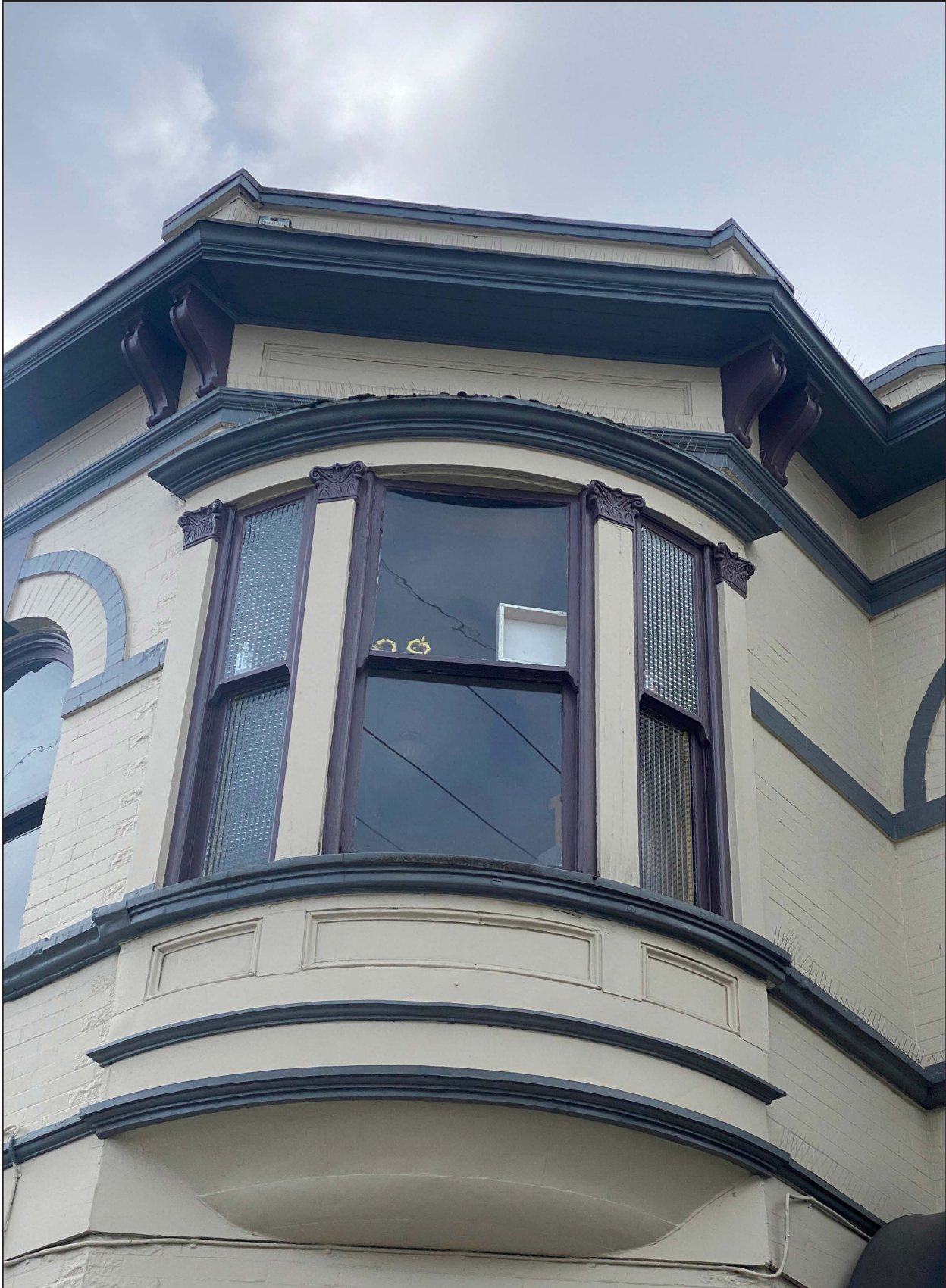
Figure 17 • 229 Broadway E, northern façade, western end detail
