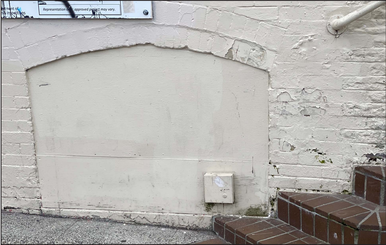
Figure 18 • 229 Broadway E, northern façade, detail of infilled opening
