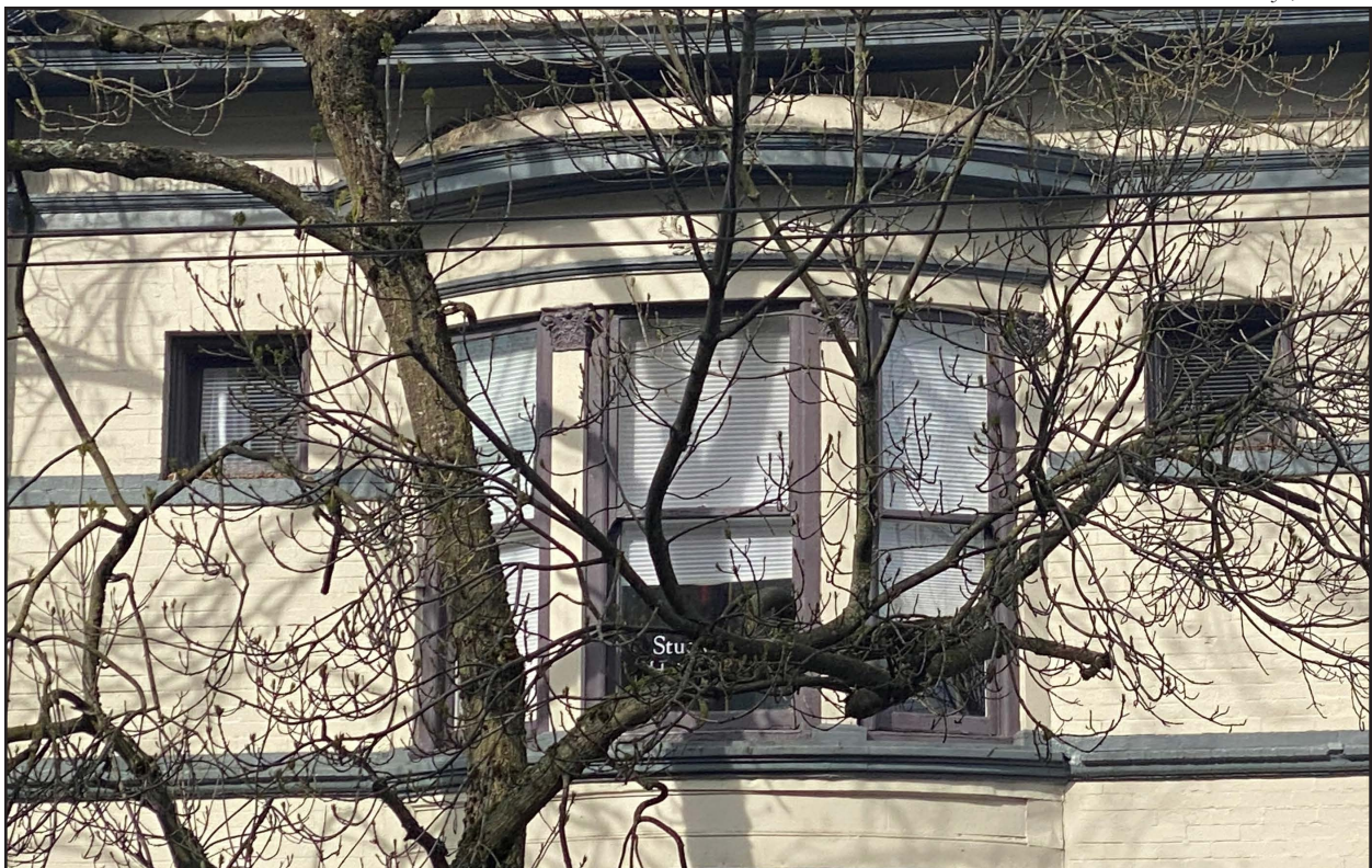
Figure 12 • 229 Broadway E, eastern façade, exterior details
