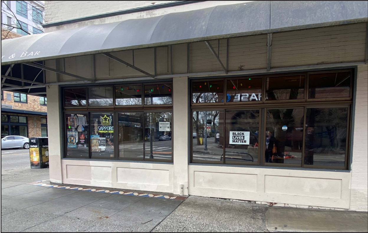
Figure 19 • 229 Broadway E, northern façade, detail of storefronts
