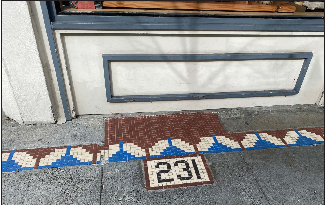
Figure 11 • 229 Broadway E, eastern façade, wooden storefront bulkhead
