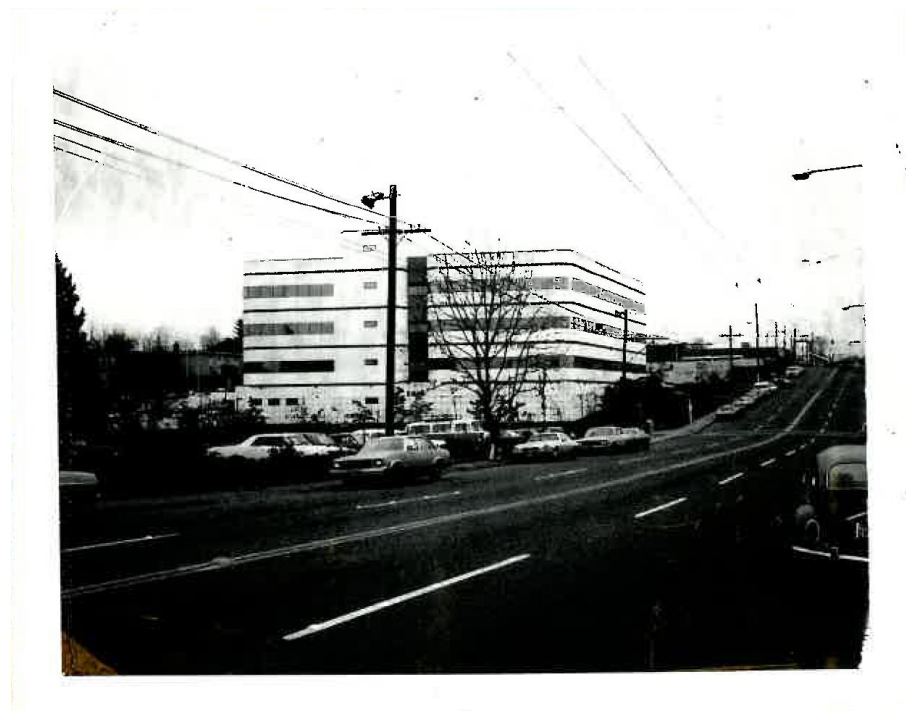
Figure 4: Original four-story building, west elevation viewed looking east on S Jackson St., 1974 Source: (King County Assessor, 1974)
