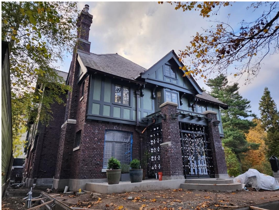
Figure 22: Southeast corner of the house, 2022. (Author's photo.)
