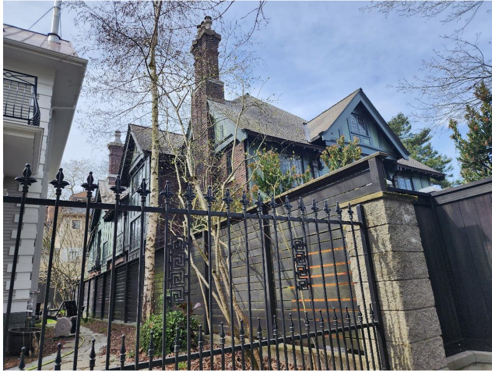
Figure 25: Southeast corner of the house, 2023. (Author's photo.)
