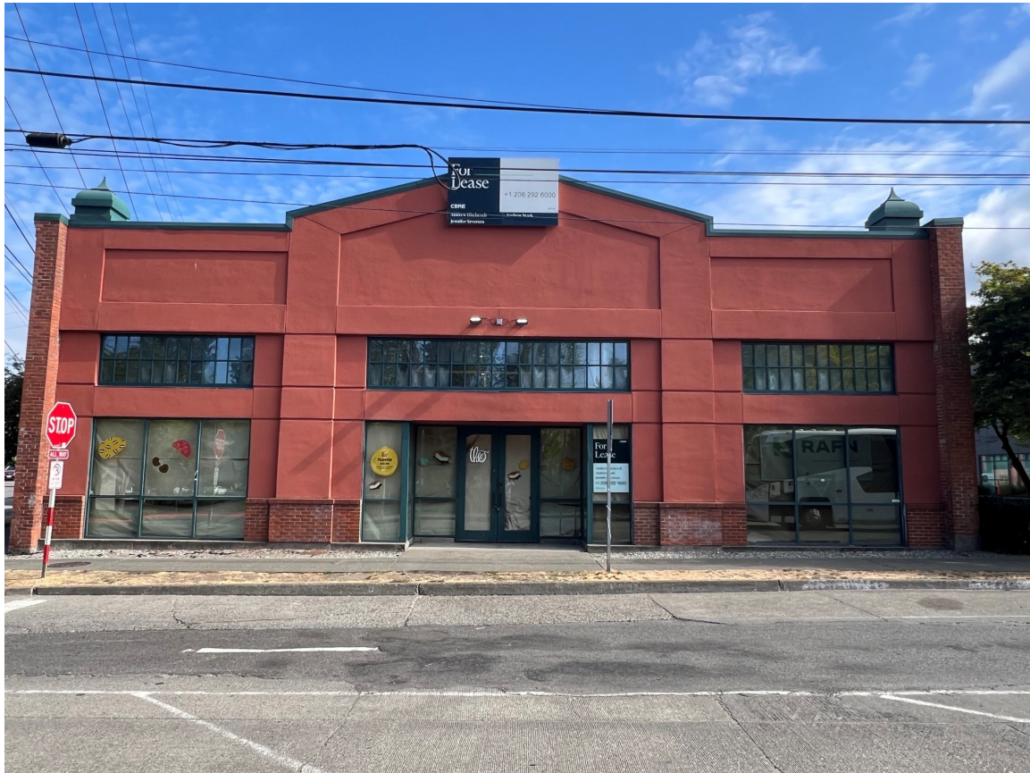
South Façade—Current Condition
