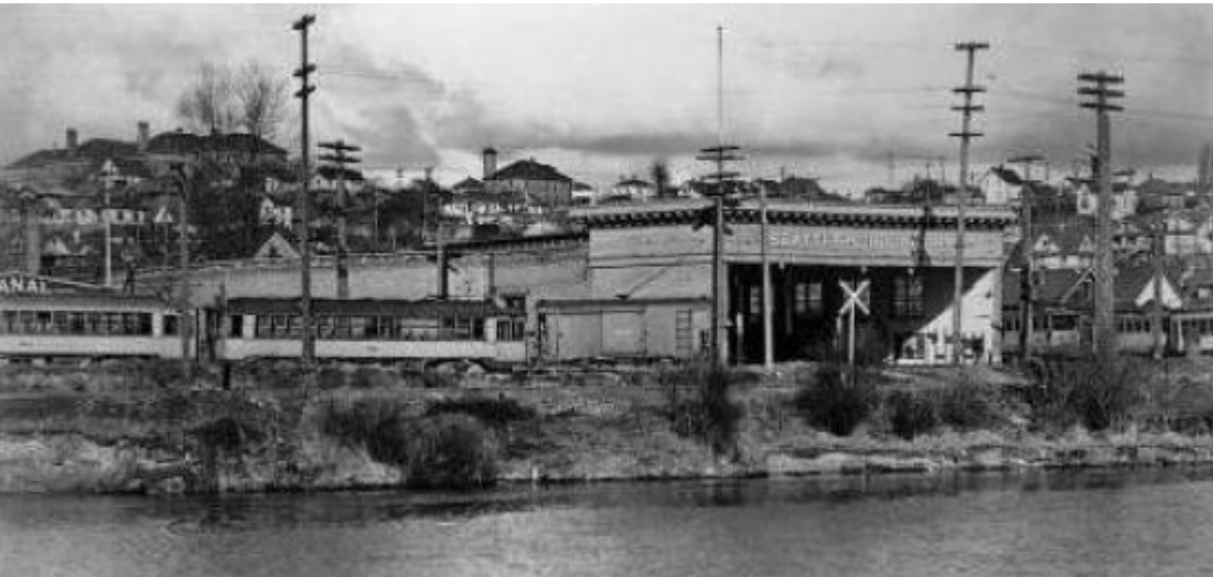
Original Structure—View From Canal
