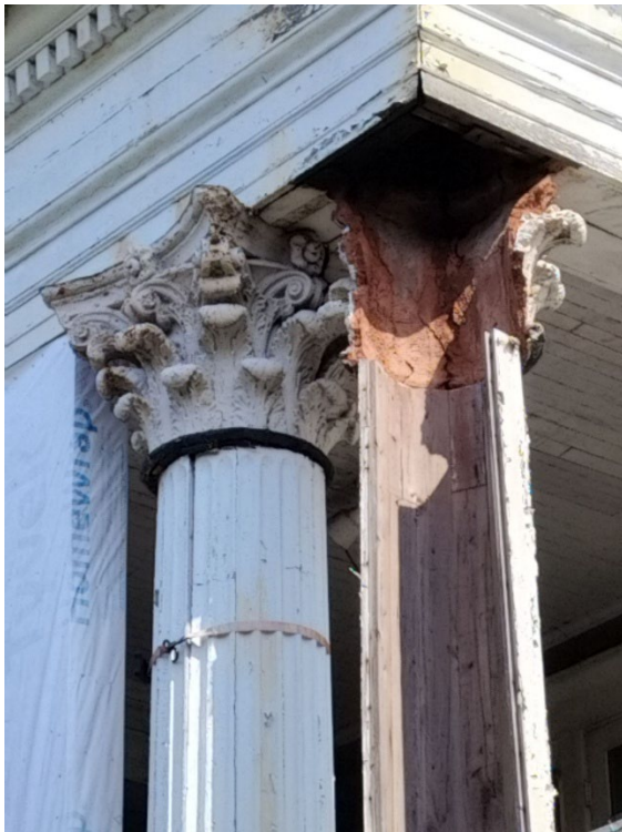
Wood and terra cotta column falling apart, other one strapped (left); older photo (right)
