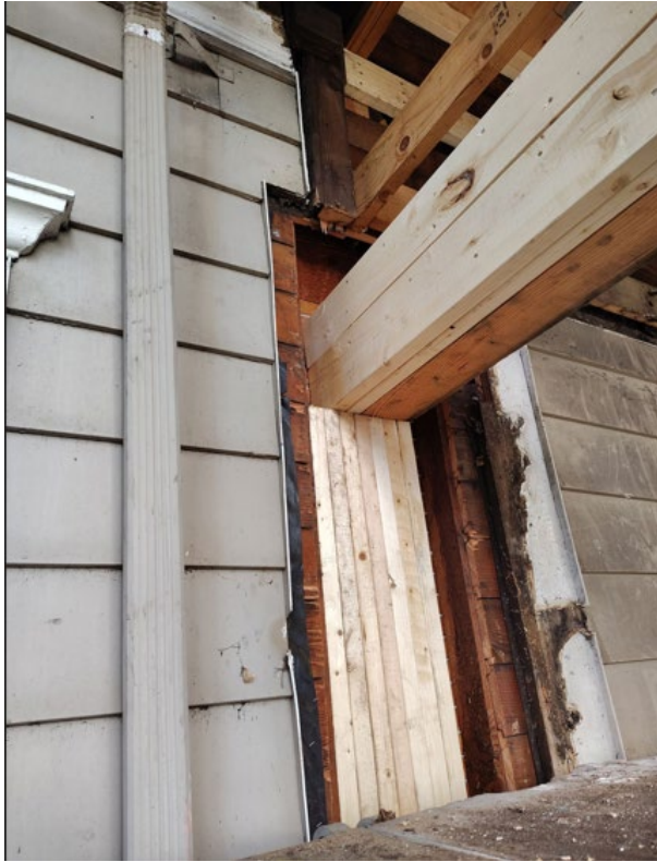
Following pilaster removal to build new structural supports and address water infiltration
