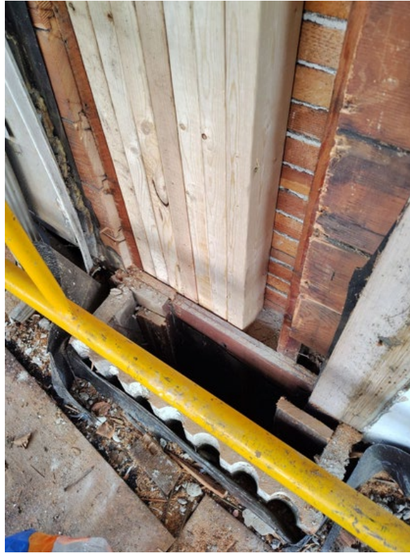
Following pilaster removal to build new structural supports and address water infiltration
