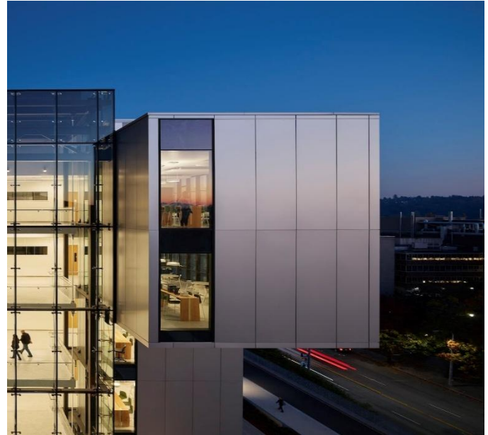
GFRC/fiberglass composite cladding on UW campus building
