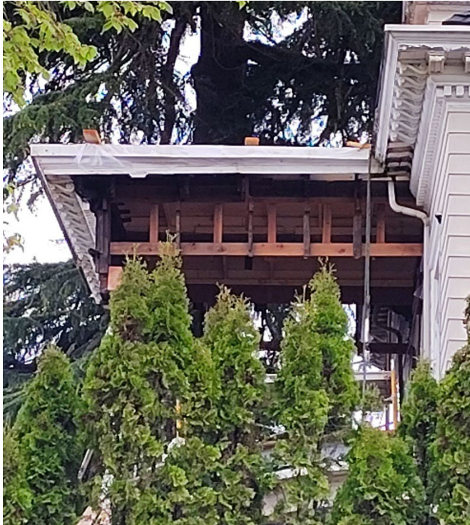
Reframing and sheathing the portico/belvedere in process
