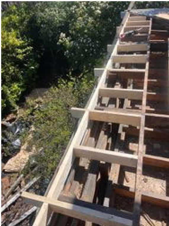
Reframing the roof of the lower porches in process
