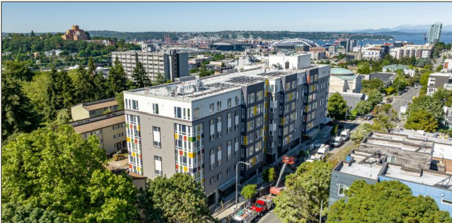
Bryant Manor Phase 1, 2024 Source: Compass Construction
