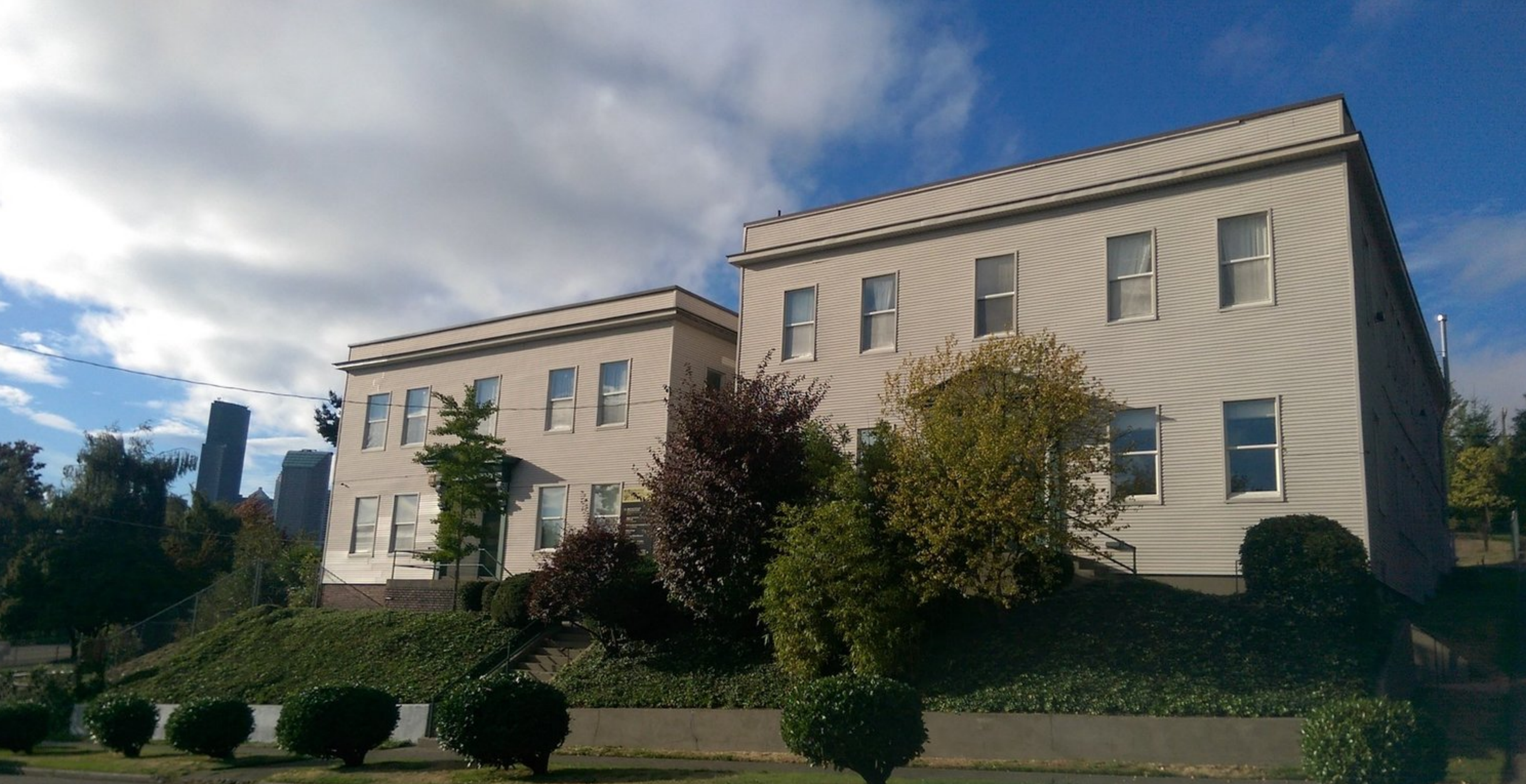
Building 1 and 2 View from South Weller Street
