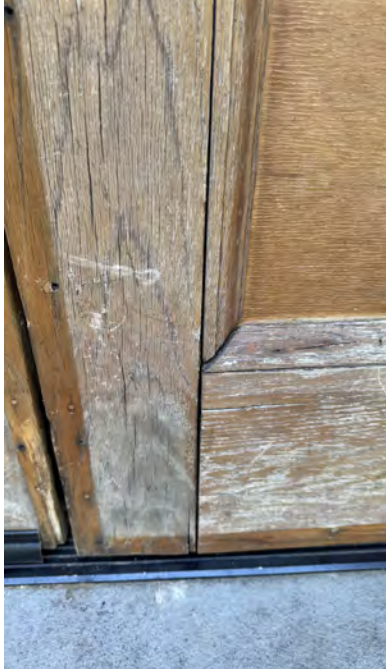
Fig. 34, 35, and 36: Damage from moisture infiltration of failing finishes at joints causing swelling and separation of components. Details of cupping and swelling wood components.
