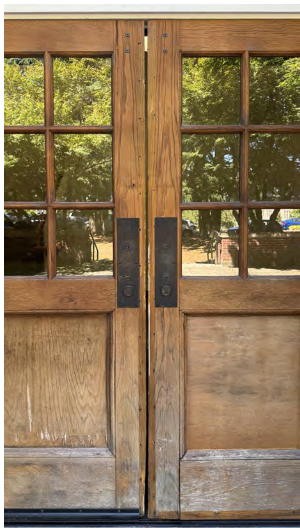
Fig. 30: Detail of doors S-ST02-06
