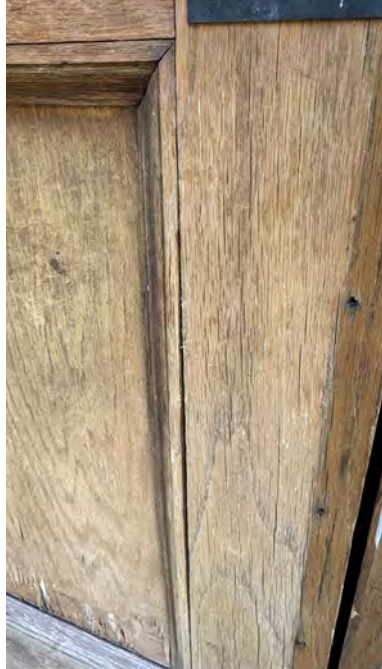
Fig. 34, 35, and 36: Damage from moisture infiltration of failing finishes at joints causing swelling and separation of components. Details of cupping and swelling wood components.
