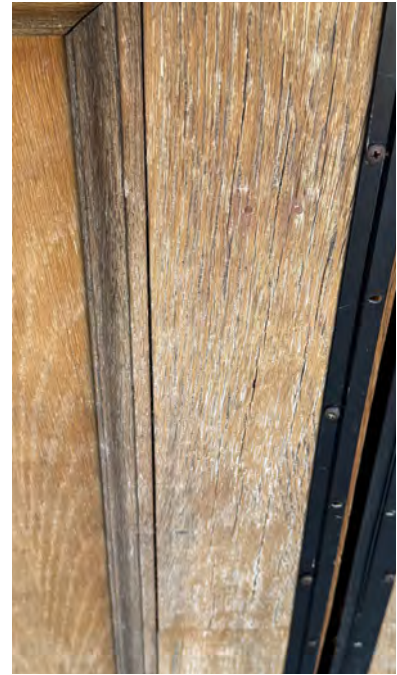
Fig. 51: Detail of dry and cracking wood.
