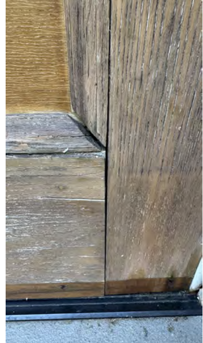
Fig. 34, 35, and 36: Damage from moisture infiltration of failing finishes at joints causing swelling and separation of components. Details of cupping and swelling wood components.
