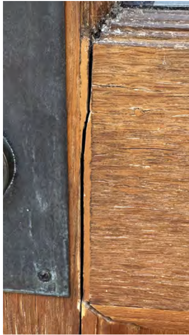
Figs. 49 & 50: Detail of failure of earlier door repair at stile to rail joint. Split occurring along length of stile connection.
