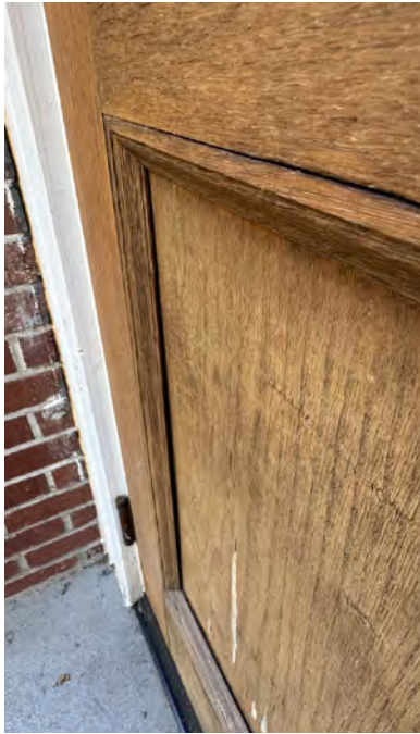
Fig. 31 & 32: Separation of door components from moisture infiltration.
