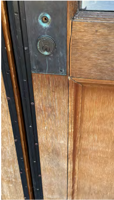
Figs. 49 & 50: Detail of failure of earlier door repair at stile to rail joint. Split occurring along length of stile connection.
