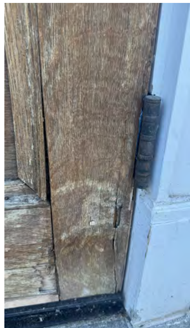
Fig. 81: Detail of loss of veneer material due to moisture & rot. These doors have also suffered damage from rocking and force.
