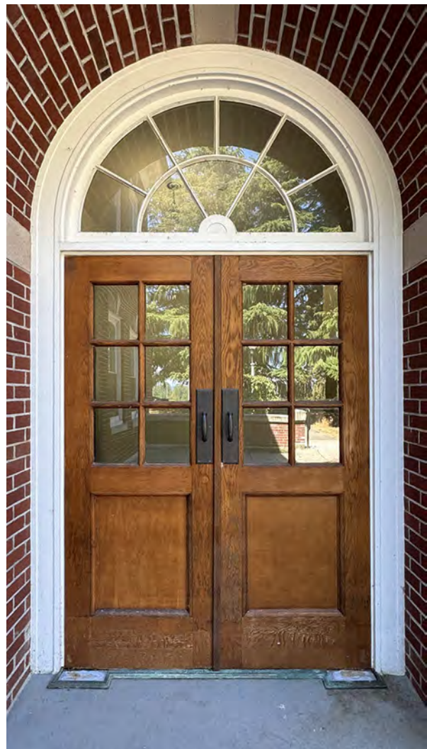
Fig. 09: Enlarged view of door pair S-ST03-05
