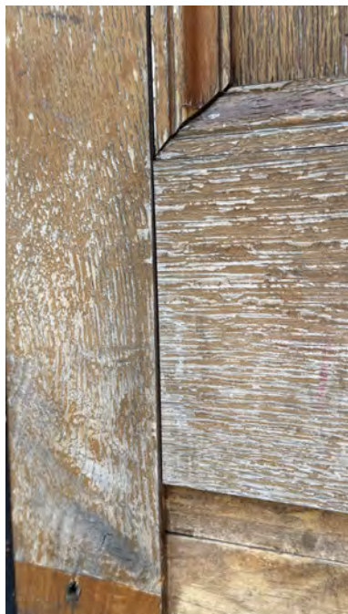
Fig. 53: Detail showing loss of veneer material at base.
