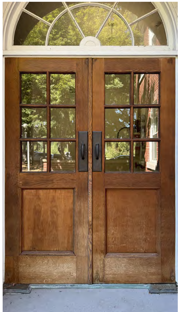
Fig. 38: Detail of door pair S-ST02-07
