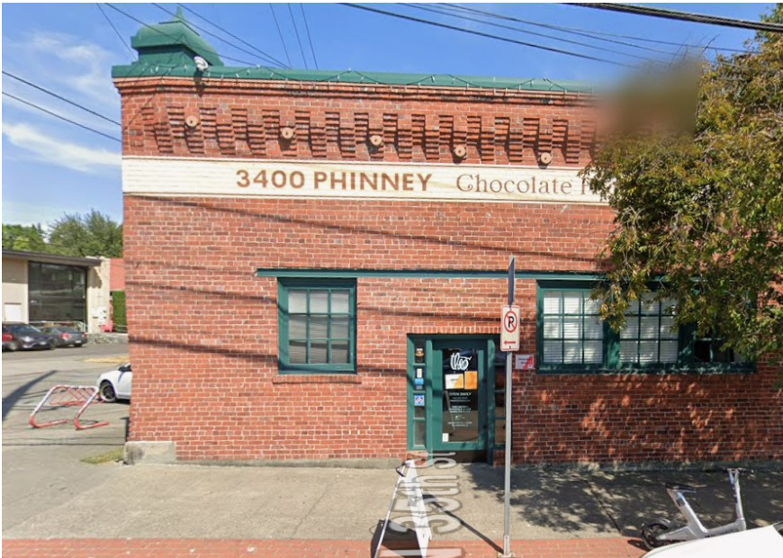
Current Signage—West Elevation
