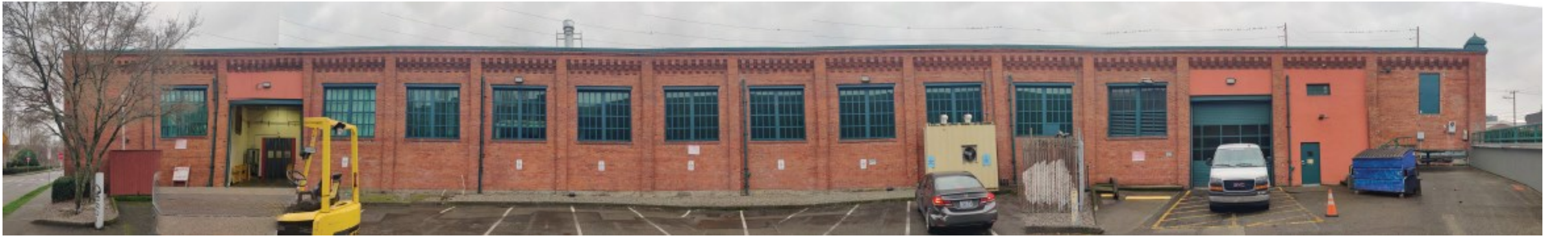
Prior Existing Condition—East Elevation
