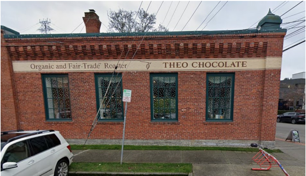
Current Signage—North Elevation
