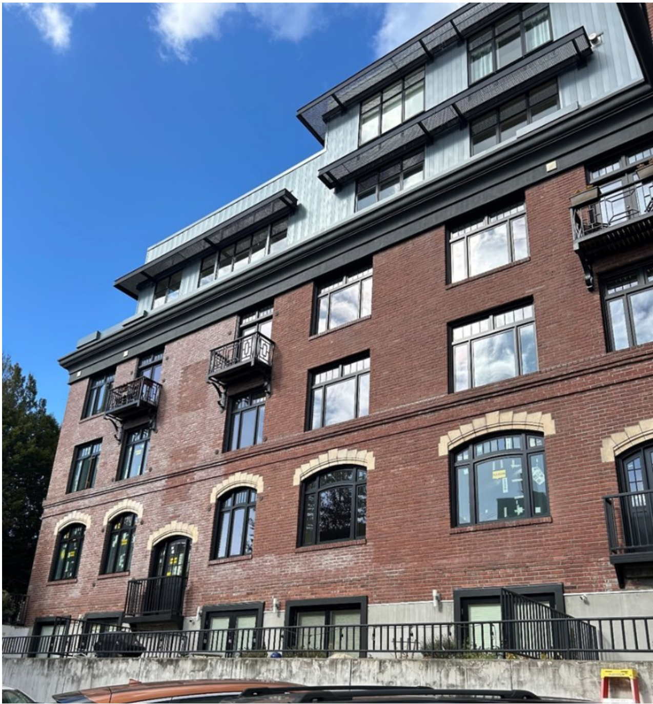
LEANONA CONDOMINIUMS WITH LPB APPROVED WINDOWS
