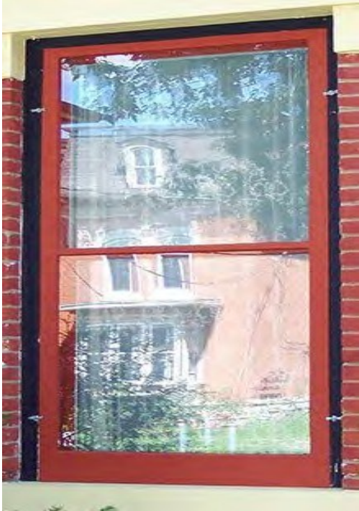
Rehabilitate with full overlay storm windows
