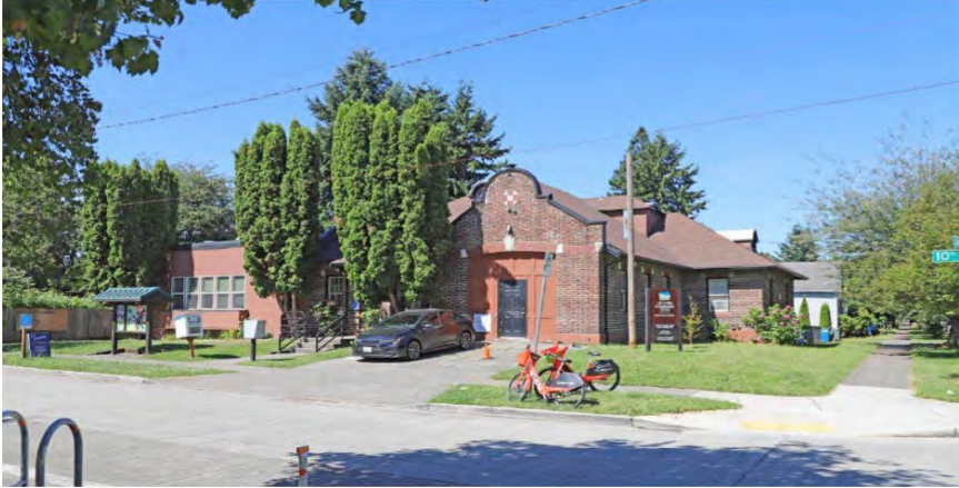
Contemporary photo – East and North sides
