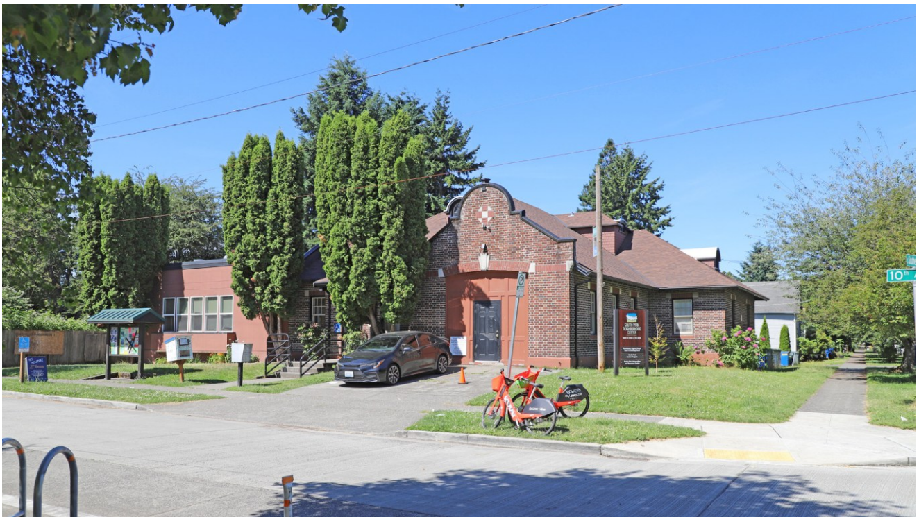
Contemporary photo – East and North sides
