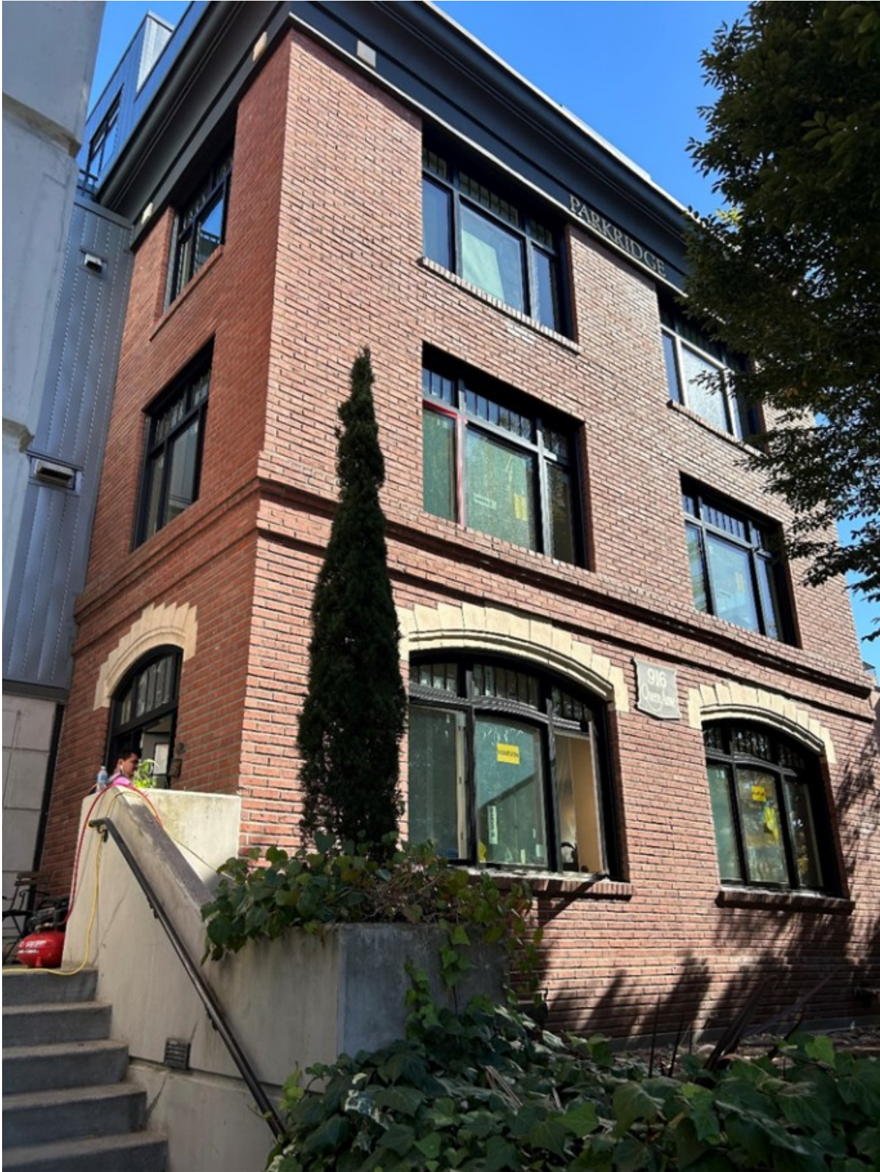
LEANONA CONDOMINIUMS WITH LPB APPROVED WINDOWS
