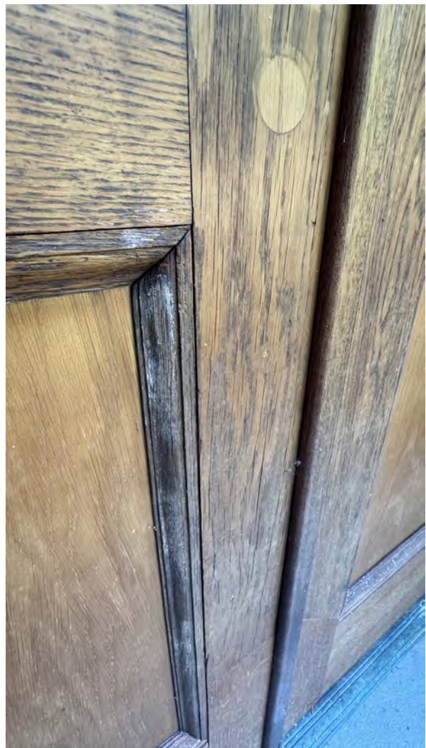
Fig. 28: Discoloration of wood from loss of protective finish.
