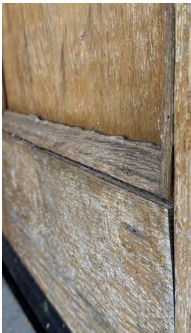
Fig. 52: Detail showing cupping of veneer from drying.
