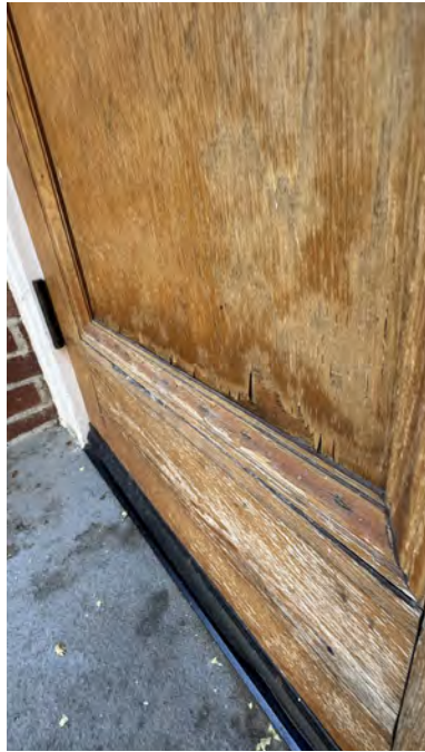
Figs. 16 & 17: Damage from moisture infiltration at failing seals at joints causing swelling and separation of components.
