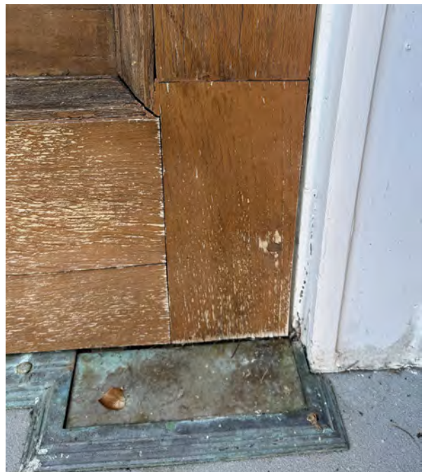
Fig. 59: detail of wood patch at base of door.
