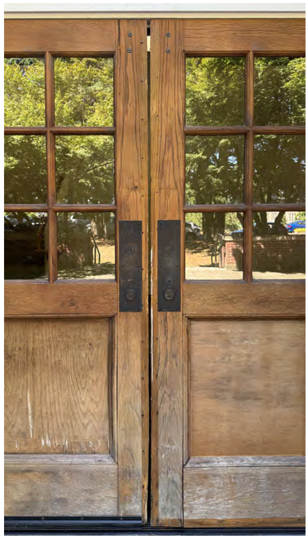
Fig. 30: Detail of doors S-ST02-06
