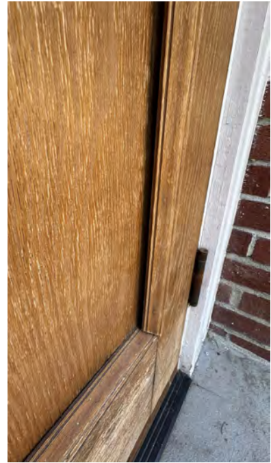
Figs. 16 & 17: Damage from moisture infiltration at failing seals at joints causing swelling and separation of components.
