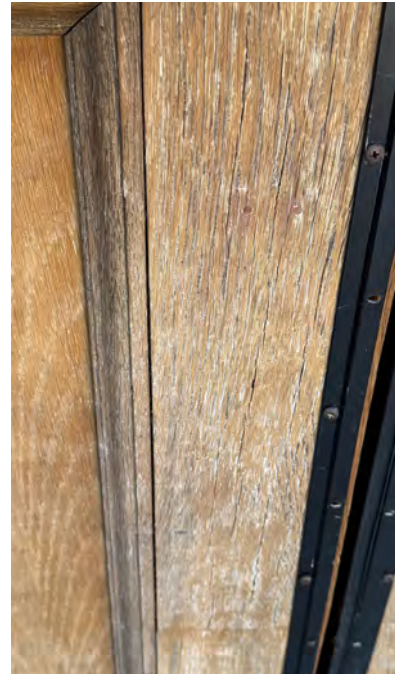
Fig. 51: Detail of dry and cracking wood.
