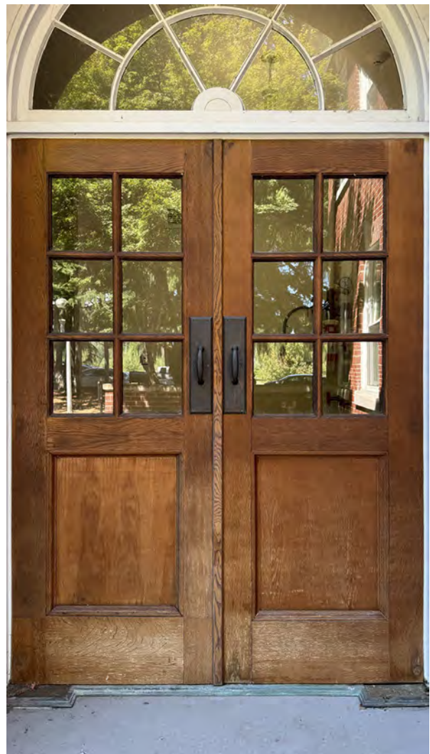
Fig. 38: Detail of door pair S-ST02-07
