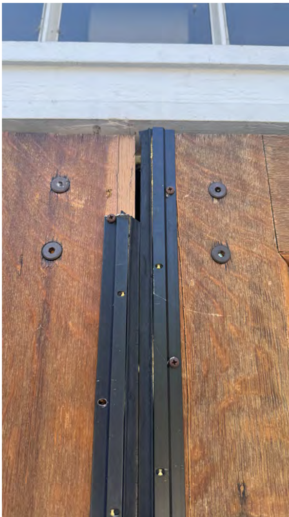
Fig. 75: Loss of portion of astragal in effort to gain access.
