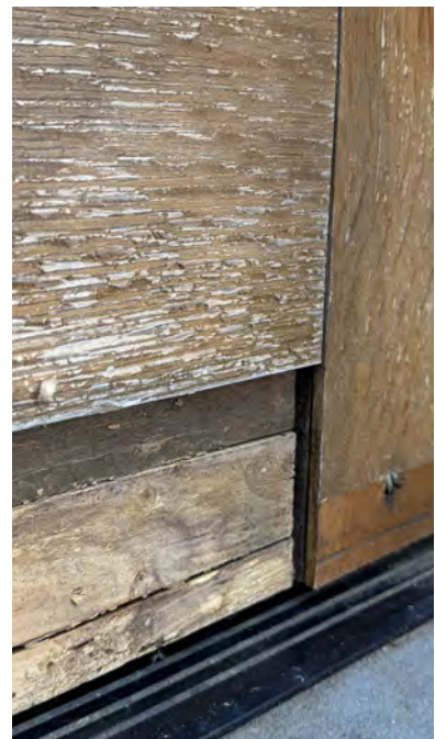
Fig. 54: Detail showing loss of veneer material at base.
