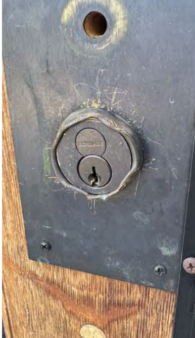
Fig. 88: Detail of damage to locks.
