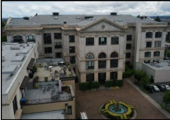
Building 1. South elevation, facing northeast.
