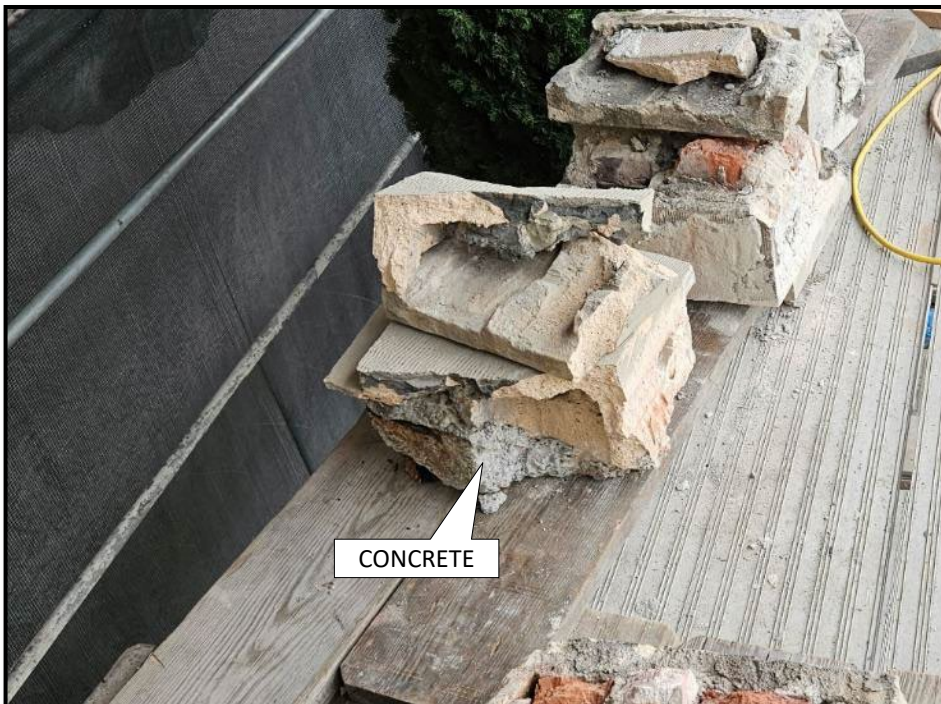
Terra cotta unit cells filled with concrete.
