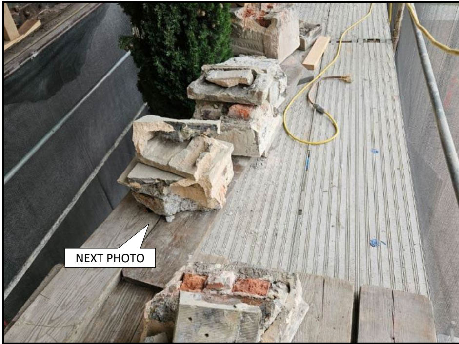
Photo A.1. Terra cotta units removed.
