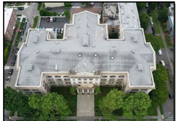
Building 1. North elevation and roof.
