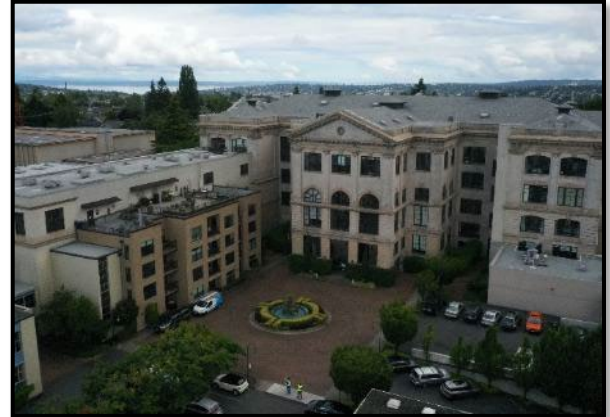
Building 1. South elevation, facing northwest
