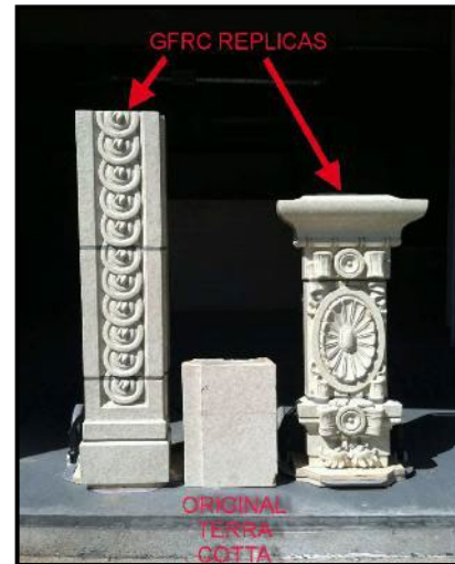
EXAMPLE OF GFRC REPLACING TERRA COTTA AT NORDSTROM BUILDING, SEATTLE
