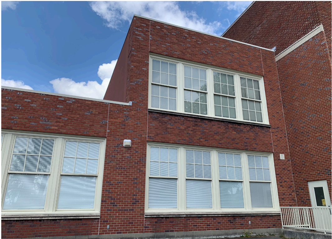
VIEW OF 2000 ADDITION FROM PLAY AREA
