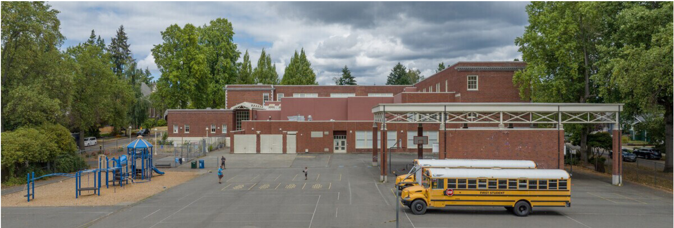
VIEW OF SOUTHERN ELEVATION
