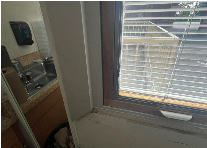
Sash deterioration
