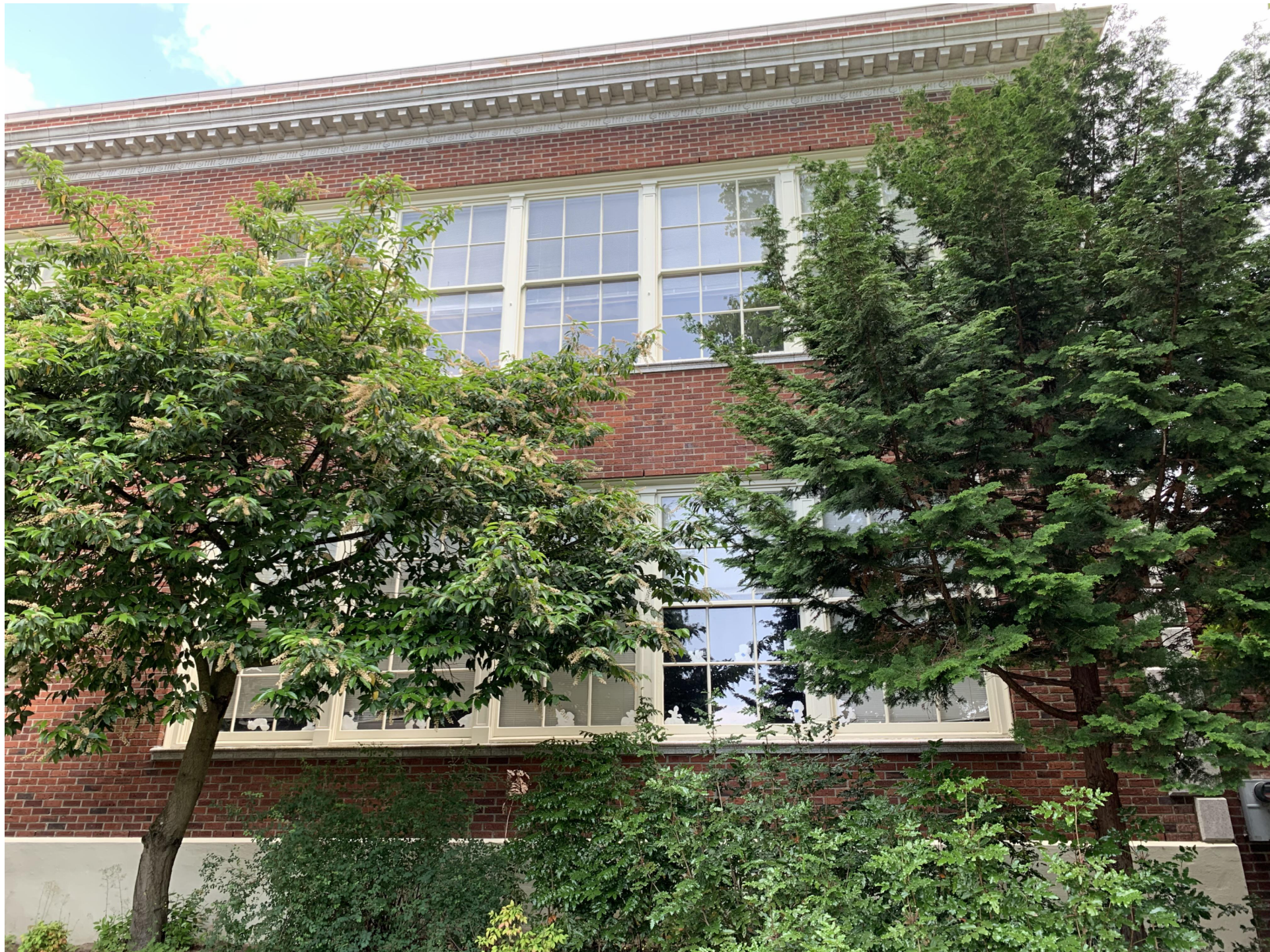
G. WESTERN FACADE TREE COVER
