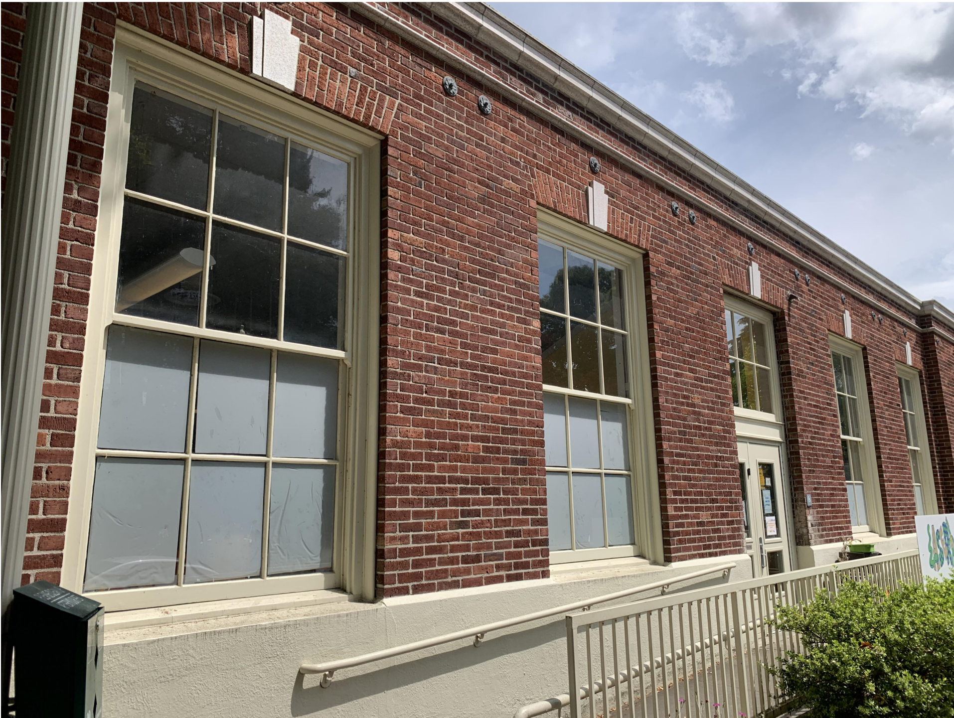
H. RAMP AT WESTERN FACADE
