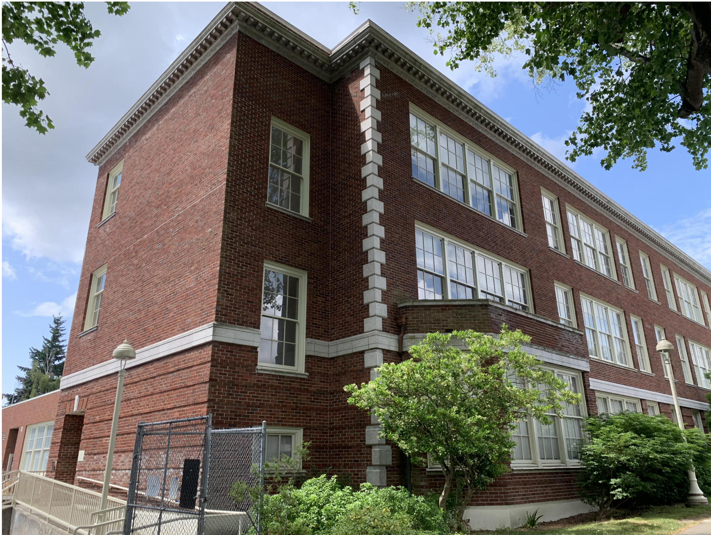
I. SOUTH EASTERN BUILDING CORNER
