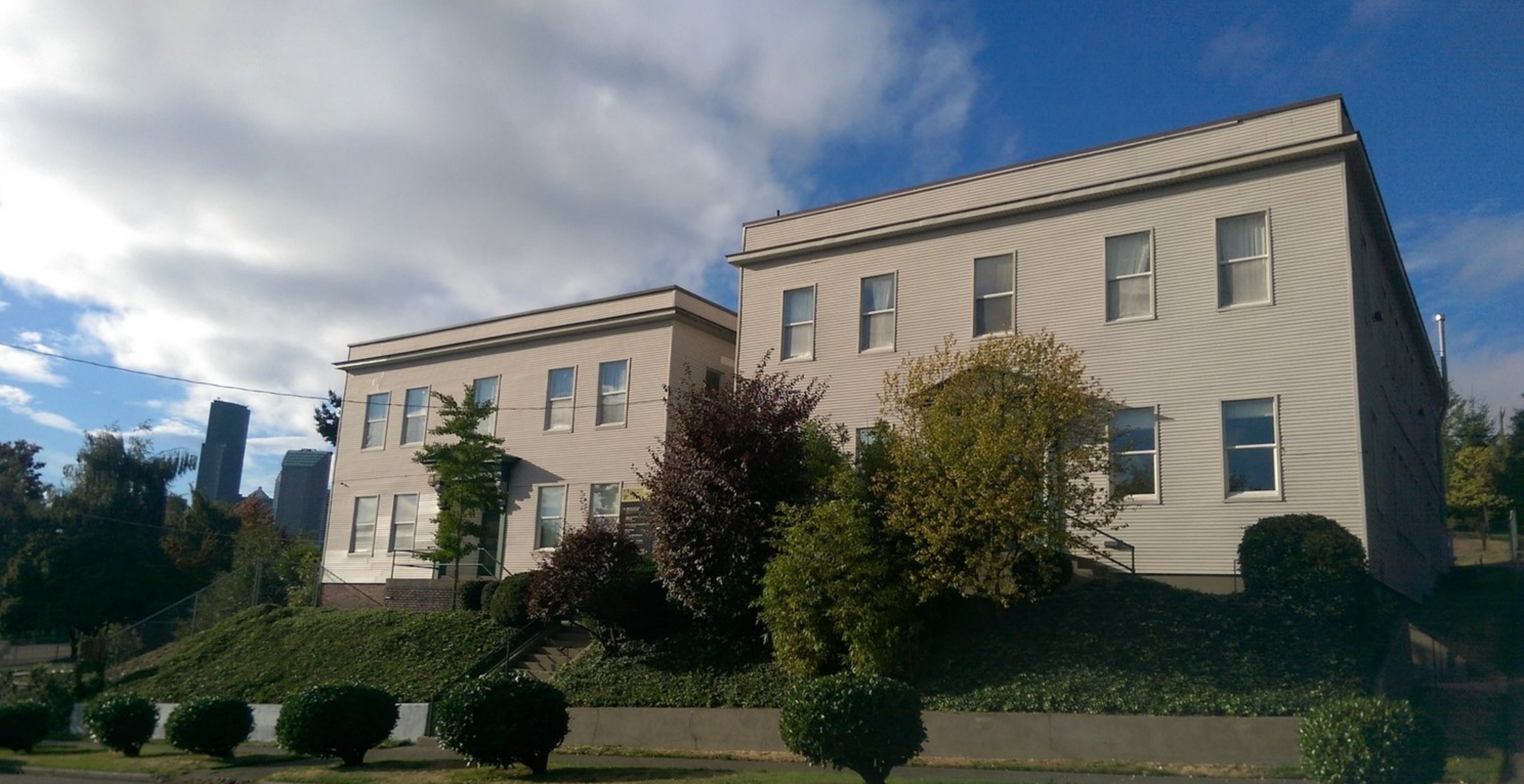
Building 1 and 2 View from South Weller Street
