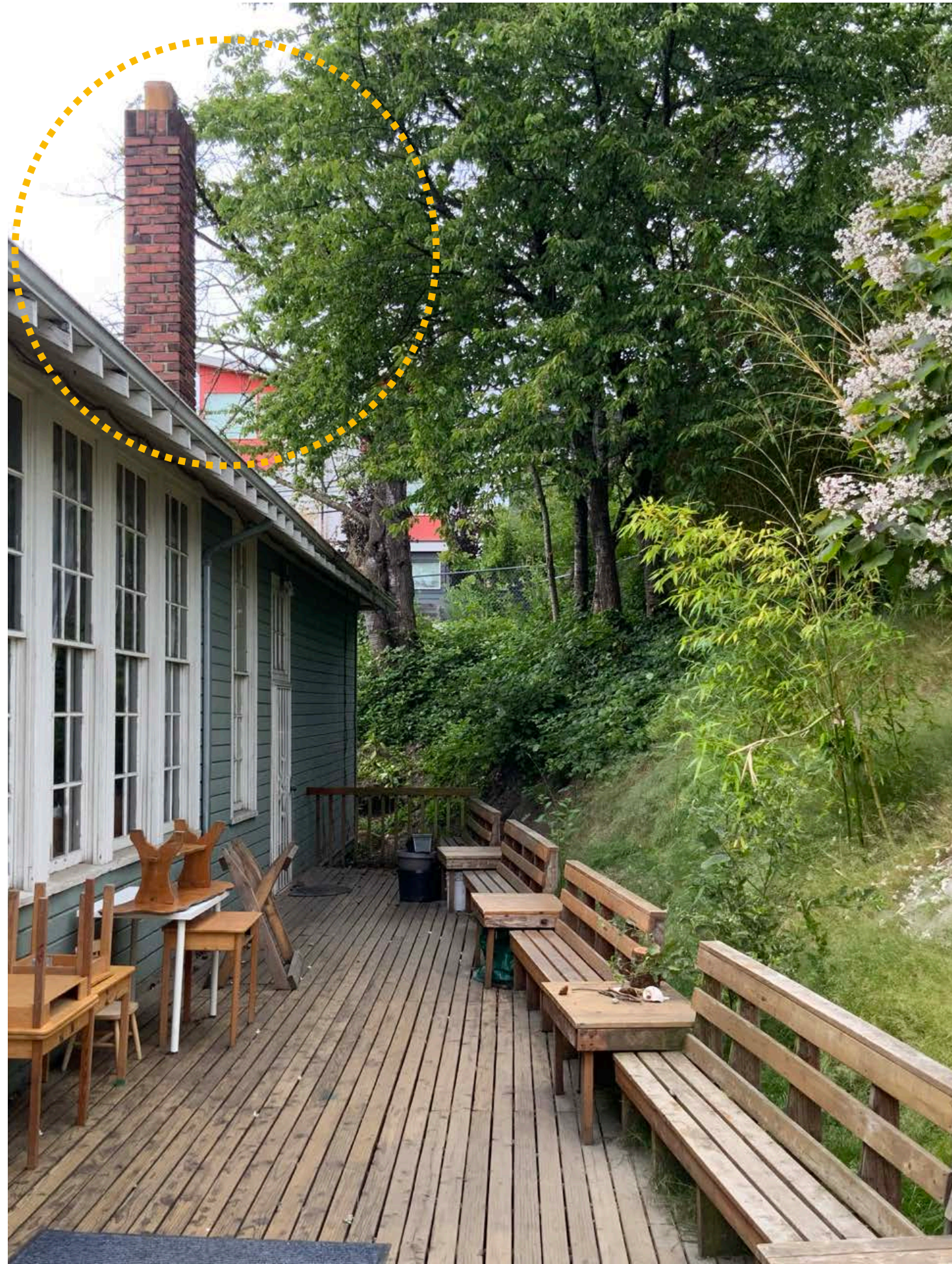
Hazard for students playing outside on the outdoor deck
