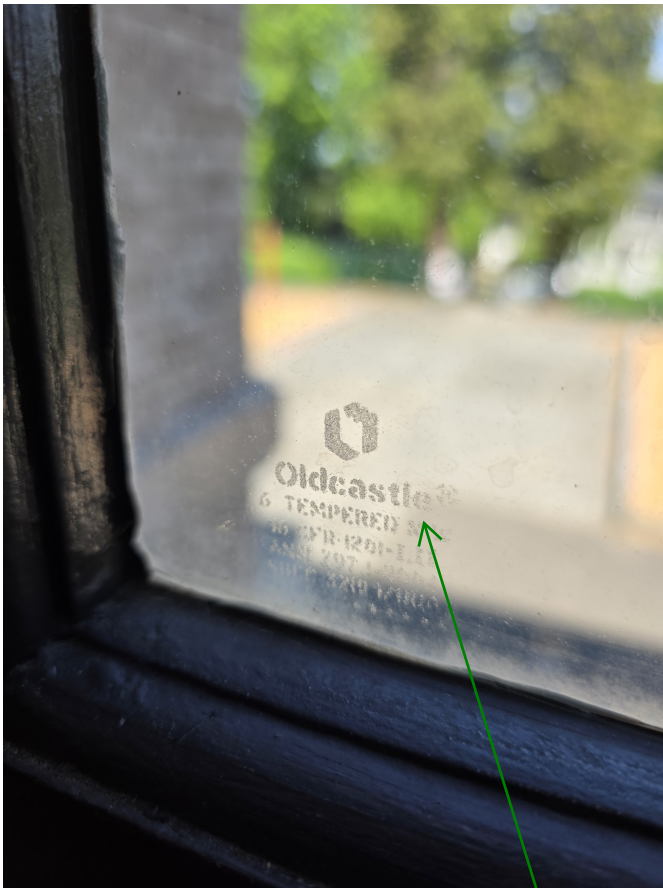
Previously replaced window glazing
