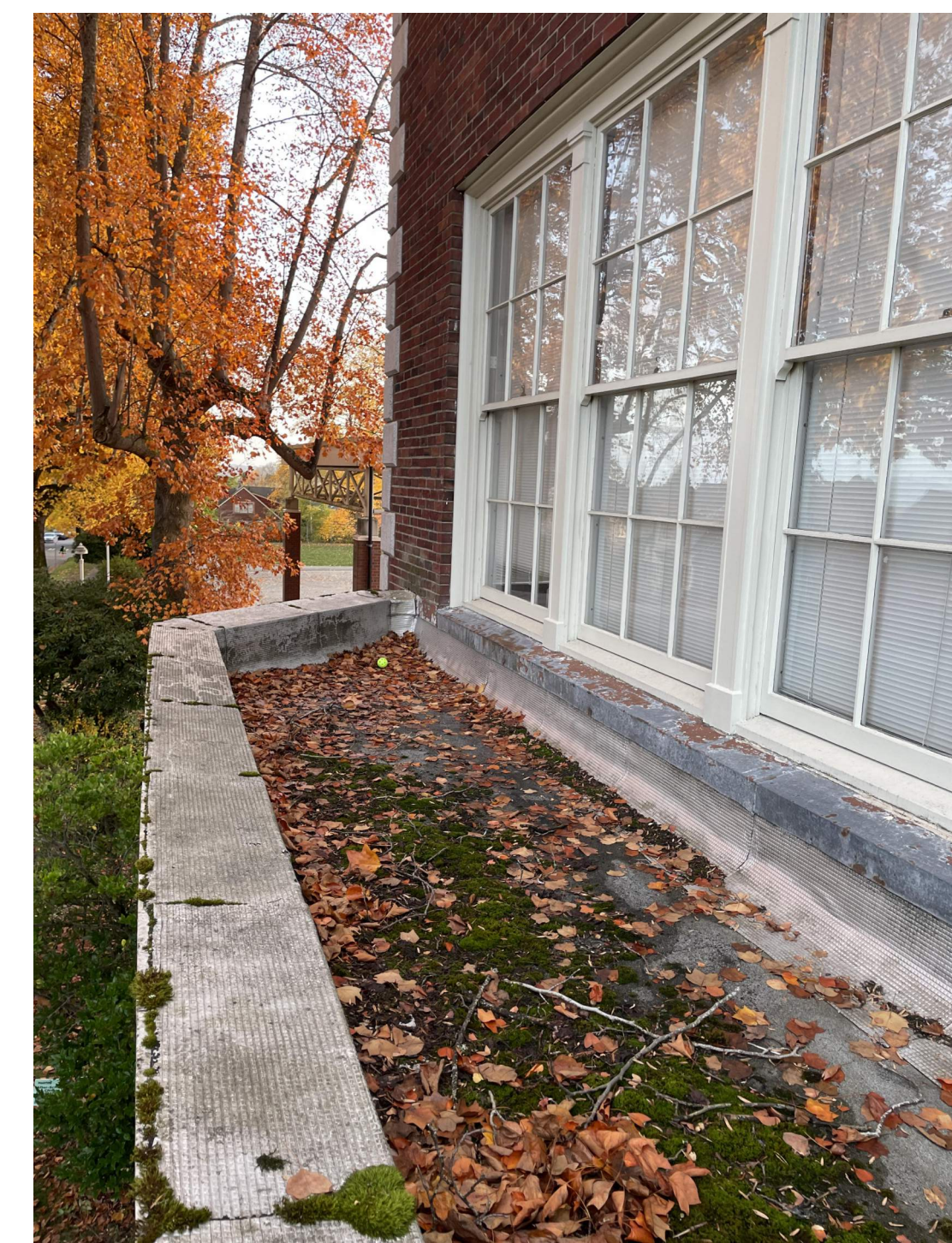
I. (E) KINDERGARTEN BAY ROOF
