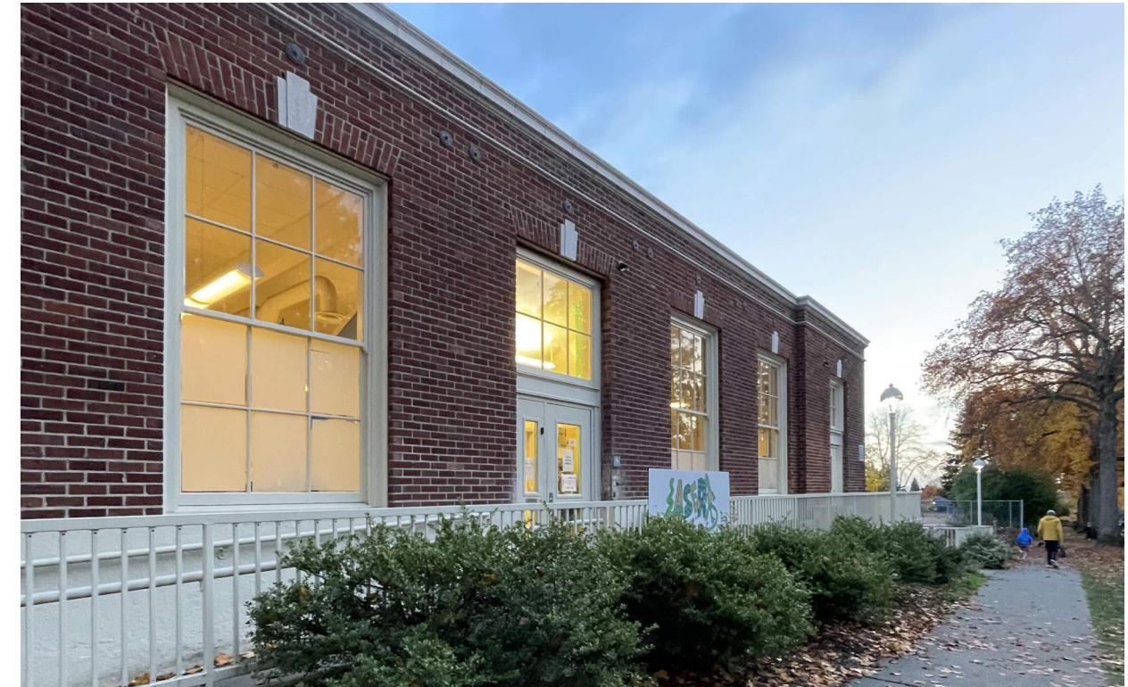
VIEW OF HISTORIC WINDOWS ON WESTERN ELEVATION
