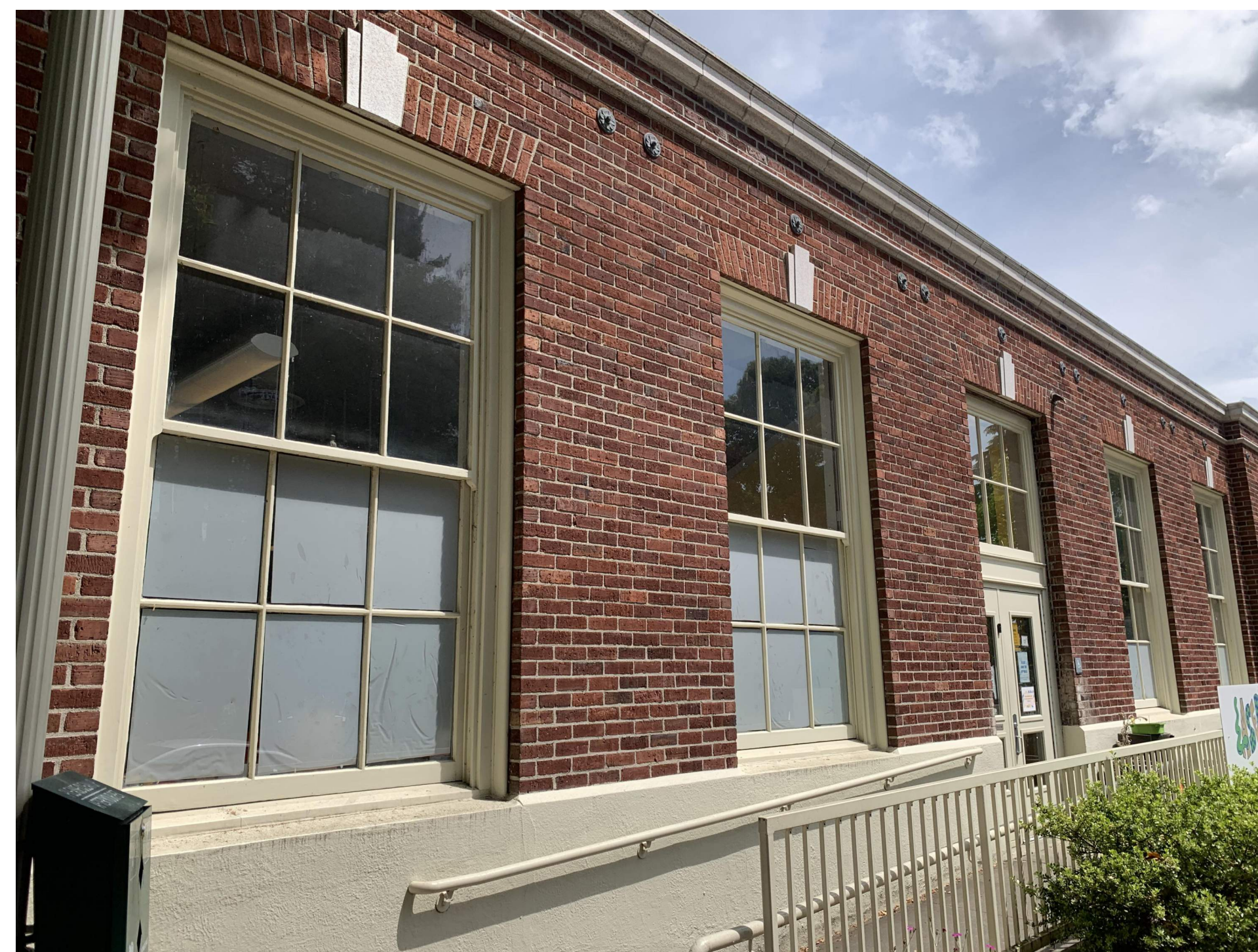
H. RAMP AT WESTERN FACADE
