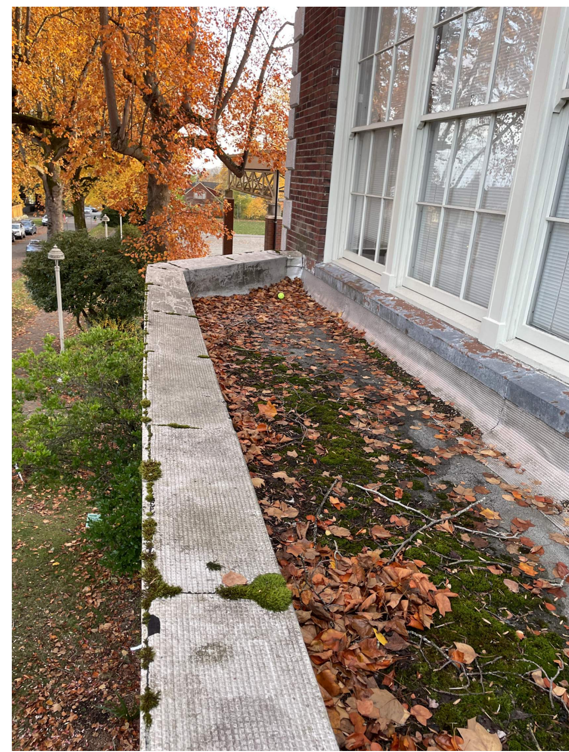
(E) KINDERGARTEN BAY ROOF EXISTING CONDITION
