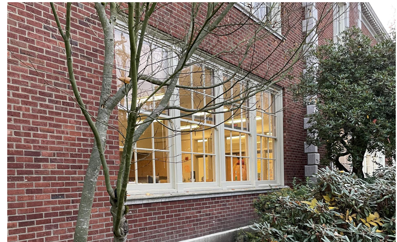
VIEW OF HISTORIC WINDOWS ON EASTERN ELEVATION
