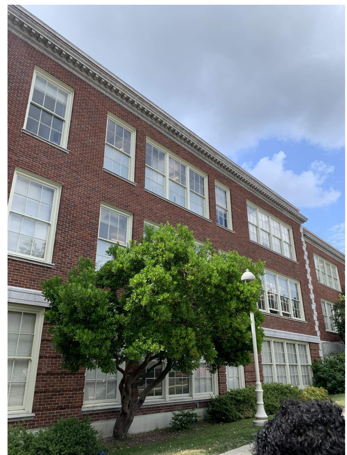
F. EASTERN FACADE TREE COVER (S)
