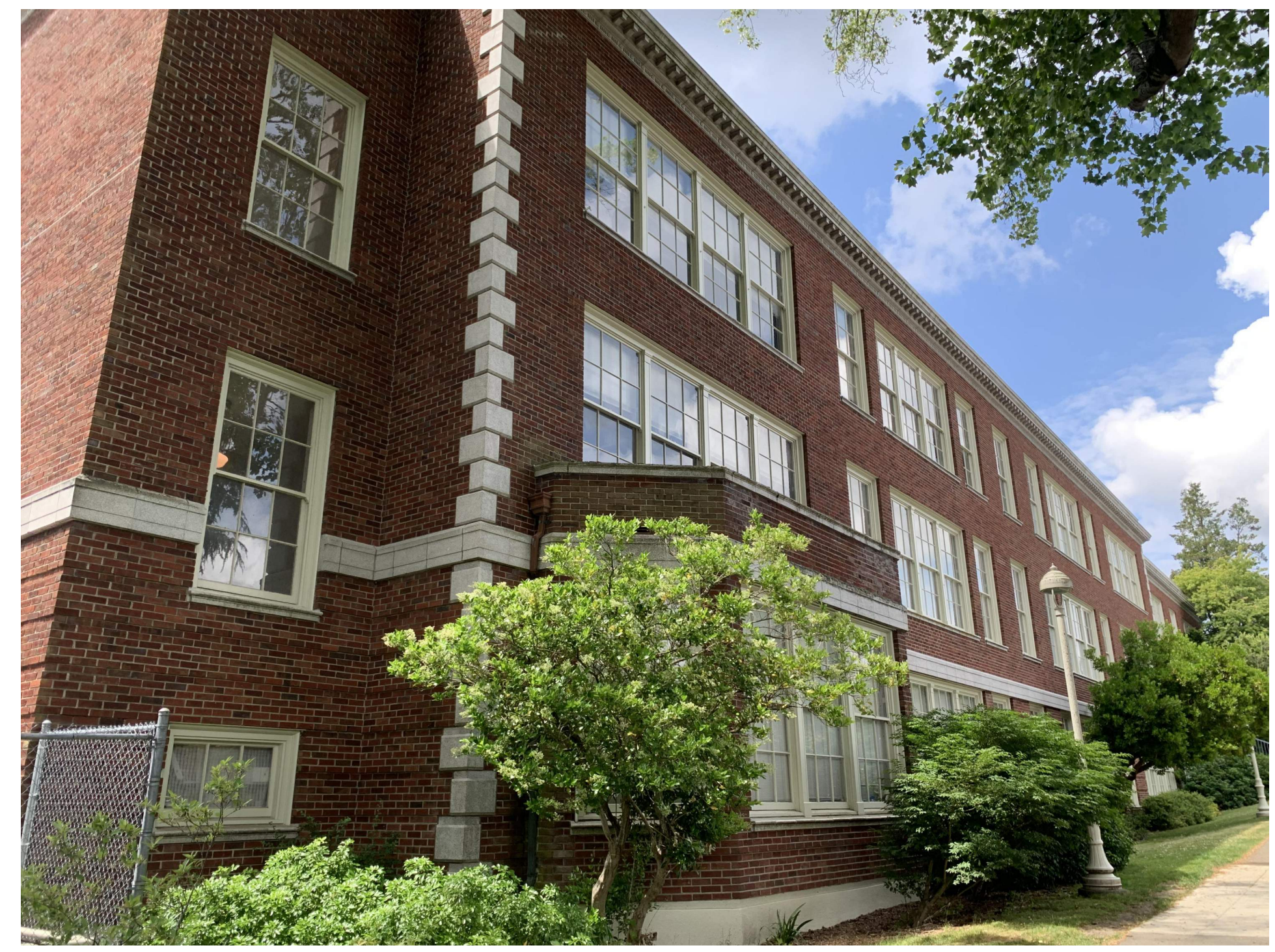
E. (E) KINDERGARTEN BAY EXTERIOR
