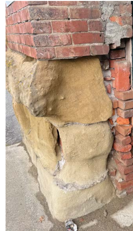
Close up of sandstone plinth
