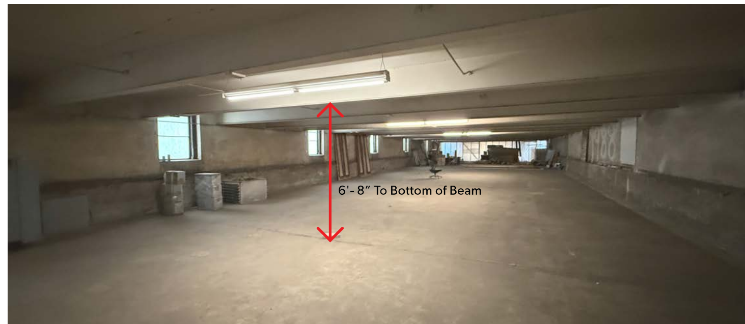
Drying malts required minimal penetrations in the facade. Current standards for re-purposing these spaces into other uses, such as residential, would be limited by the current configuration of windows.
