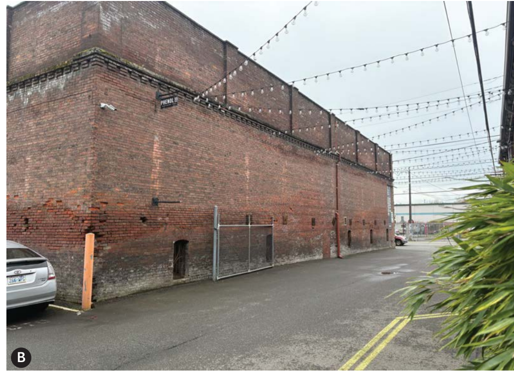
NORTH FACADE - ALLEY WITH BOTTLING PLANT
