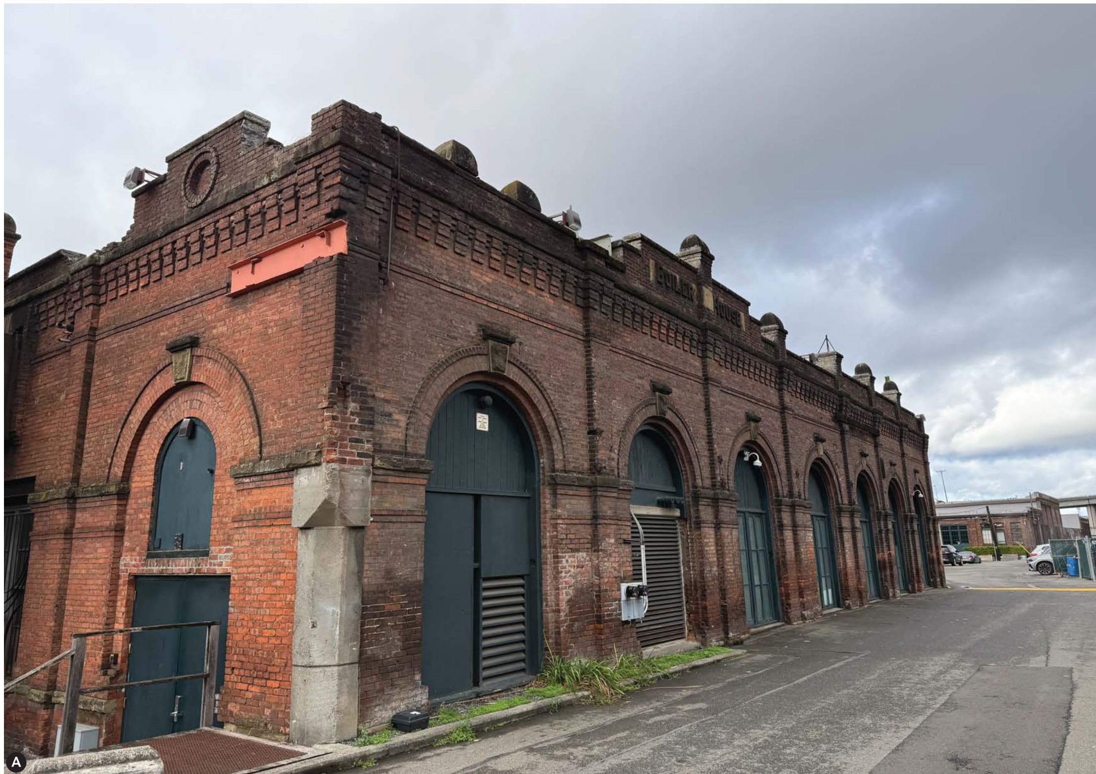
EAST FACADE - BSNF RAILWAY
