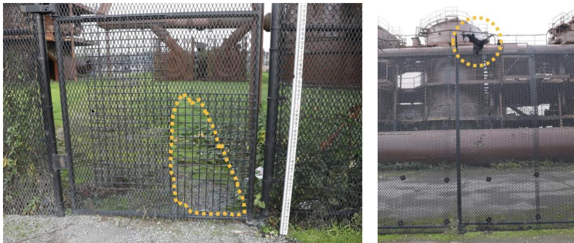
Figure 6. Photographs taken during GEAR’s November 12, 2025, site inspection. Left ) A photograph depicting a missing section of metal fencing on the west perimeter (with additional metal-grating welded over the missing section). Right ) A partially torn/ripped garment on the barbed wire at the top of the fencing on the east perimeter.
