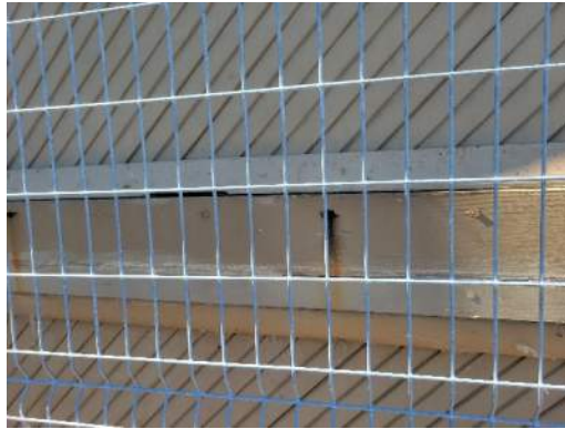
Photo 13 – Corroded fasteners
