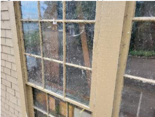
Figure 2 - xC1 Glass soiling
