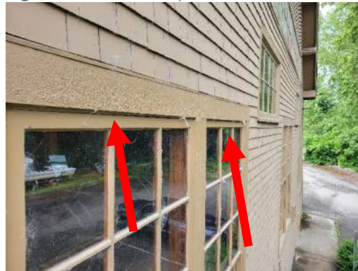
Figure 5 - xD1 & xD2 Misalignment at fixed upper sash.
