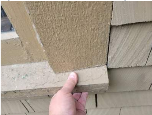
Figure 11- xE2 Loose sill connection
