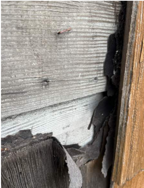
EXISTING ORIGINAL HORIZONTAL SIDING UNDER 1980-ERA SHINGLES
