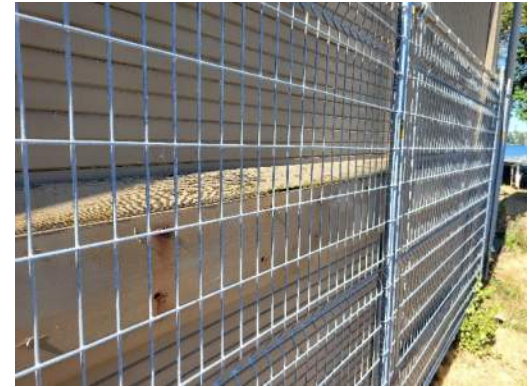
Photo 16 – Corroded fasteners
