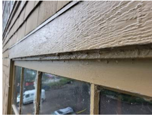
Figure 13 - xE2 sealant repairs
