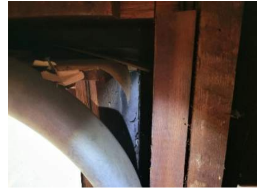
Figure 7 - xC3 Close up of cut frame at conduit.
