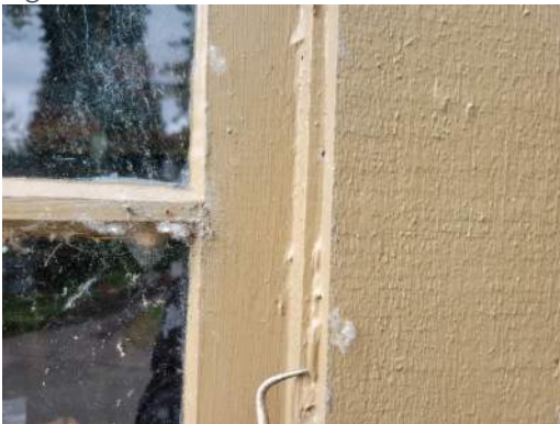
Figure 12- xE2 sealant repairs
