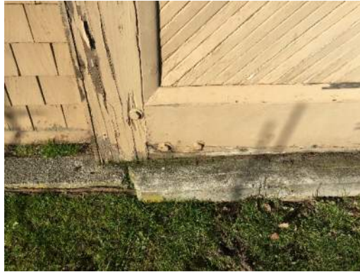
Photo 4 - Dry rot at Door A sill
