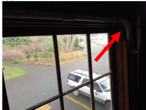
Figure 6 - Cut out at top corner frame for conduit clearance.
