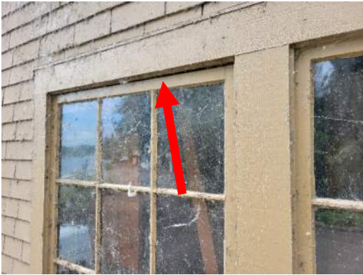
Figure 1 - xC1 misaligned upper sash
