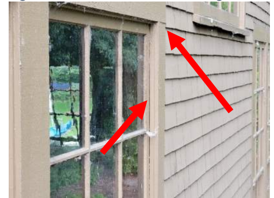
Figure 9 - xC4 minor misalignment at jamb
