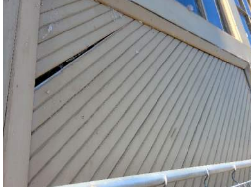
Photo 14 – Damaged infill panel
