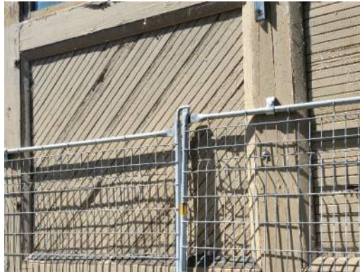
Photo 6 - Deteriorated Wood Infill
