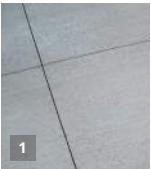
Pedestrian Concrete CIP CONC BROOMED FINISH ACCESSIBLE PATH
