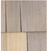
CEDAR SHINGLE SHAKERTOWN STORM GRAY (SEMI-TRANSPARENT) EAST & WEST FACADE SIDING
