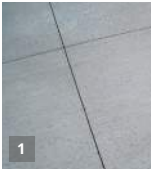
Pedestrian Concrete CAST-IN-PLACE LIGHT BROOMED FINISH ACCESSIBLE PATH
