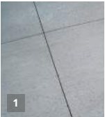
Vehicular Concrete CAST-IN-PLACE LIGHT BROOMED FINISH FIRE ACCESS TURNAROUND
