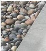
Gravel Filter Strip COBBLE AND GRAVEL FILTER STRIP BELOW CONCRETE WALK
