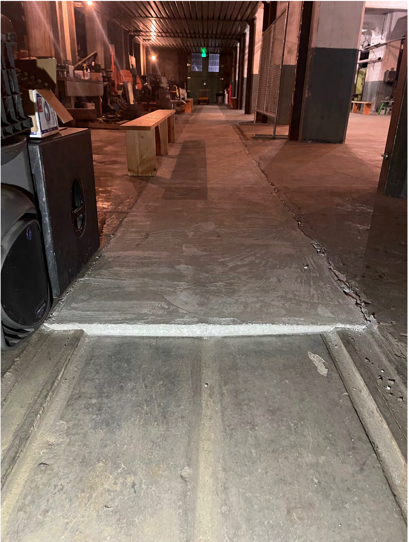
Ash Cart Track East Ash Room with Completed Concrete Infill Looking South. Showing North Extent Preserving Open Trackway for Interpretation While Other Sections Are Filled. Also Showing Section View Of Poured Concrete at North Extent.
