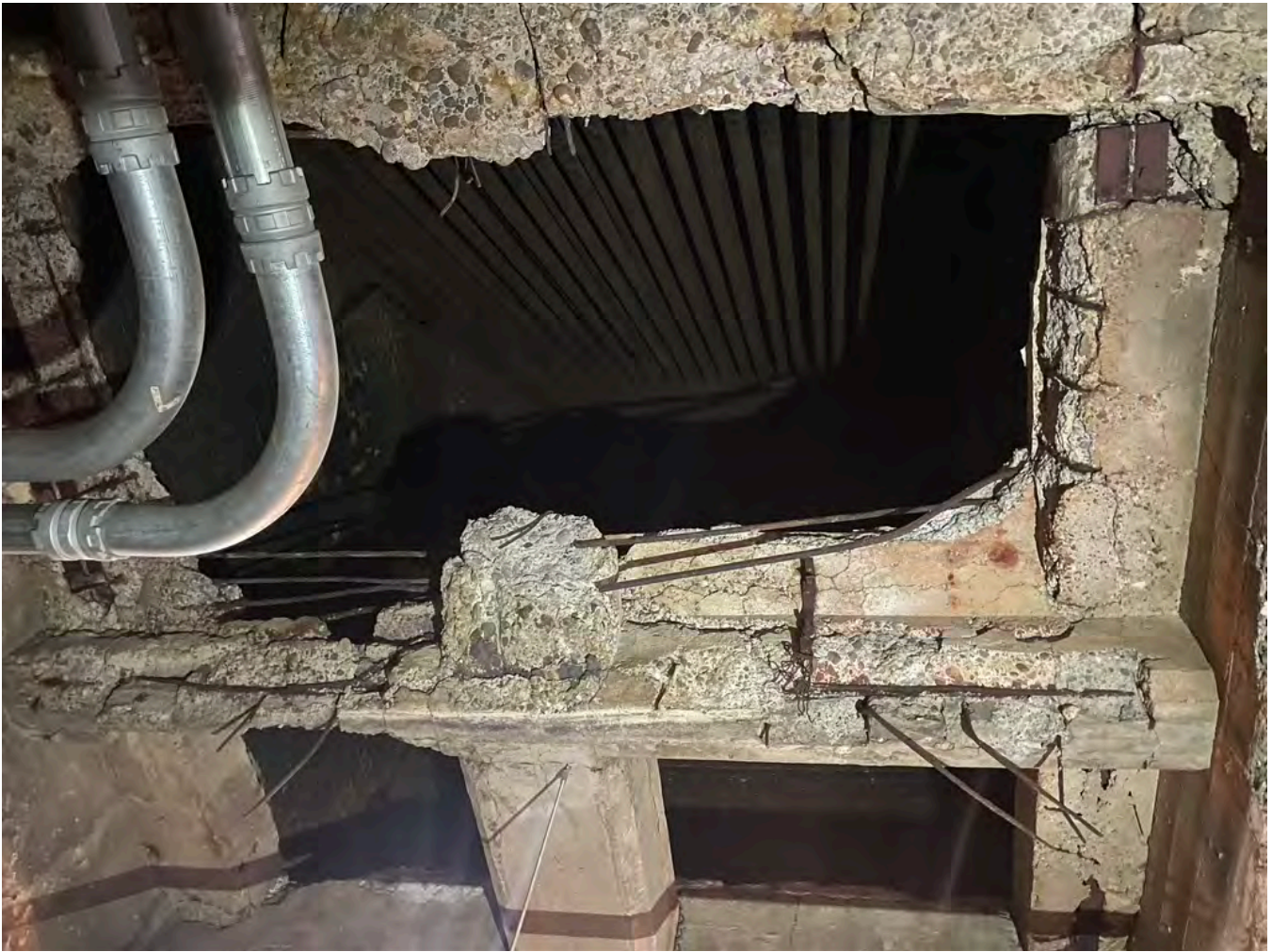
Boiler Floor/Ash Hopper After Loose Brick and Debris Removal
