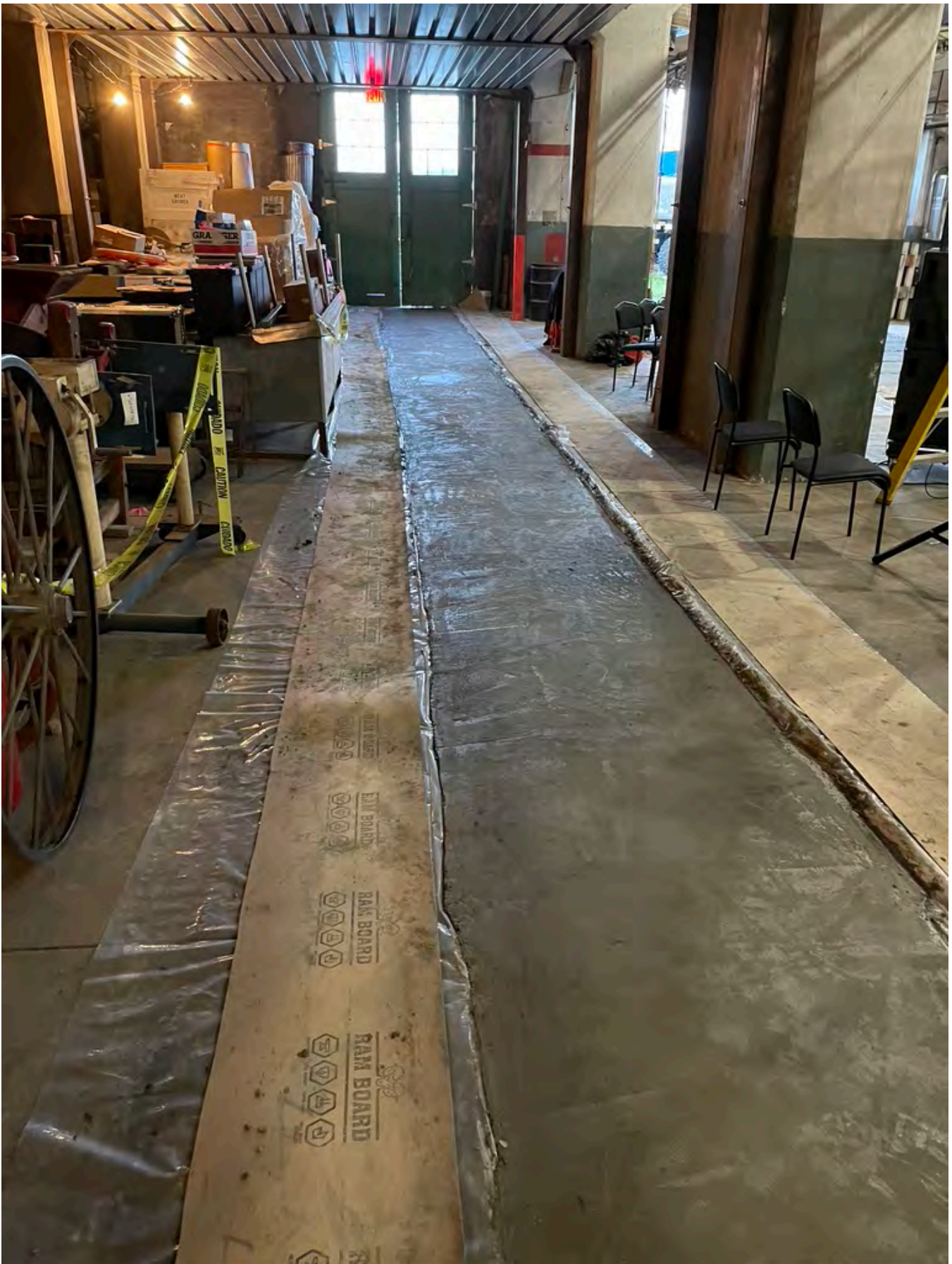
Ash Cart Track East Ash Room Looking South During Concrete Pour And Finishing
