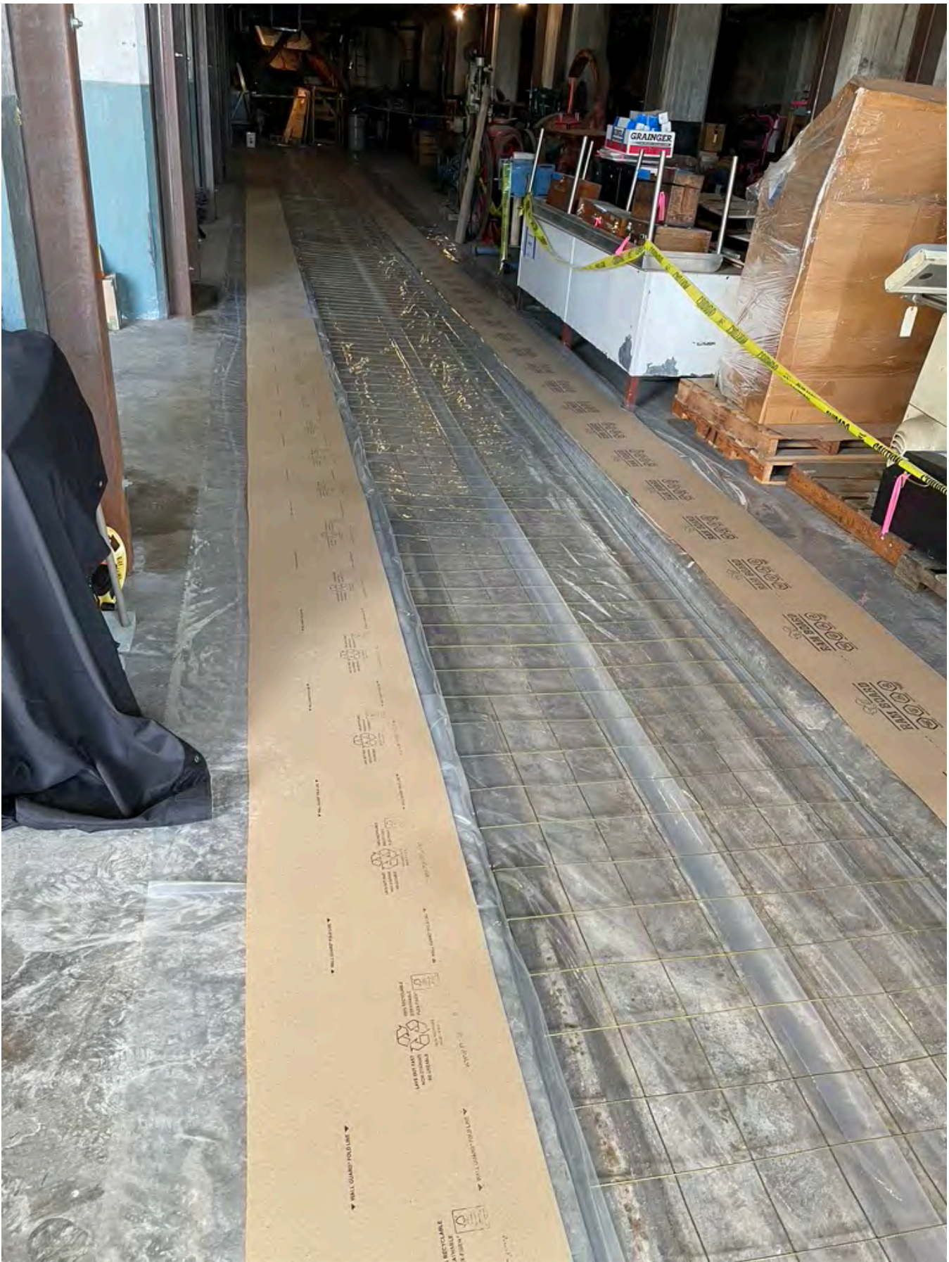
Ash Cart Track East Side Prepped for Concrete Pour with 6mil plastic sheeting for separation from existing trackway and track protection of surrounding areas during pour. Steel reinforcing mesh for concrete strengthening and ram board on each side for protection during pour. Standard prep on all track infill areas.
