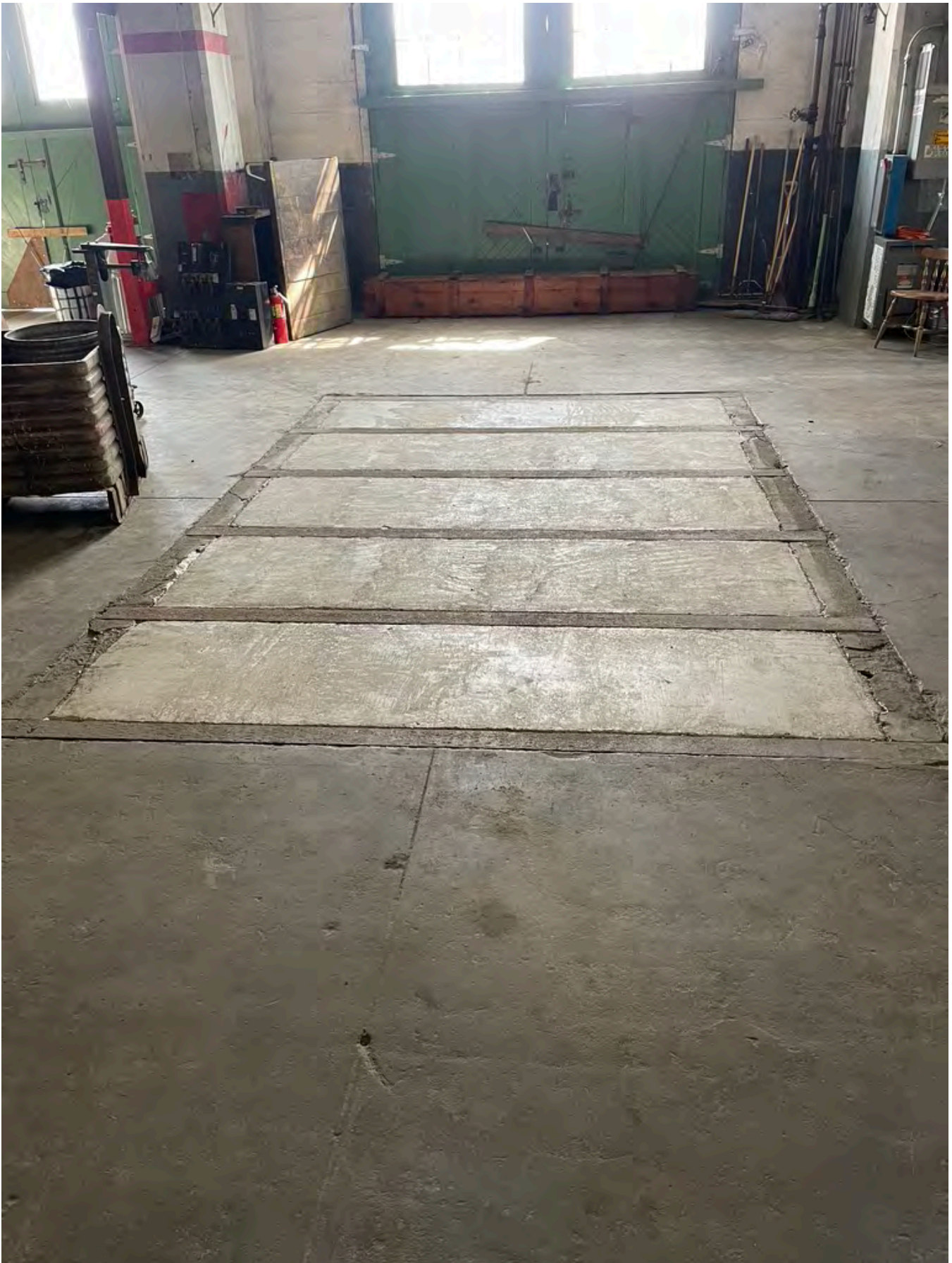
Fished Concrete Infill Over Debris Pile In Pipe Trench In Ash Room.
