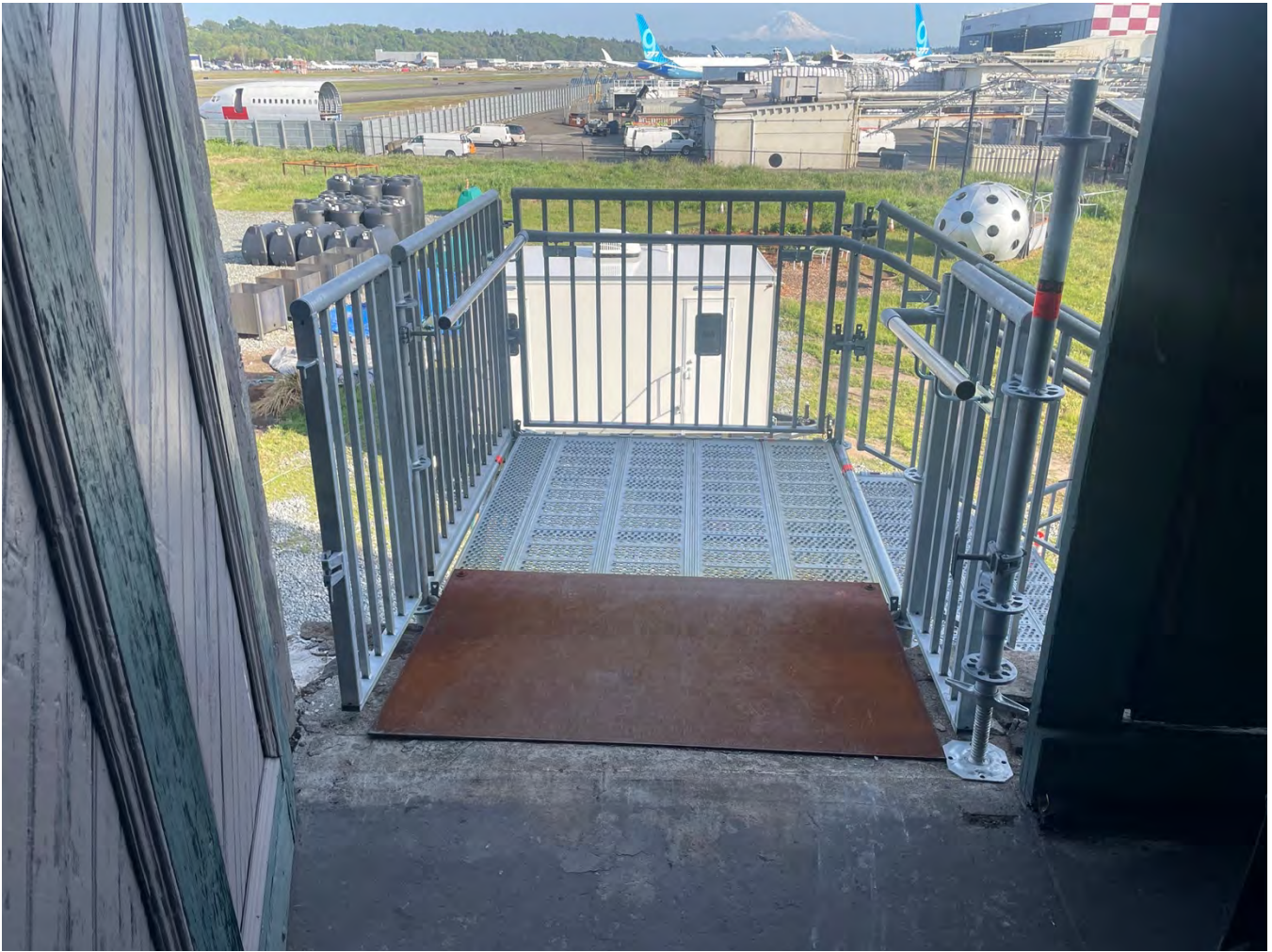
S Boiler Room Egress Scaffold Stair from inside Boiler Room
