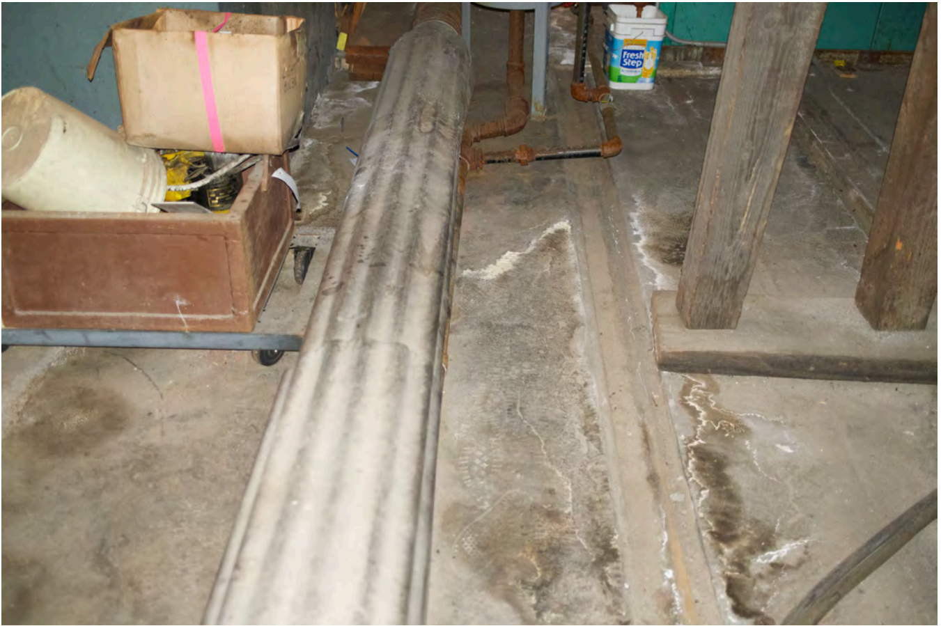
Oil Pipe West Ash Room Prior to Raising. Note Corrugated Sheet Metal Insulation Cover
