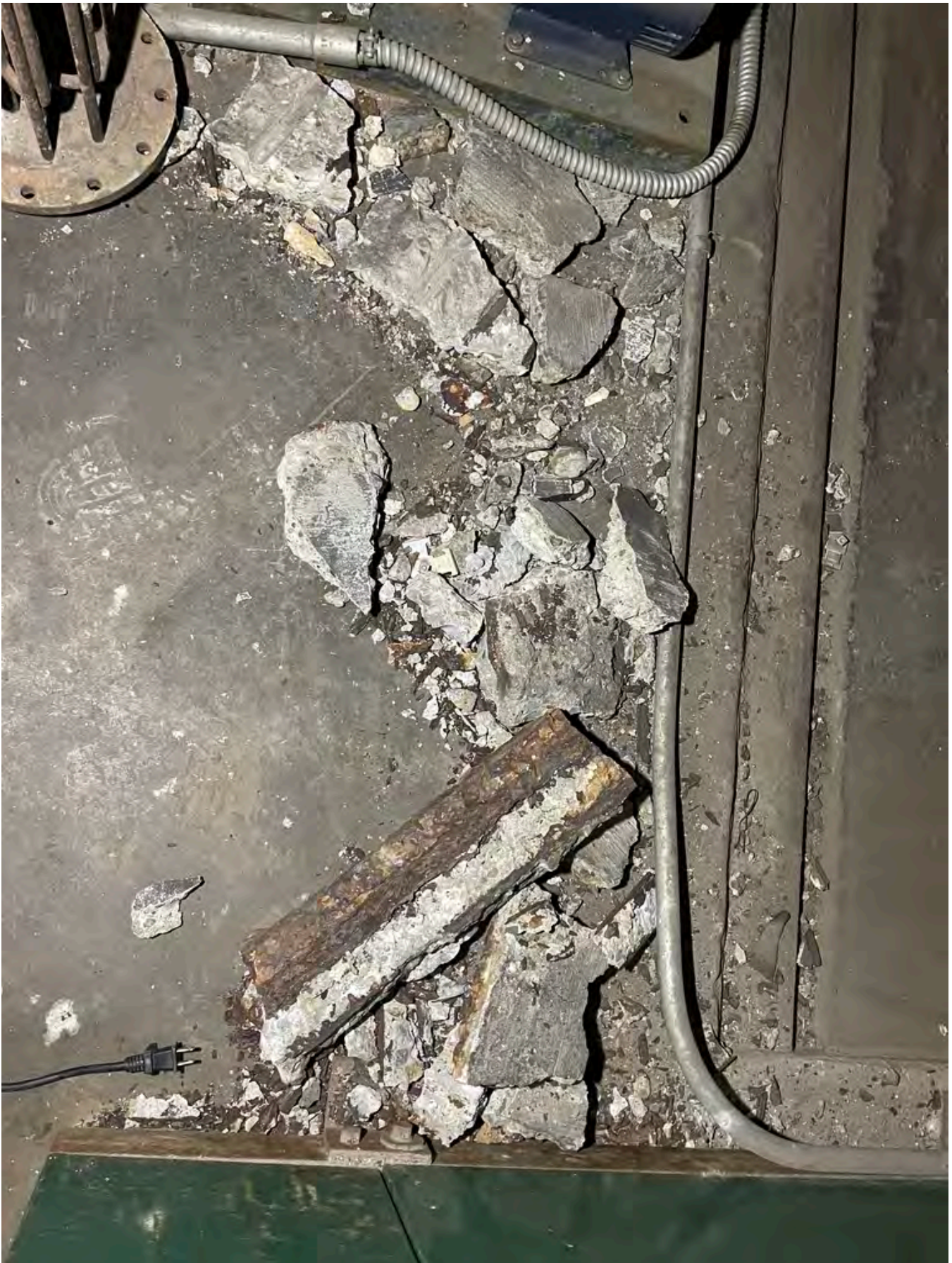
Brick and Debris Fallen From Boiler Floor and Previous Ash Hopper Removal Above. Full Bricks and Concrete Chunks Fell on a Regular Basis Prior to Loose Brick and Debris Removal Project.
