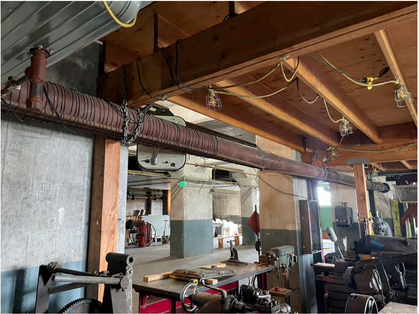
Oil Pipe Southwest Ash Room After Raising. Secured to Existing Structure with Chain.
