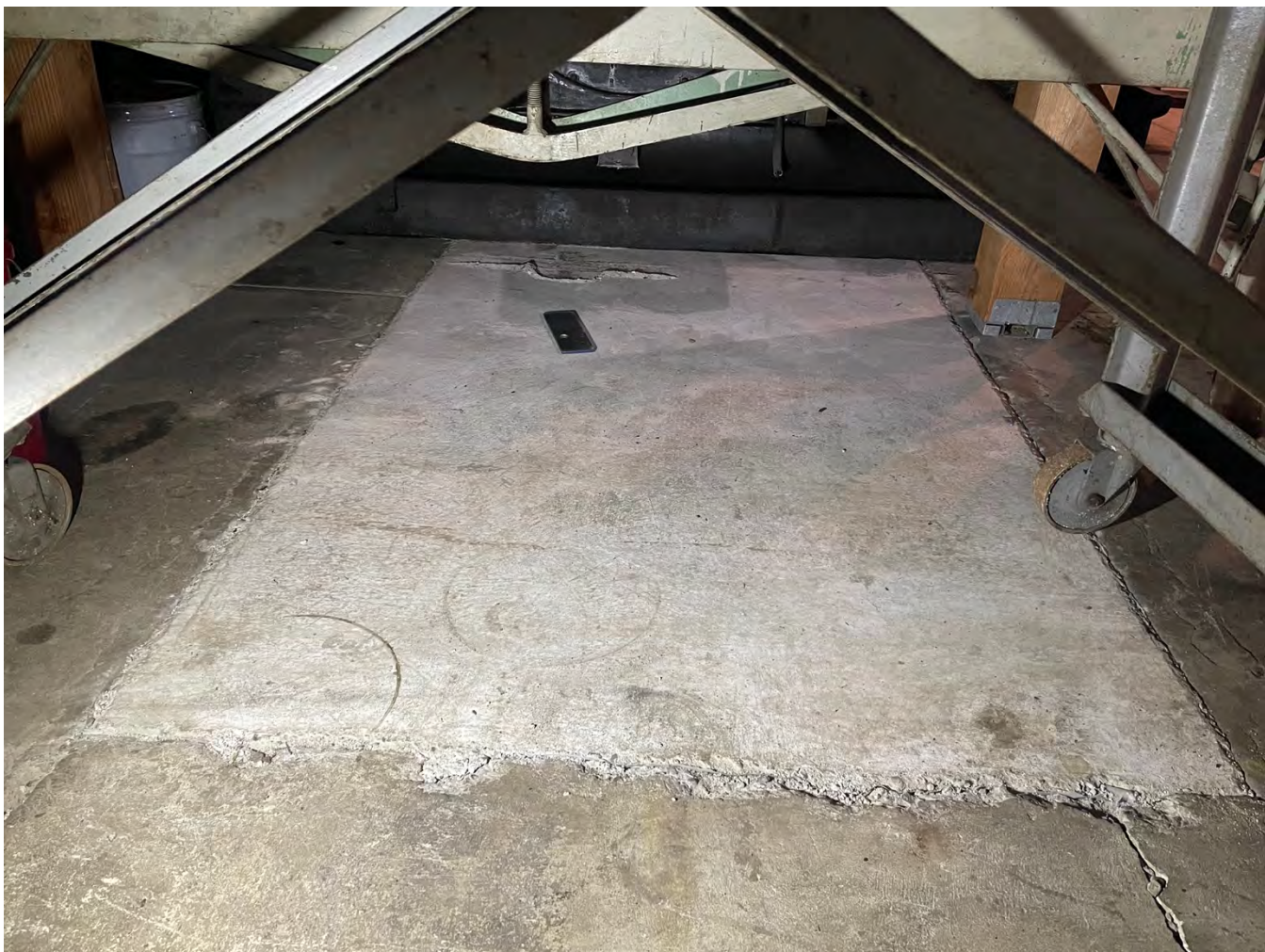
Ash Cart Track West Ash Room After Completed Concrete Infill. Note New Concrete Infill against Old Concrete Infill in Same Trackway.
