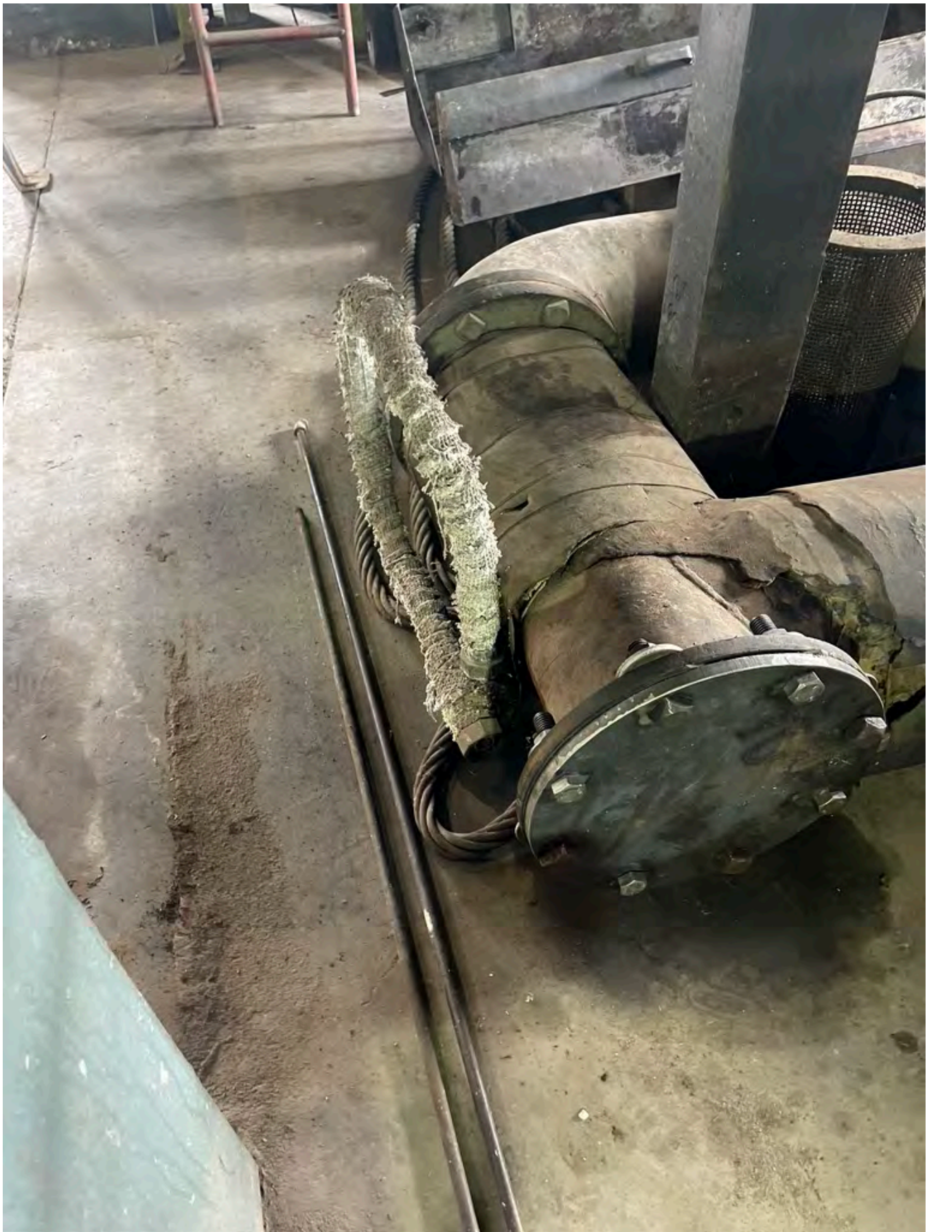
Oil Pipe South Connection After Disconnection and Raising with New Sealing Plate and Neoprene Washer
