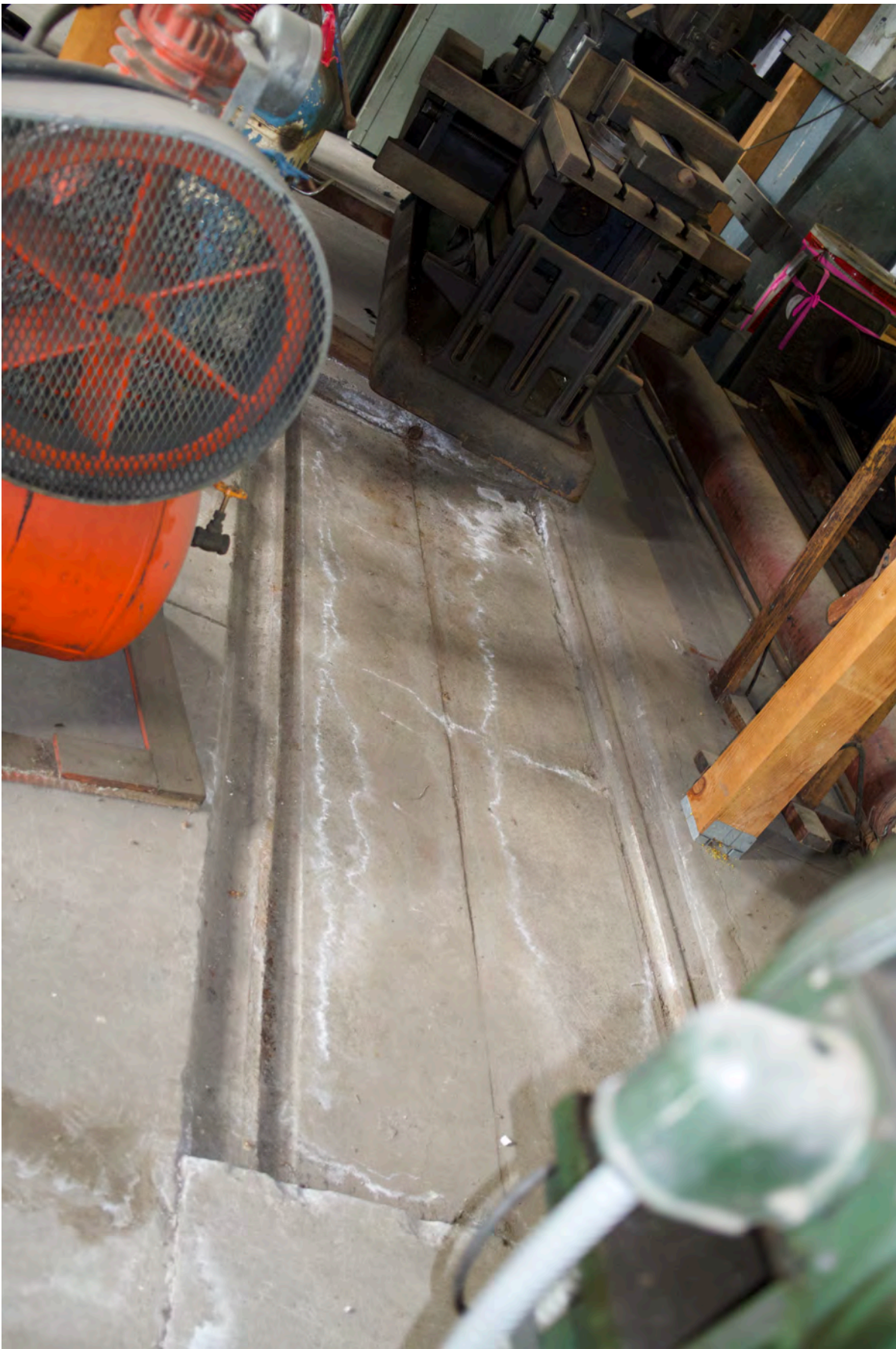
Ash Cart Track W Ash Room Prior to Concrete Infill
