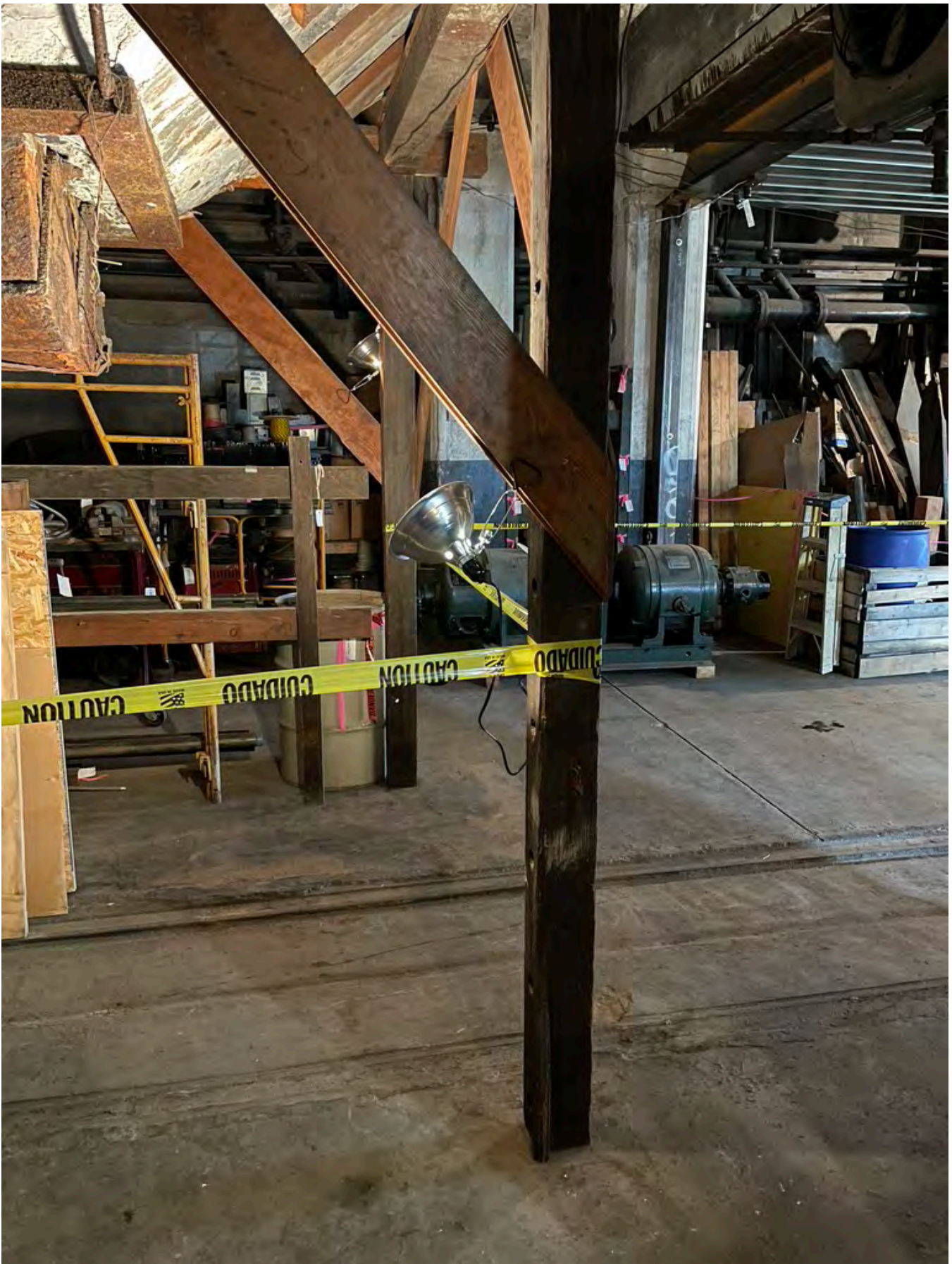
Ash Cart Track NE Ash Room Prior to Concrete Infill
