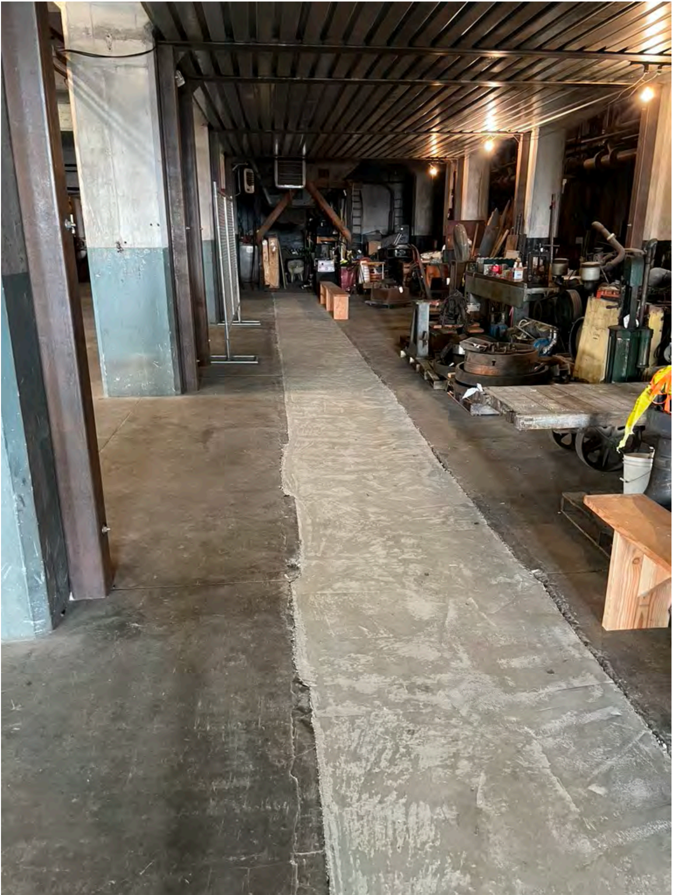
Ash Cart Track E Ash Room With Completed Concrete Infill Looking North
