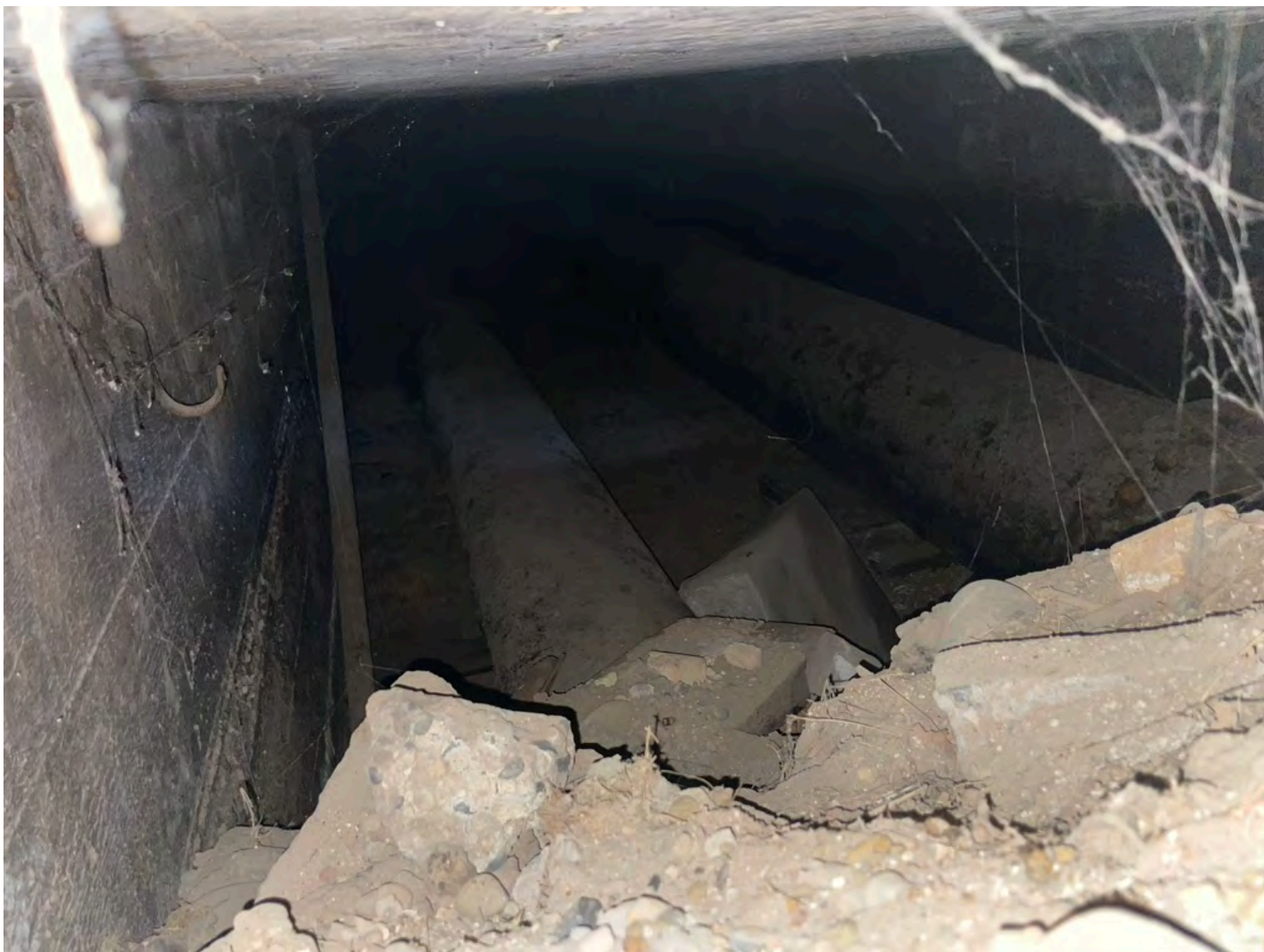
Water Intake Pipe Trench Running N/S Under Ash Room. View from top of Debris Pile facing Down and North
