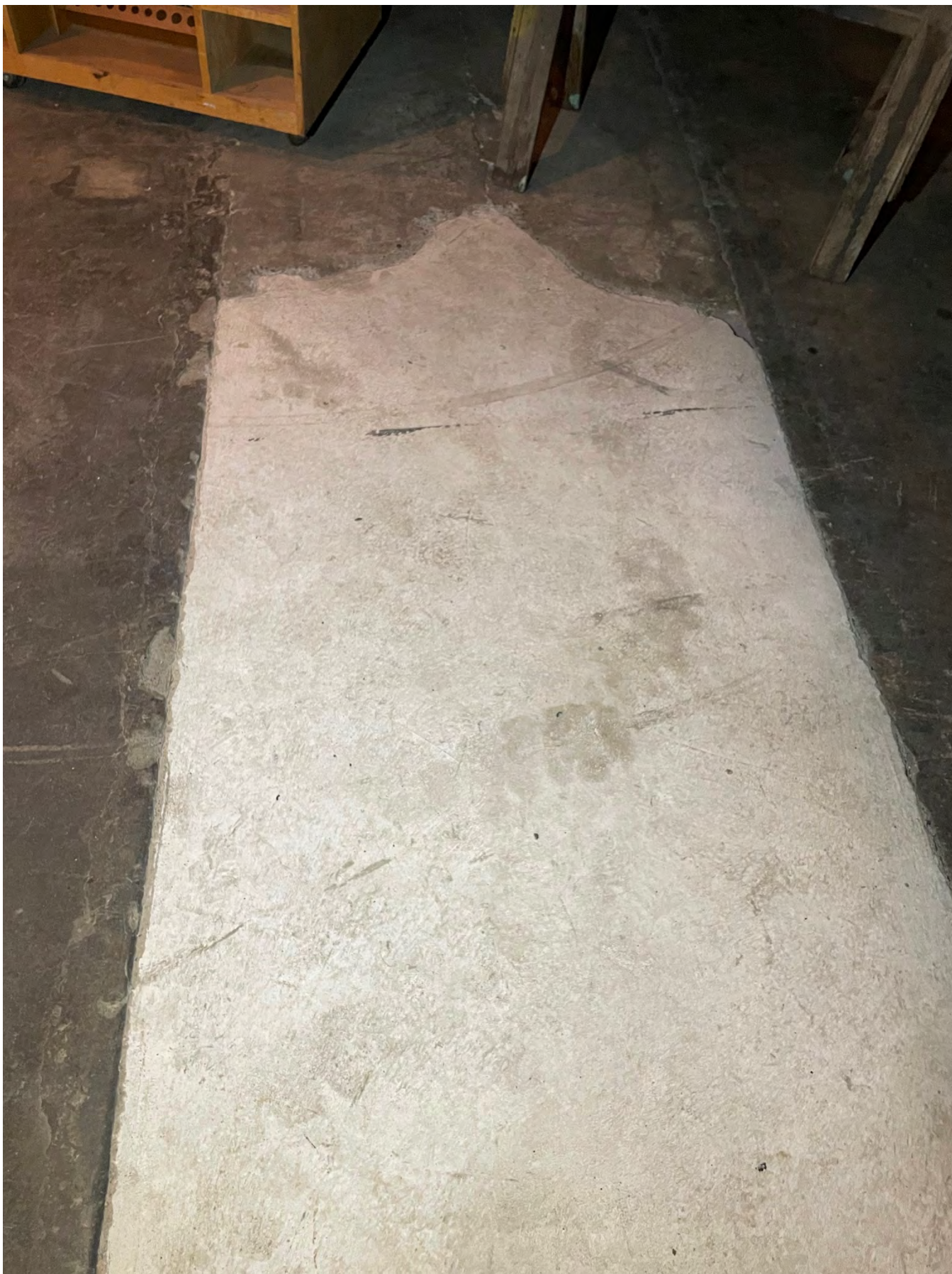
Ash Cart Track NW Ash Room After Completed Concrete Infill. Note New Concrete Infill Against Old Concrete Infill in Same Trackway.
