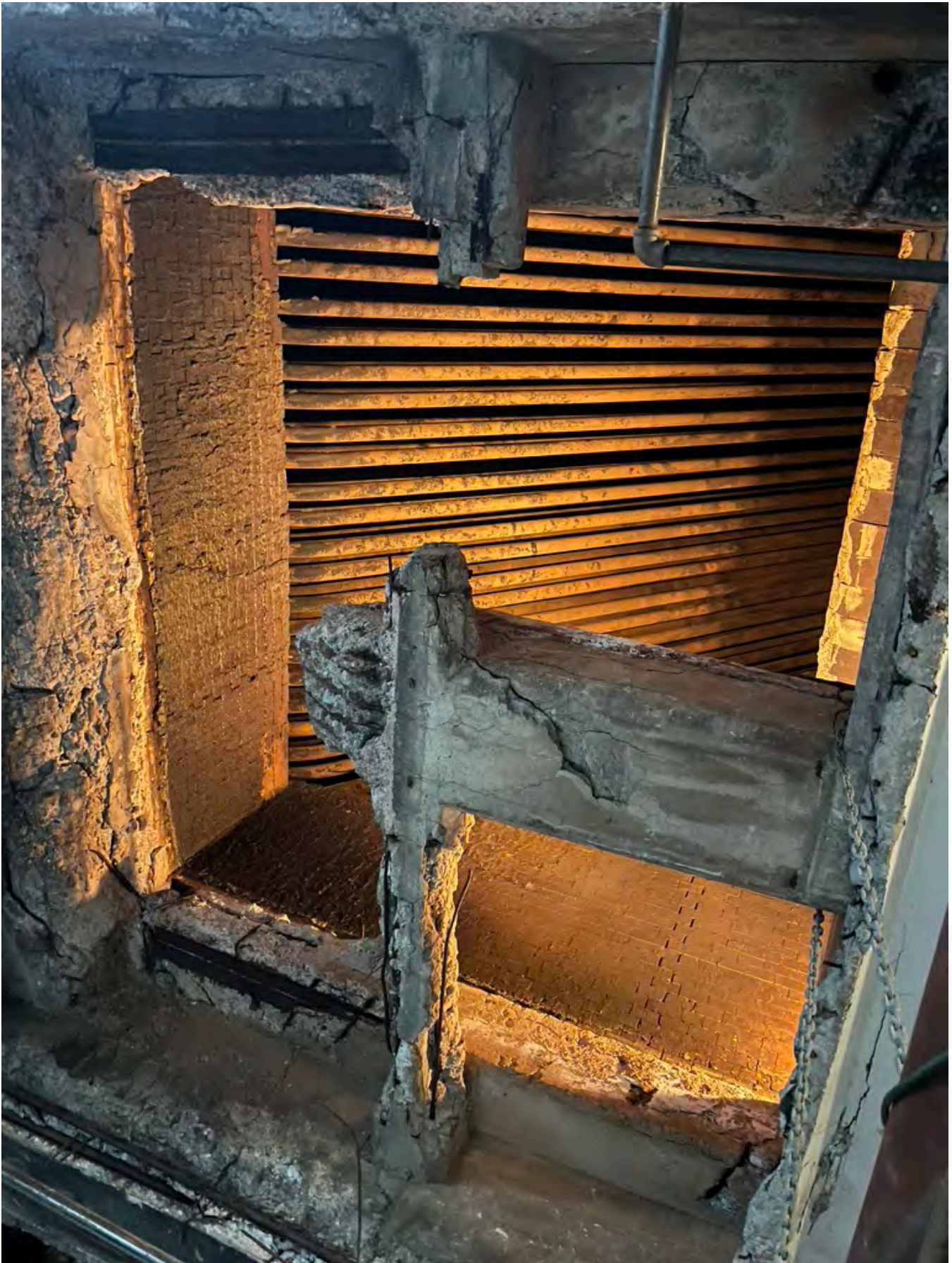
Boiler Floor/Ash Hopper After Loose Brick and Debris Removal
