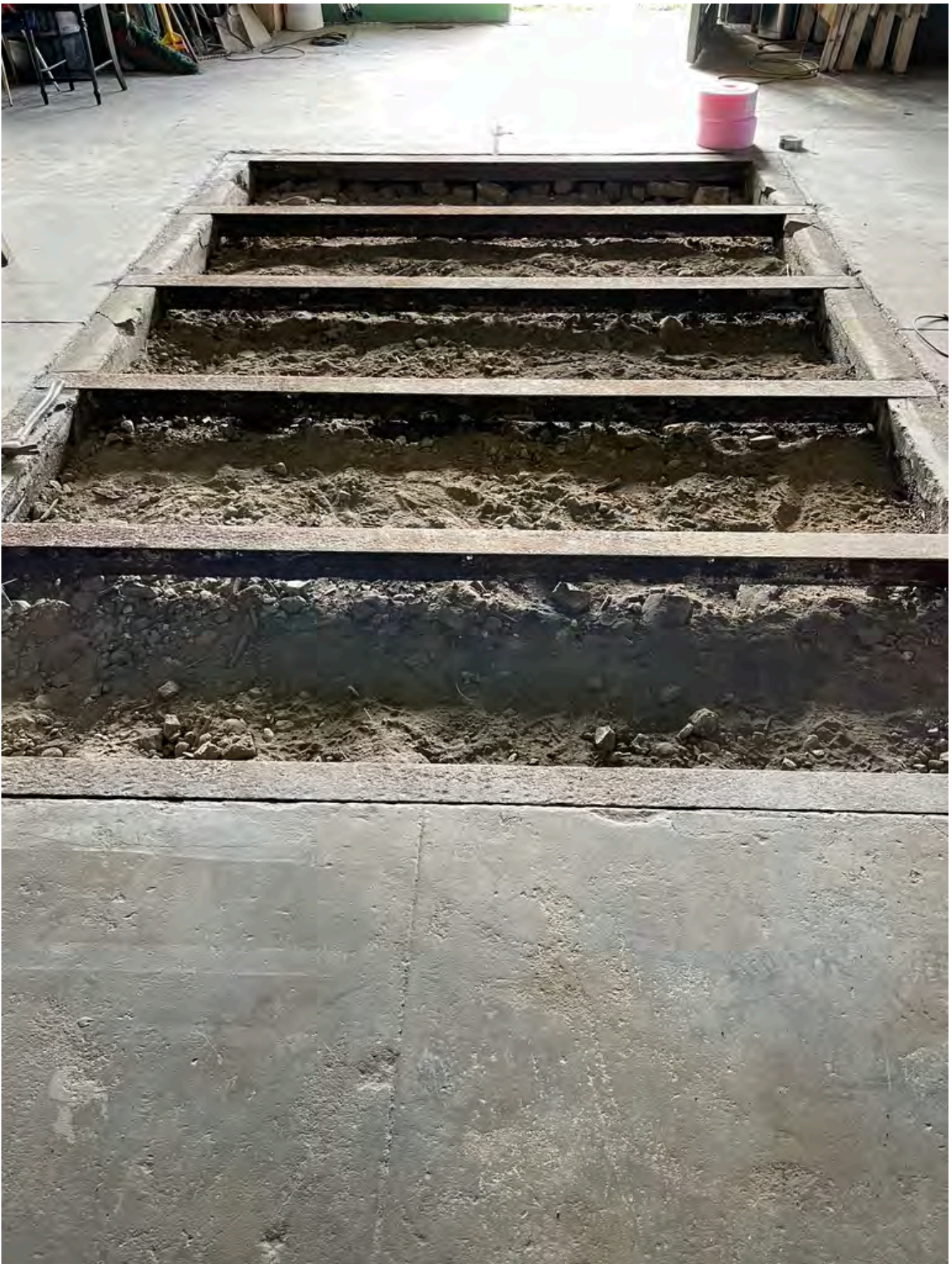
Debris Pile After Stabilization. Debris Transferred from Center to Edge of Pile and Compacted For Stabilization. See Far Edge With Built up Heavier Debris.
