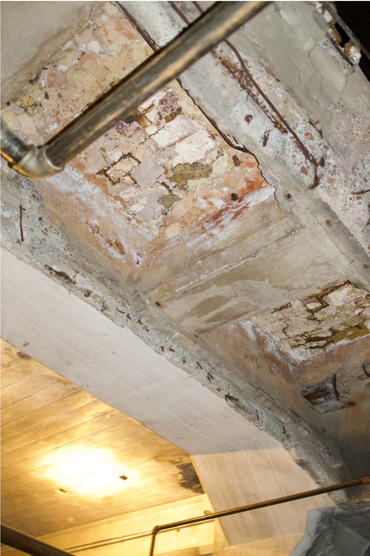
Boiler Floor/Ash Hopper Existing Condition With Loose Brick and Concrete from Previous Hopper Removal
