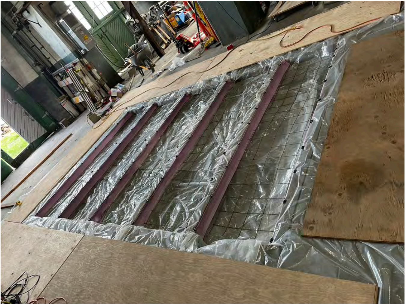
6 Mil Plastic Sheetting Over Gravel Base to Separate For Future Removal and Protect Existing Structure. Foam Infill at Tracks to Maintain Separation And Protect Existing Structure. Steel Wire Concrete Reinforcement Mesh for Imbedded Structure. Final Prep for Concrete Pour with Plywood Over Plastic Surrounding Pour Area to Protect Existing Building During Pour and Finishing.
