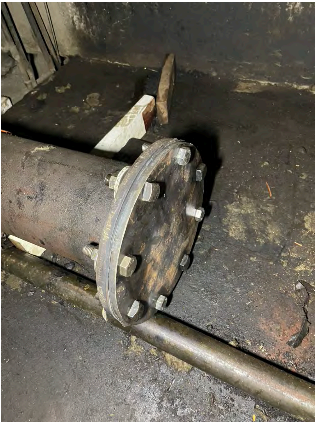
Oil Pipe Northwest Ash Room Remaining Lower Section Disconnected and Sealed with Sealing Plate and Neoprene Washer.
