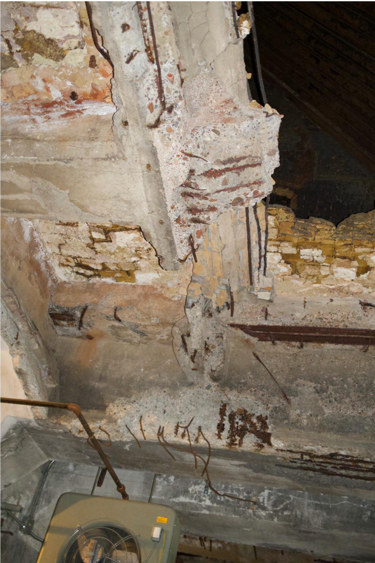
Boiler Floor/Ash Hopper Existing Condition With Loose Brick from Previous Hopper Removal
