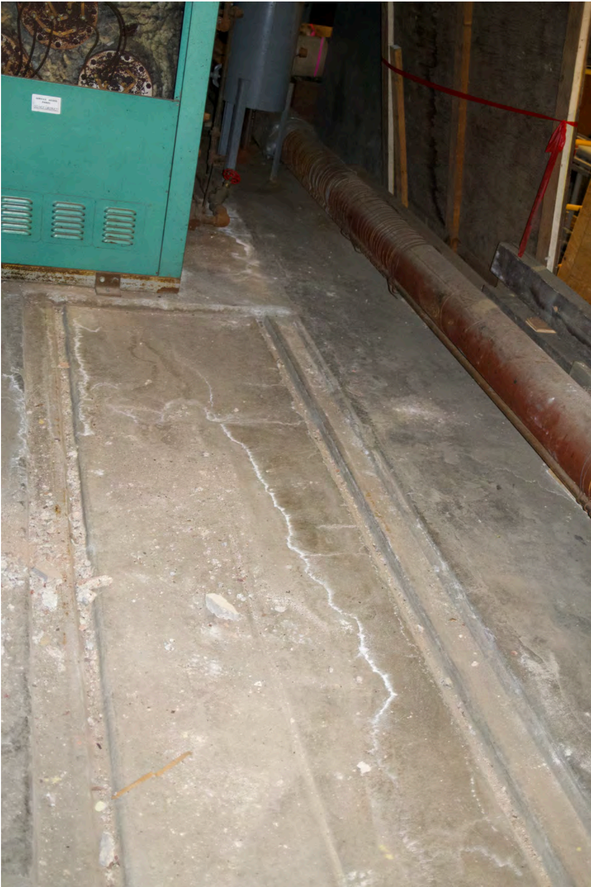
Ash Cart Track NW Ash Room North End prior To Concrete Infill
