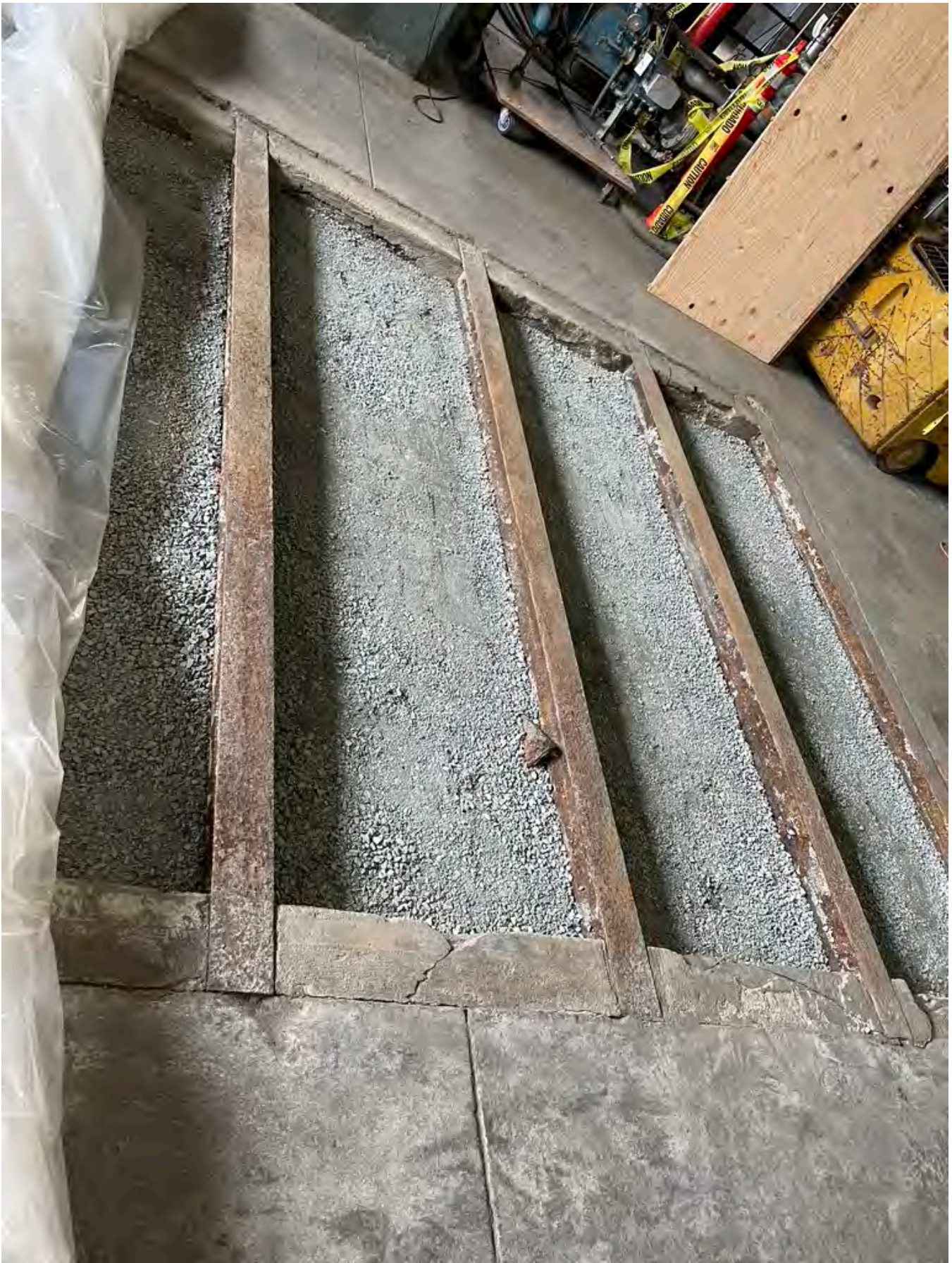
Debris Pile With Approximately 4" Deep 5/8"Minus Crushed Rock. Leveled and Compacted Approximately 4" Below Finished Surface
