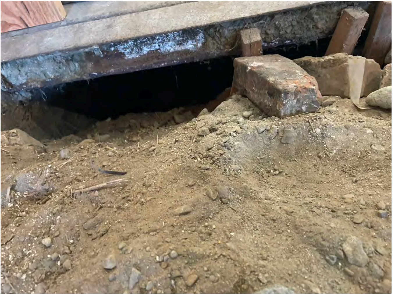
Debris Pile Edge in Trench Prior to Stabilization
