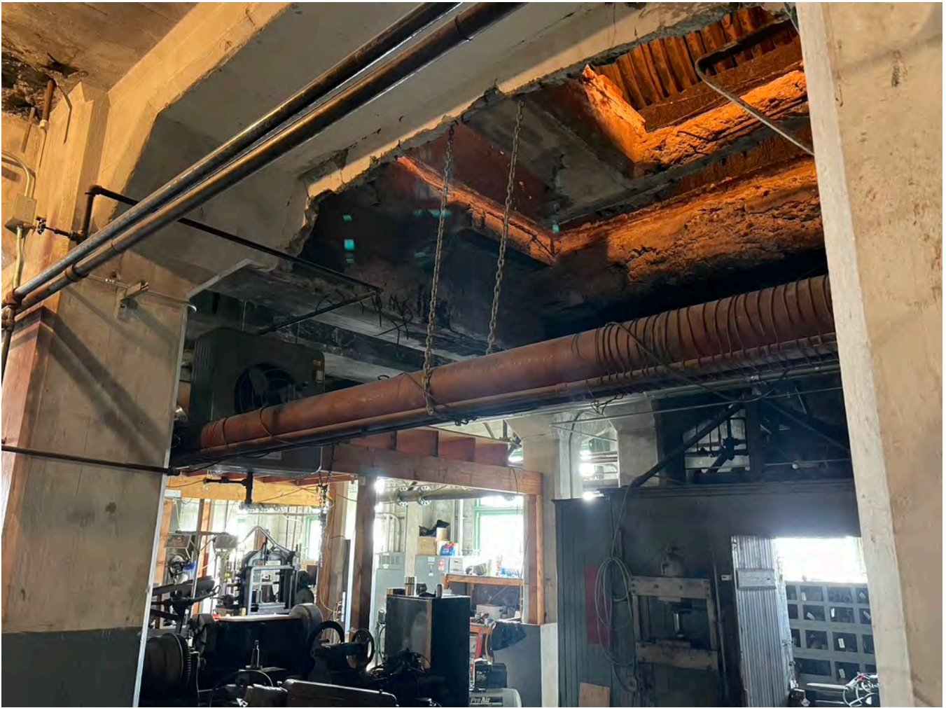
Oil Pipe West Ash Room After Raising. Secured to Existing Structure with Chain.
