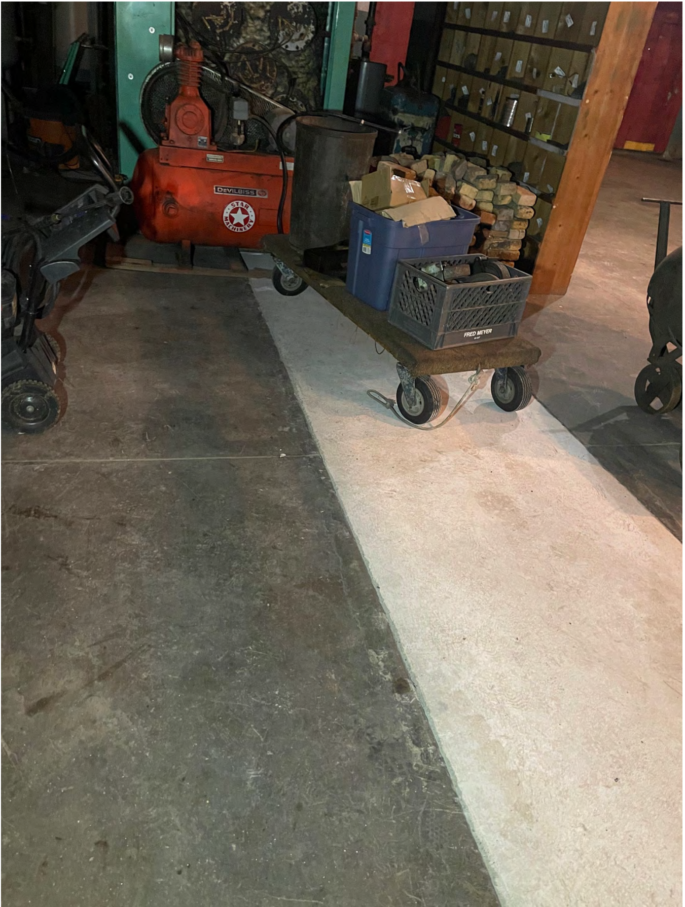
Ash Cart Track NW Ash Room After Completion of Concrete Infill
