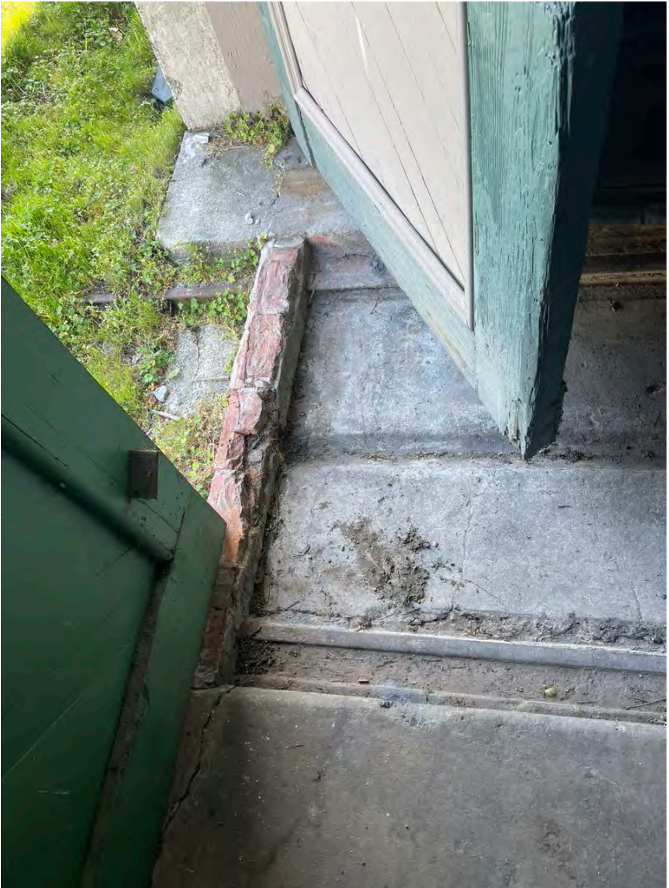
Ash Cart Track SE Ash Room Prior to Concrete Infill (South Extent of Infill at South Door)
