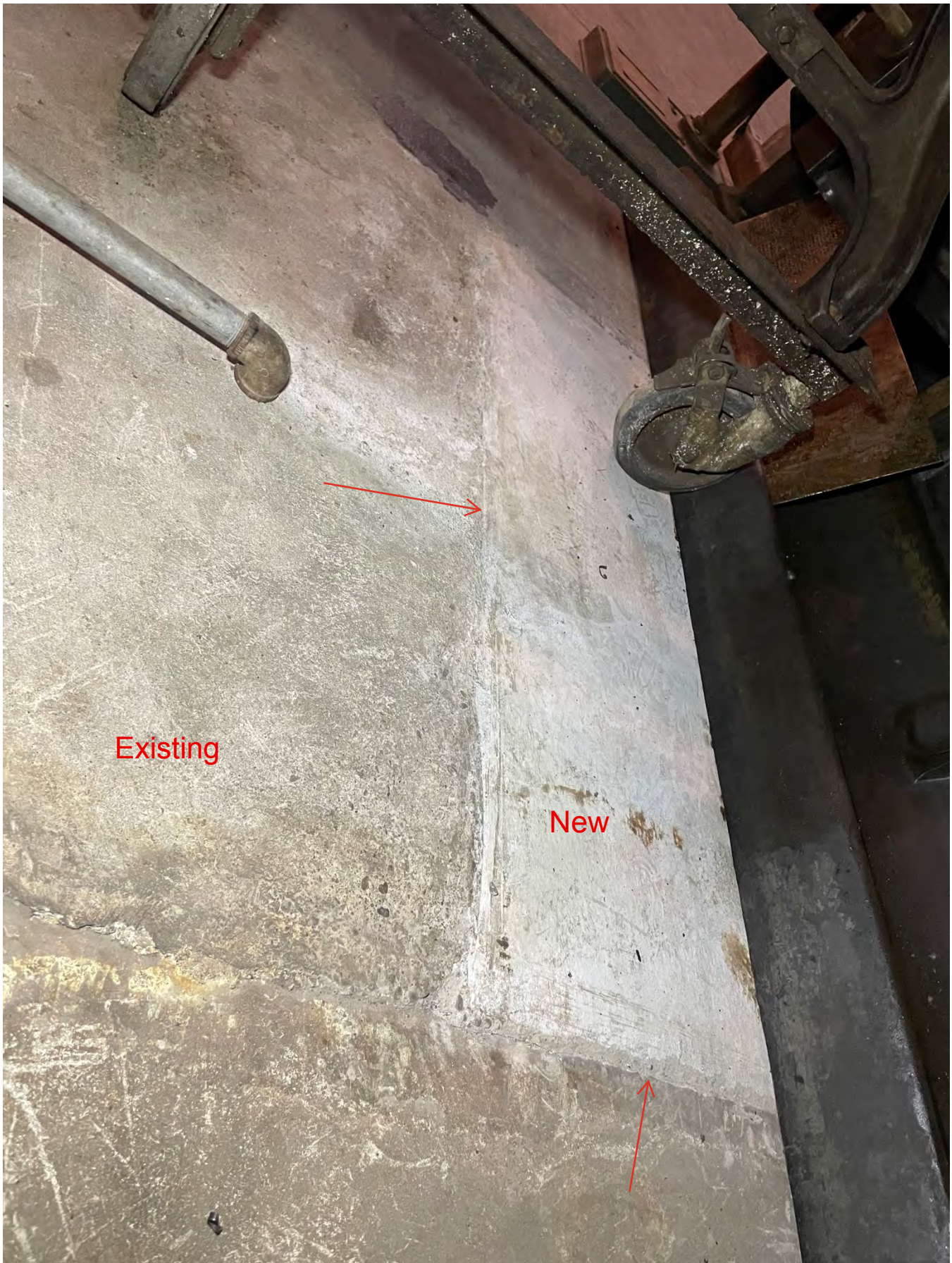
Ash Cart Track West Ash Room After Concrete Infill Completed. Note New Concrete Infill Against Old Concrete Infill in Same Trackway.
