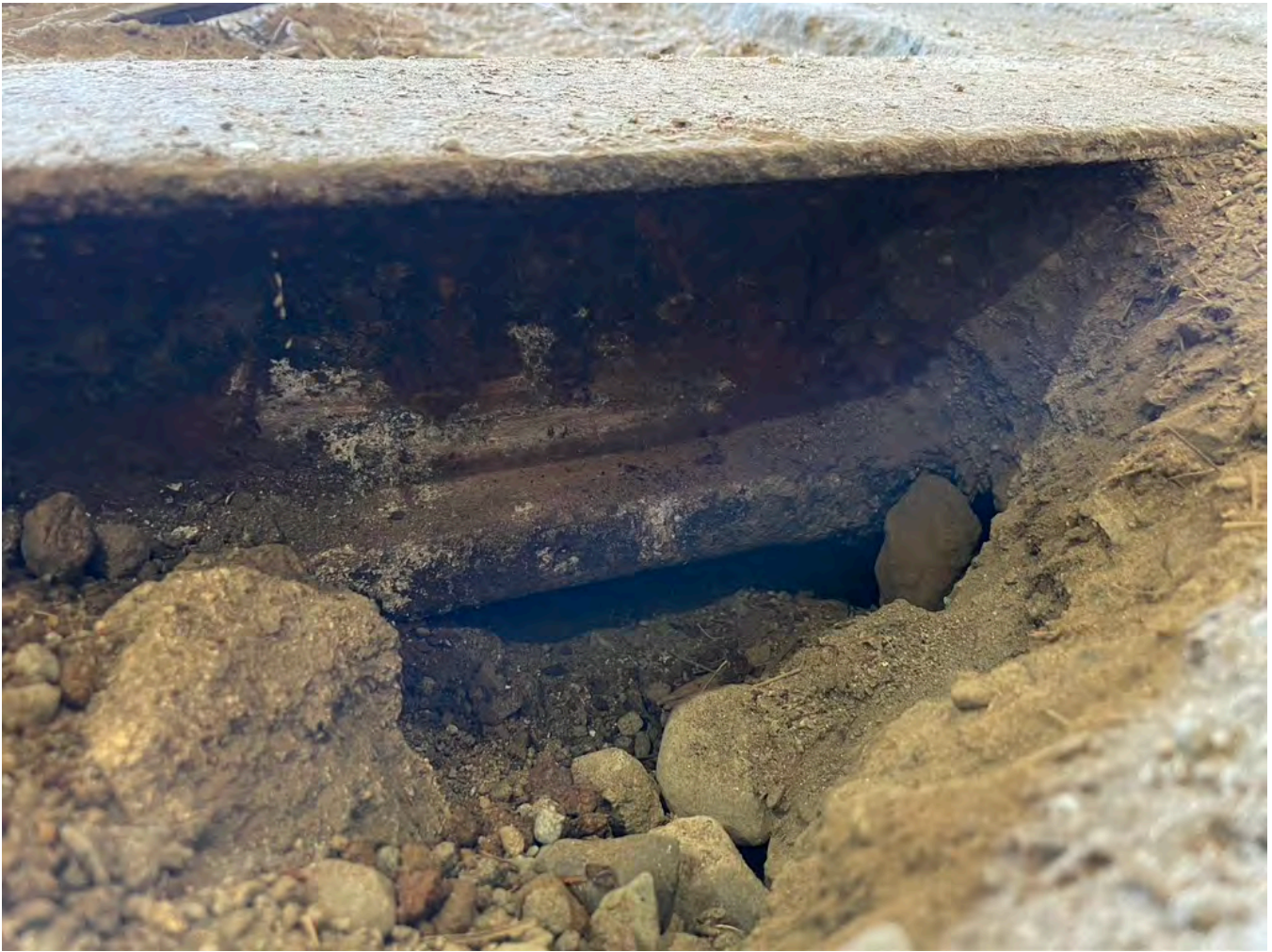
Detail of upside Down Railroad Track Structure at Surface of Opening. Previously Used to Support Steel Plates to Cover Trench
