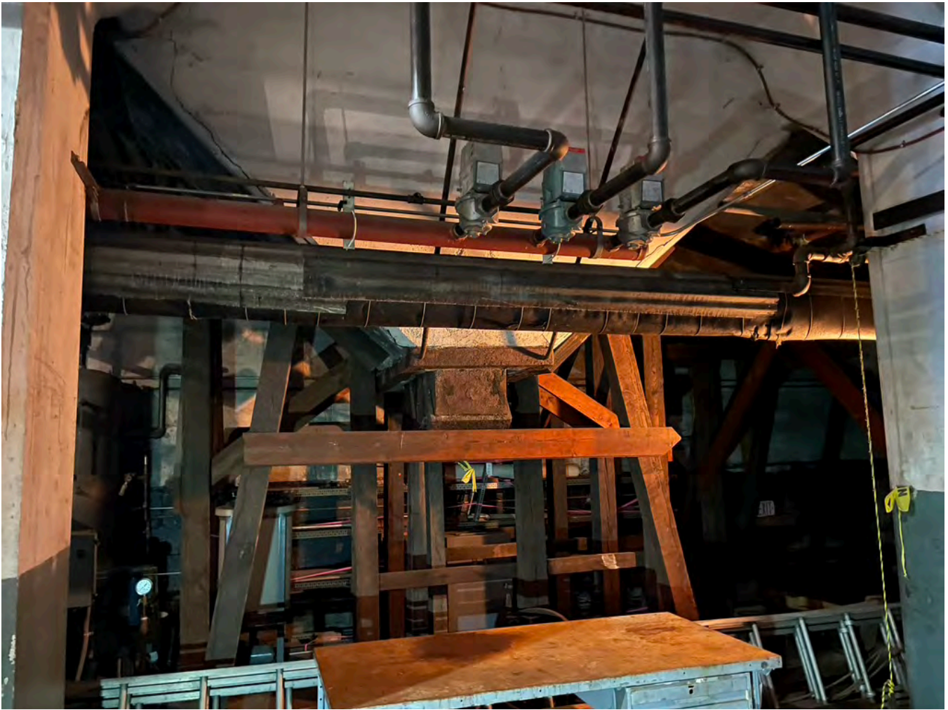
Oil Pipe Northwest Ash Room After Raising. Secured to Existing Structure with Chain.
