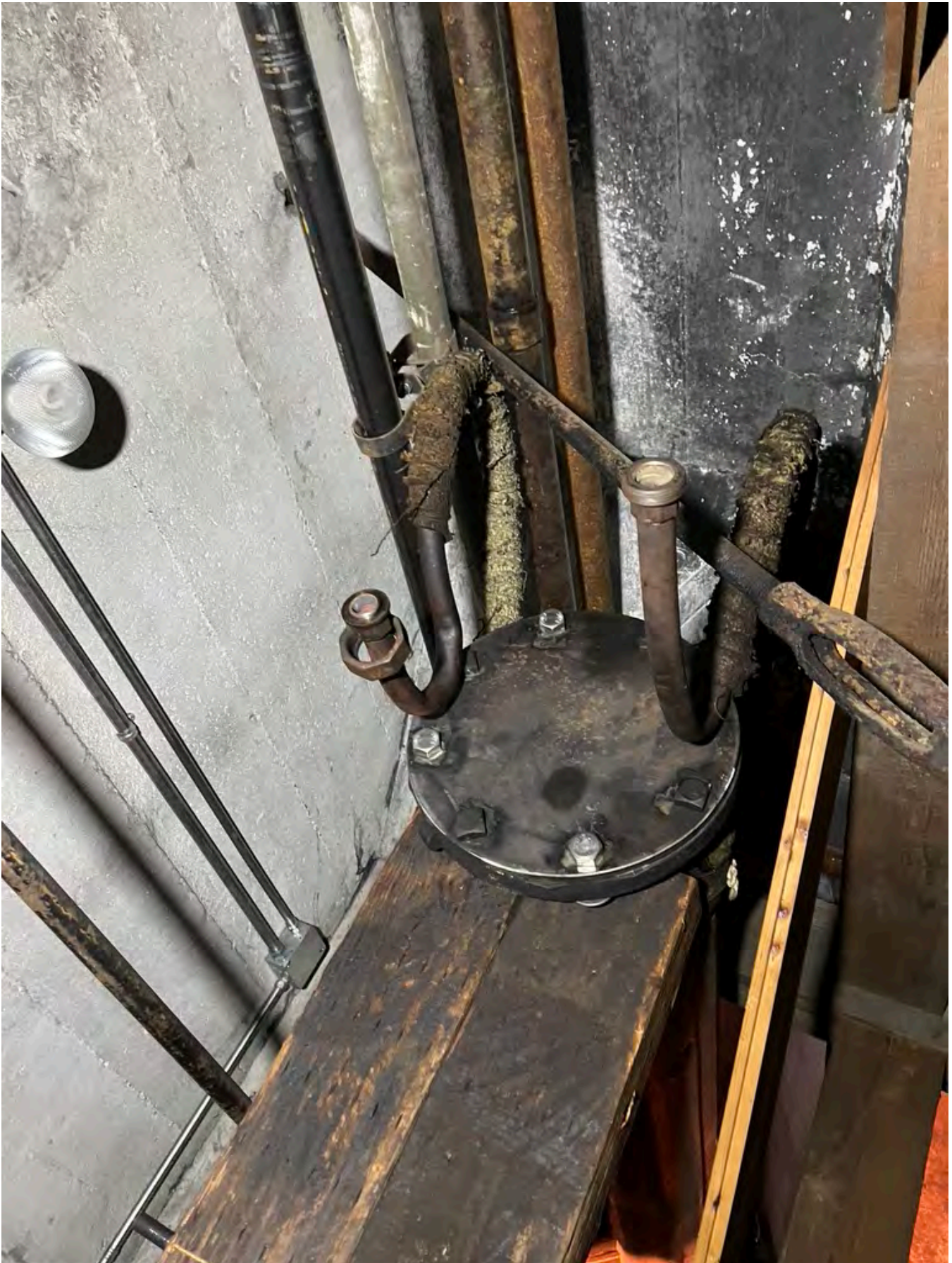
Oil Pipe Northwest Ash Room After Raising. Secured to Existing Structure with Chain and Braced on Solid Wood Post. North Extent with Sealing Plate and Neoprene Washer. Note Steam Heat Loop Pipes Disconnected at Unions.
