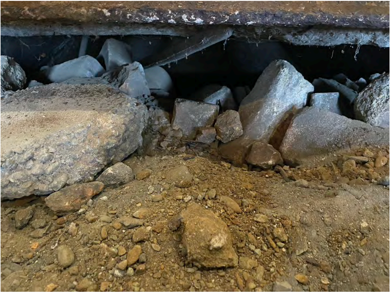
Debris Pile After Stabilization with Heavier Debris Edge Build Up for Structure
