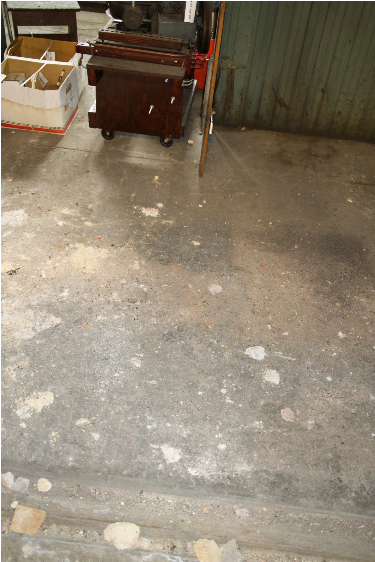
Brick and Debris Fallen From Boiler Floor and Previous Ash Hopper Removal Above. Full Bricks and Concrete Chunks Fell on a Regular Basis Prior to Loose Brick and Debris Removal Project.
