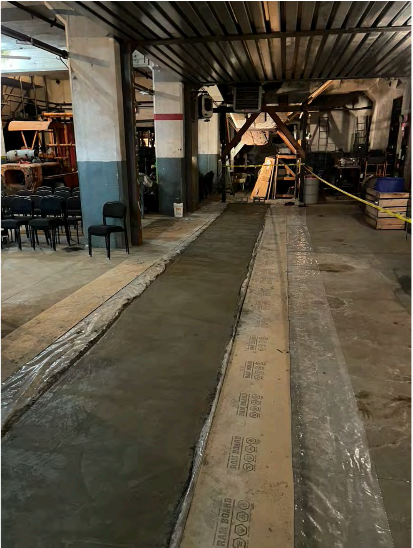
Ash Cart Track East Ash Room Looking North During Concrete Pour and Finishing
