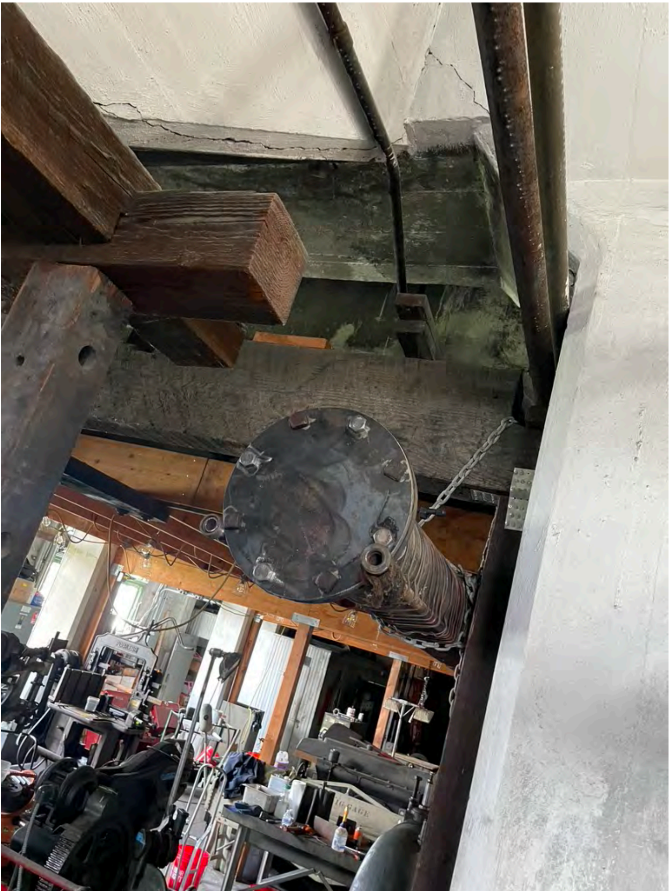
Oil Pipe West Ash Room After Raising. South Extent with Sealing Plate and Neoprene Washer. Note Steam Heat Lines Disconnected at Unions. Pipe Secured with Chain to Existing Structure.
