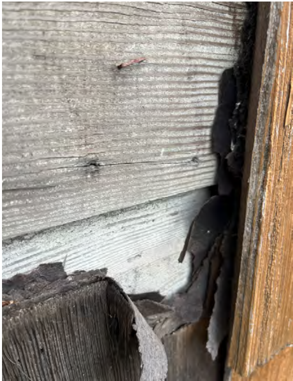
EXISTING HORIZONTAL SIDING UNDER 1980-ERA SHINGLES
