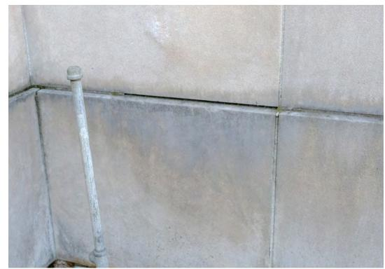
Areas of mortar loss and surface dirt
