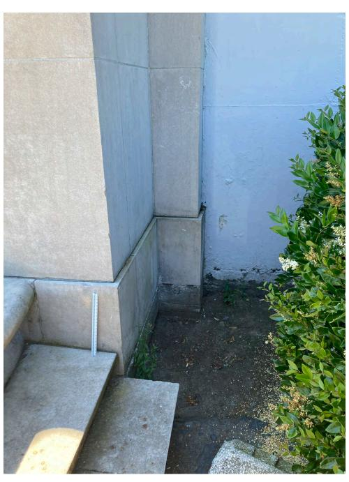
North Memorial Stone Wall and Stadium Concrete Wall at Grade - Chiping at Exposed Slab and Corner
