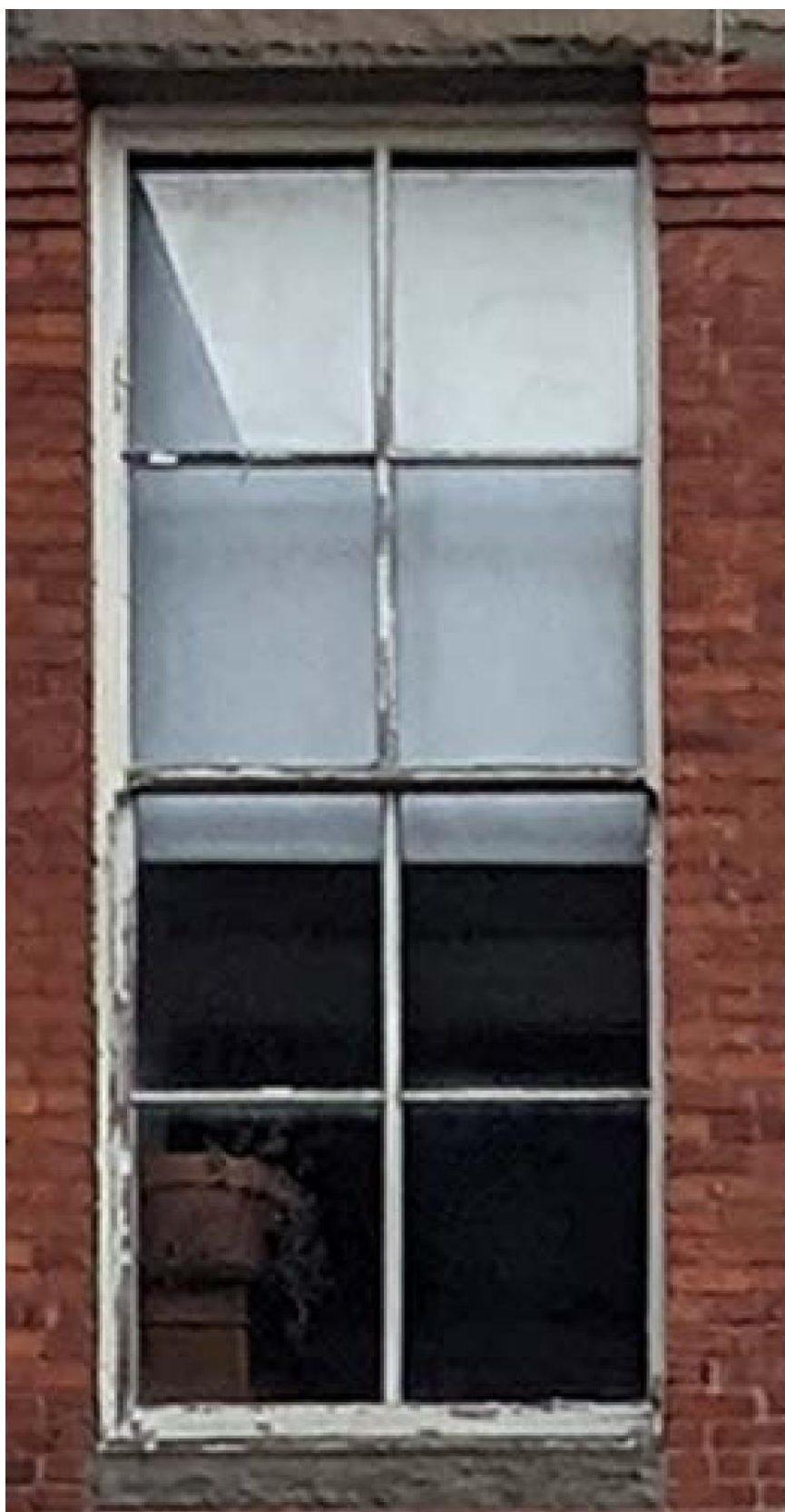
1 Existing 1892 Double Hung Window NTS
