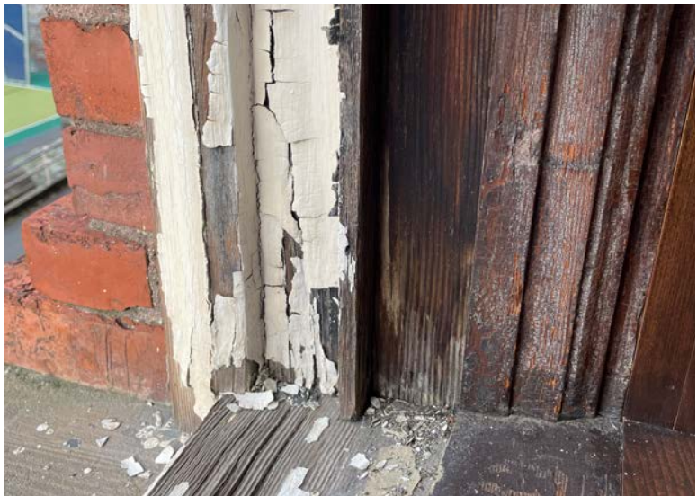
Exterior paint failure resulting in weathered bare wood at frame and sill
