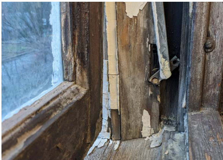
1916 tilt hardware in very bad condition
