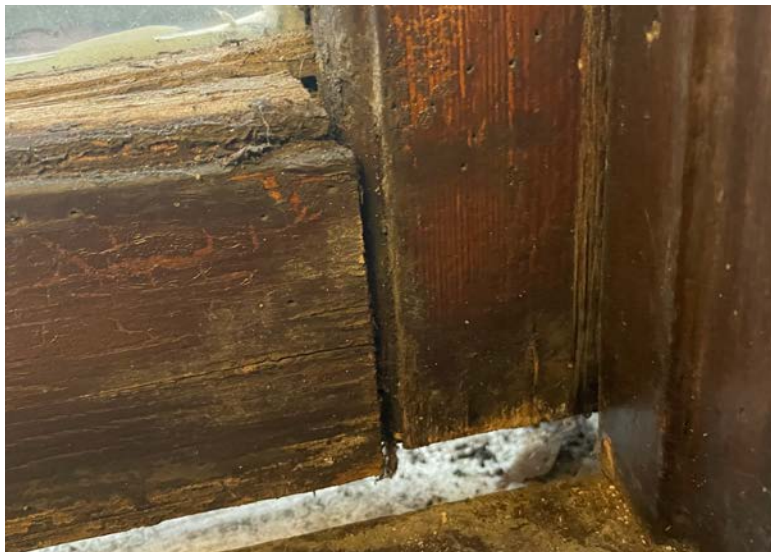
Separation between stile and bottom rail
