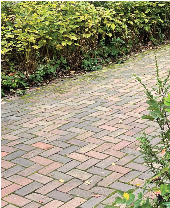
Non-historic brick pathway to be dismantled, salvaged, and re-installed. The original herringbone pattern with soldier course edge to be recreated. No new brick anticipated to be introduced as part of this rehabilitation project.
