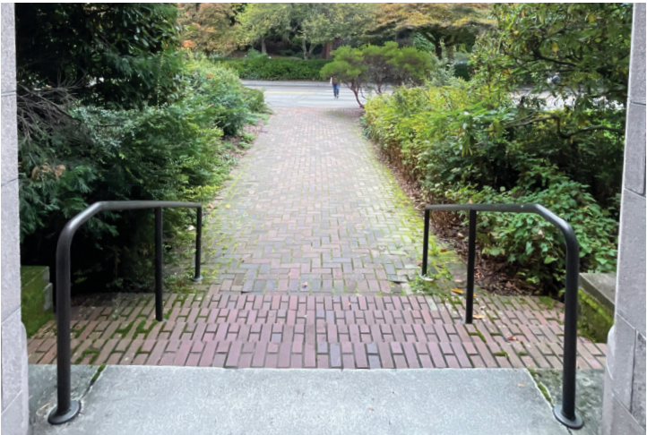
Uneven surfaces at handrail and pathway
