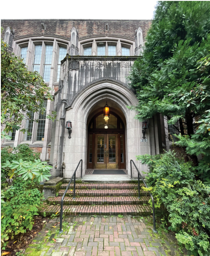
Historic north entry with brick stairs to be preserved. Non-historic railing to be removed and replaced.
