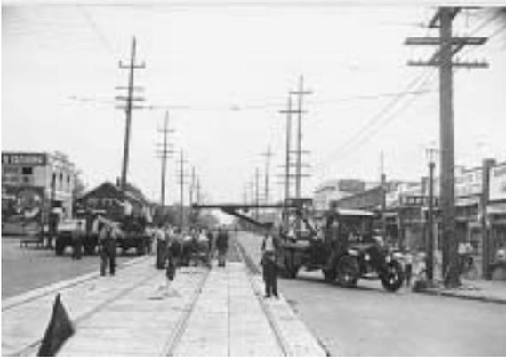
1934 pre-cast concrete slabs being set along Beacon Avenue South for the streetcar tracks. This WERA project provided work for numerous individuals in a time when work was scarce. Source: University of Washington Libraries, Special Collections, UW20653z.
