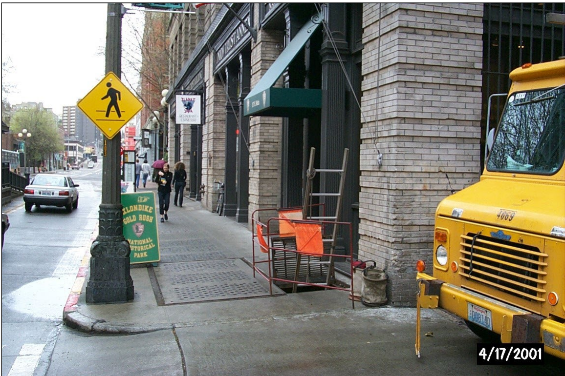
Photo 4 – A view of the same location, taken in 2001, with ladder access in use. (Source: Seattle City Light, 2001.)
