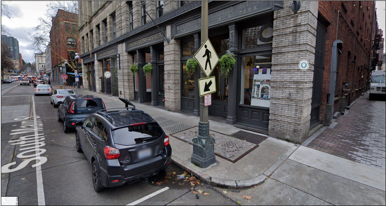
Photo 2 – View to the southeast showing Vault 22V-4 on the corner of South Main St. (on the left) Nord Alley (on the right), and in front of the Union Trust Annex. (Source: Google Maps, street view, 2021.)
