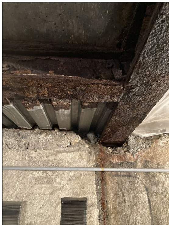
Photo 7 – Detail view showing general conditions of the steel beams and ceiling decking in the vault. (Source: SCL, 2022.)
