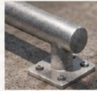
METAL FINISH Galvanized Finish Steel structure + hardware
