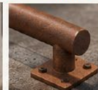
METAL FINISH Stabilized Rust Steel structure + hardware
