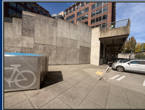
Figure 2.2 showing current locker in relation to the ADA ramp
