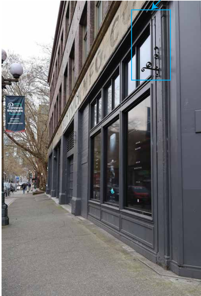
South Washington Street (Looking East)
