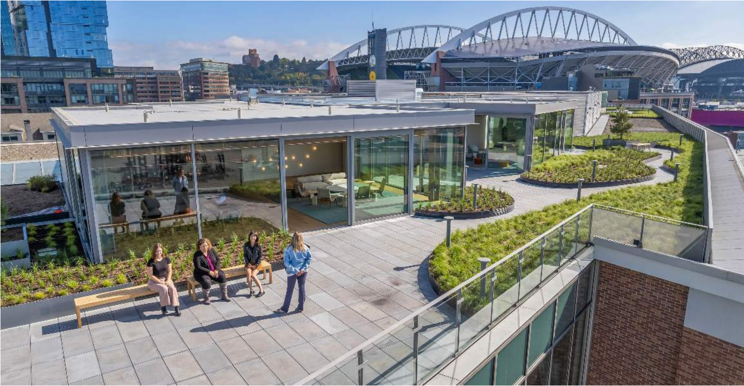
EXISTING CONDITIONS AT ROOF DECK LEVEL
