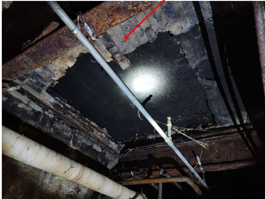
Fig 24: Ceiling near middle of areaway
