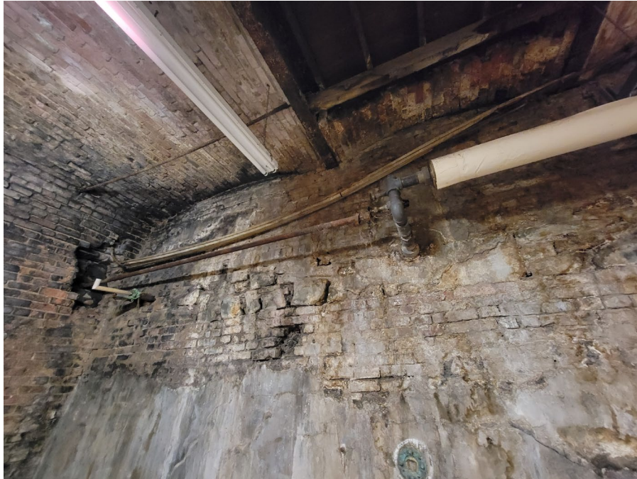
Fig 7: Near north end of areaway looking at street wall
