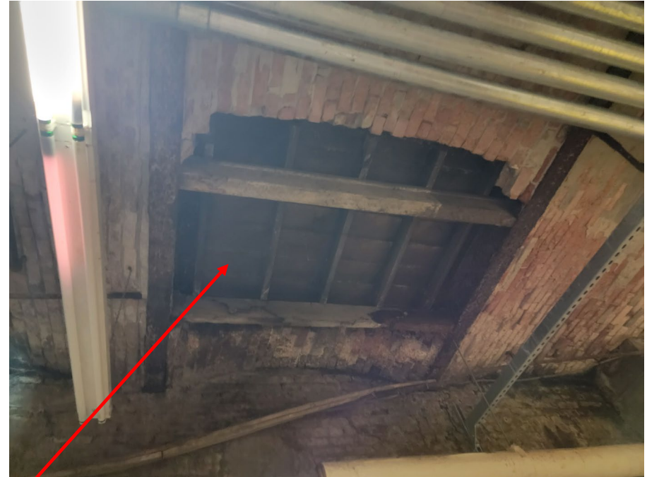
Fig 8: Looking at ceiling near north end
