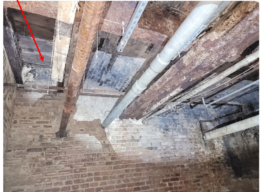
Fig 25: Ceiling near north end of areaway
