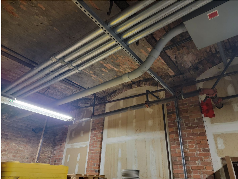
Fig 11: Openings building face from inside of areaway at south end
