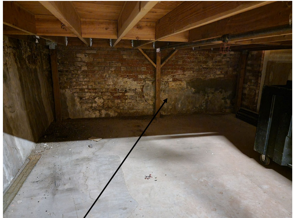
Fig 6: South end of areaway
