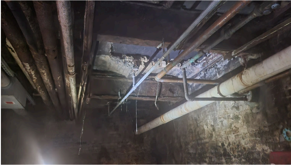
Fig 22: Northeast corner of areaway
