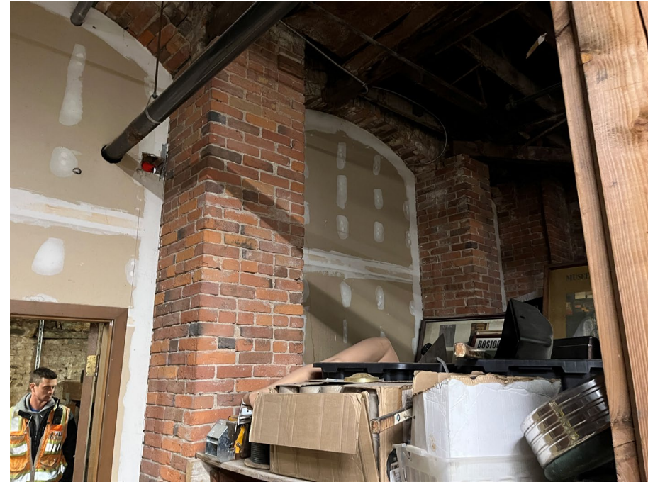
Fig 12: Openings looking towards areaway from building at south end
