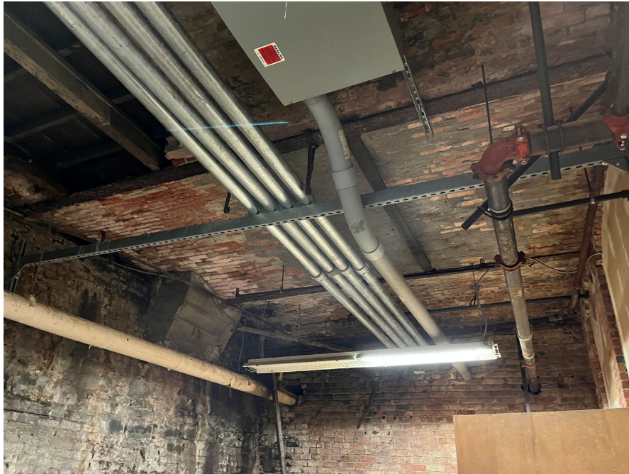
Fig 9: Barrel arch ceiling near south end
