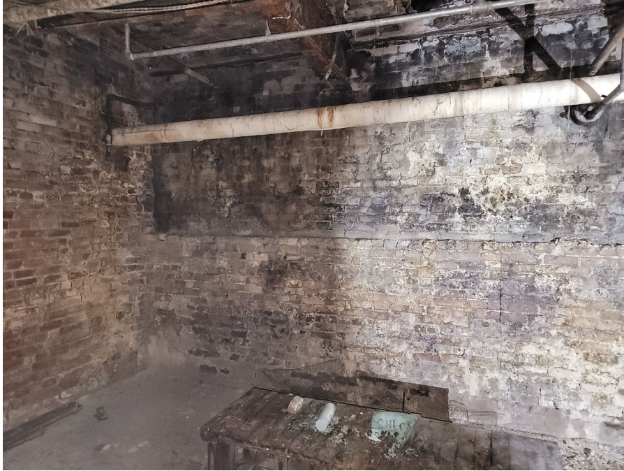
Fig 16: Near north end of areaway looking at street wall
