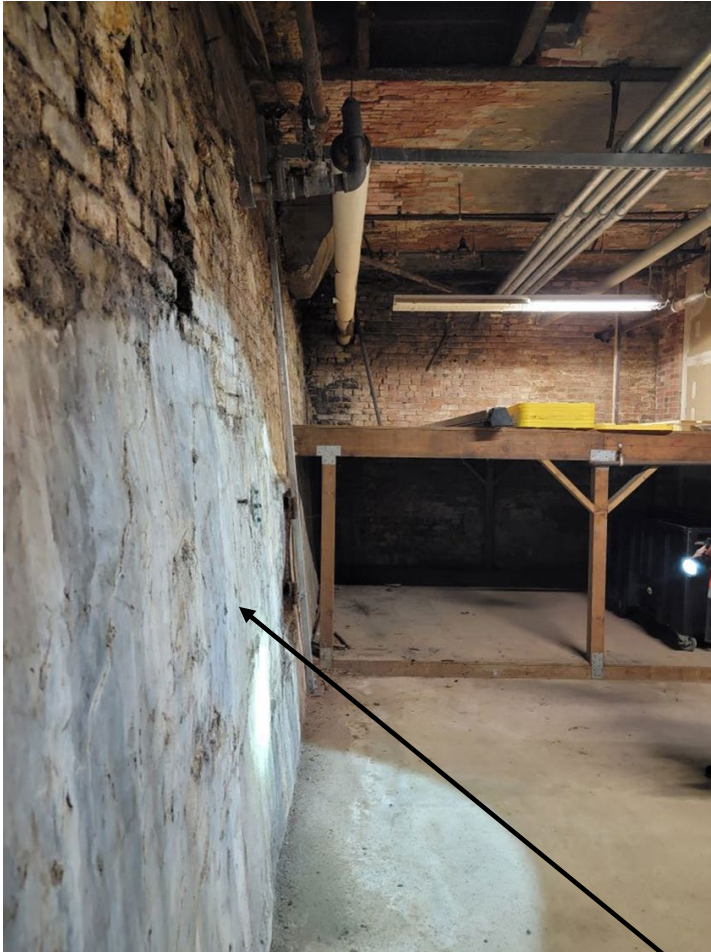
Fig 5: Looking at south end of areaway
