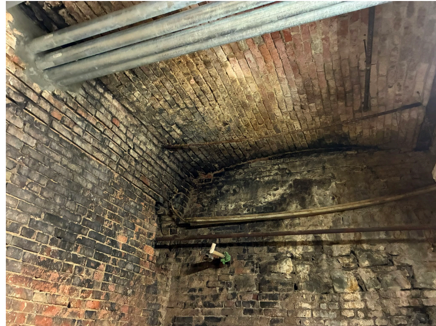
Fig 10: Barrel arch ceiling near north end
