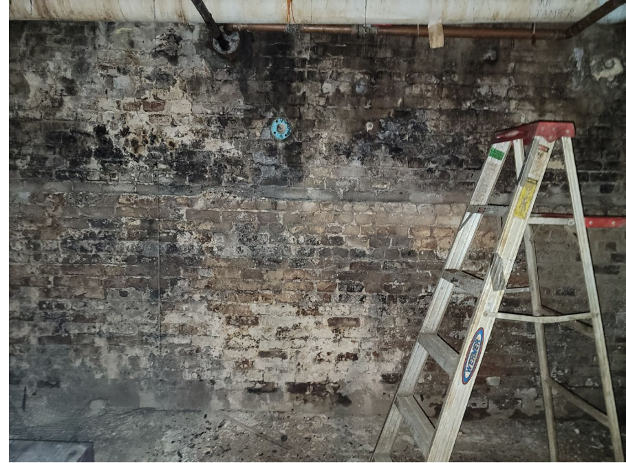
Fig 17: Looking at east at street wall near middle of areaway
