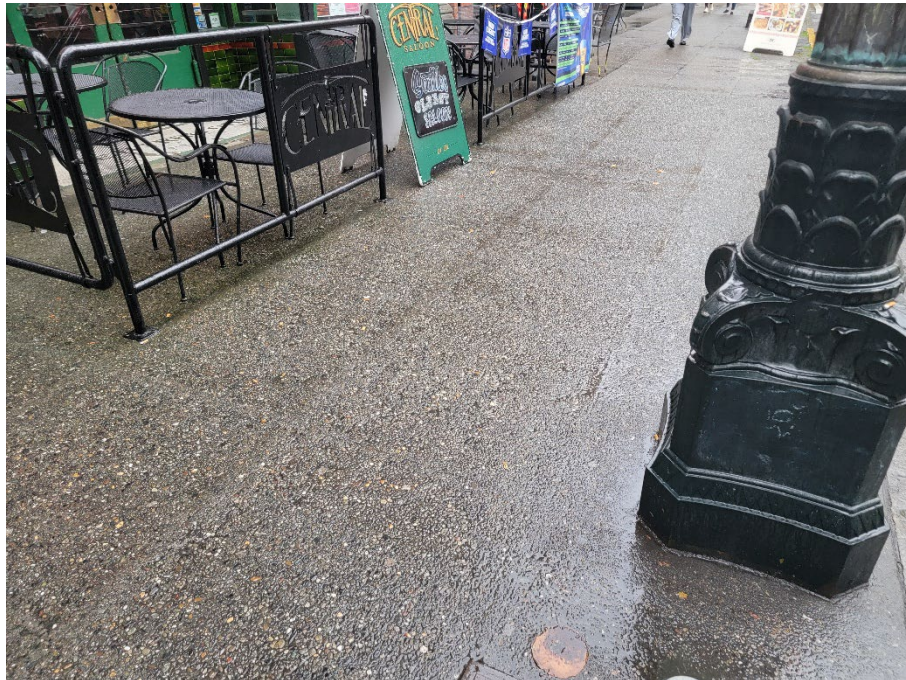
Fig1: Near south end of areaway, looking north at sidewalk
