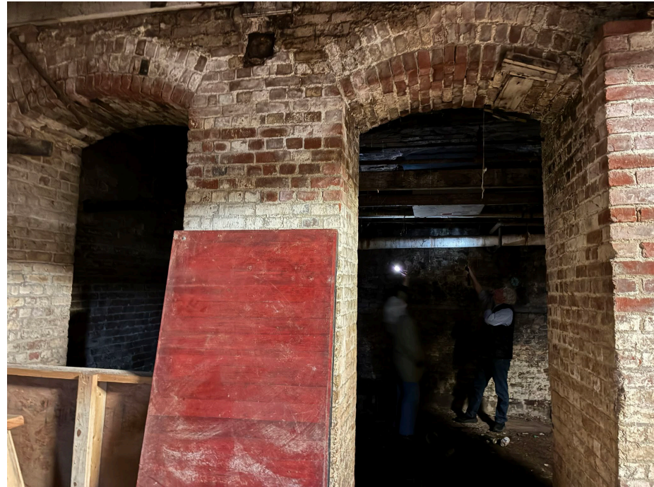
Fig 19: Looking east from building at north end of areaway
