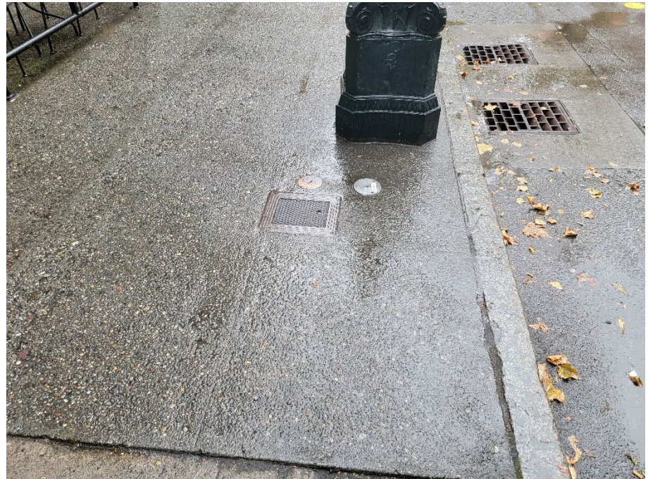
Fig 2: At south end limits of areaway, looking north at sidewalk
