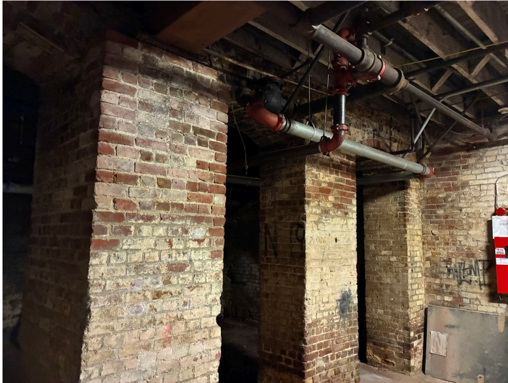
Fig 20: Looking towards the south end of areaway from building
