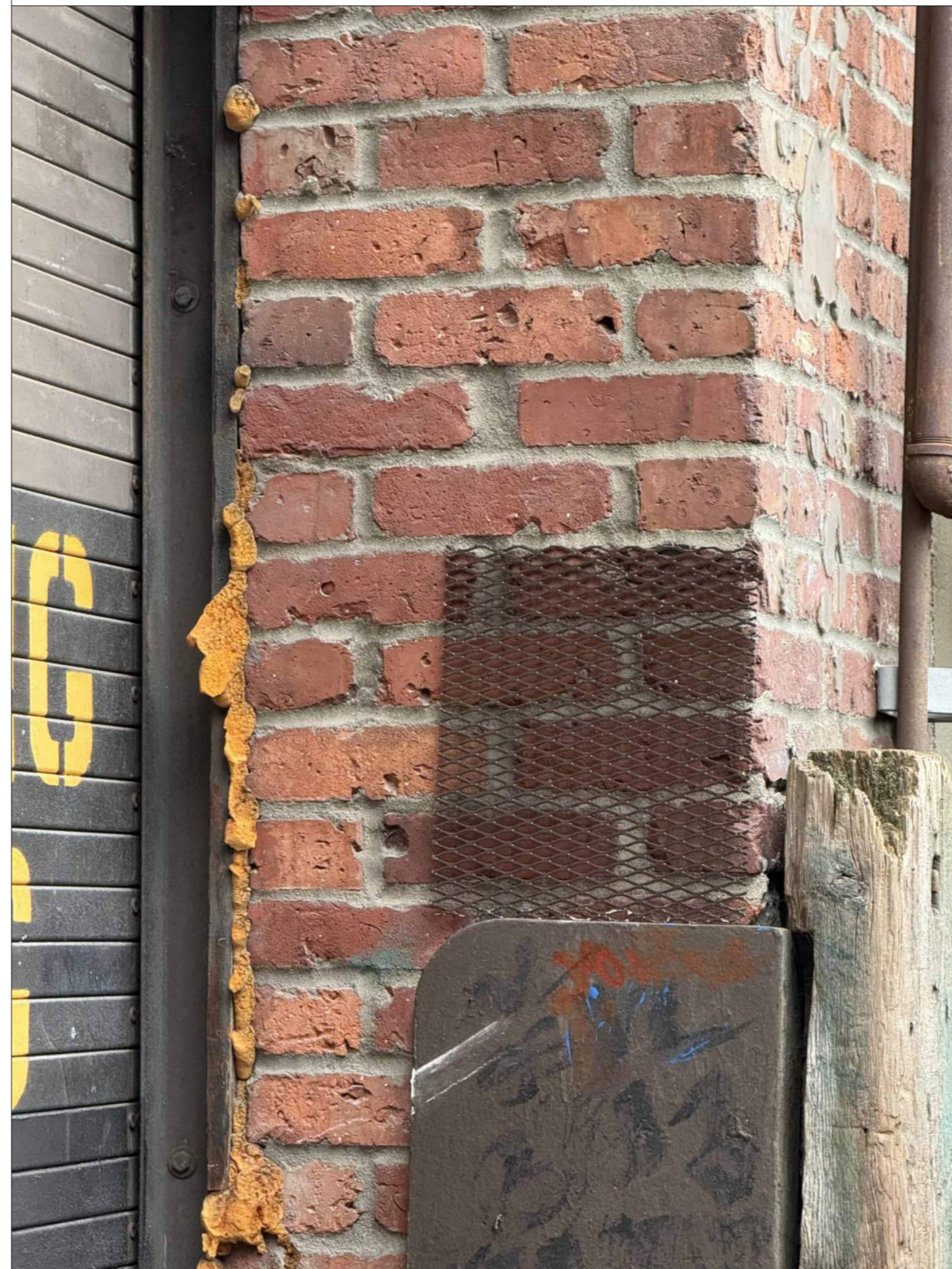
PHOTOGRAPH OF METAL SAMPLE AGAINST BRICK - ENLARGED 1/2x13-15 FLATTENED EXPANDED METAL PAINTED WITH SHER-KEM FAST DRY GLOSS ULTRA DEEP F75C00201
