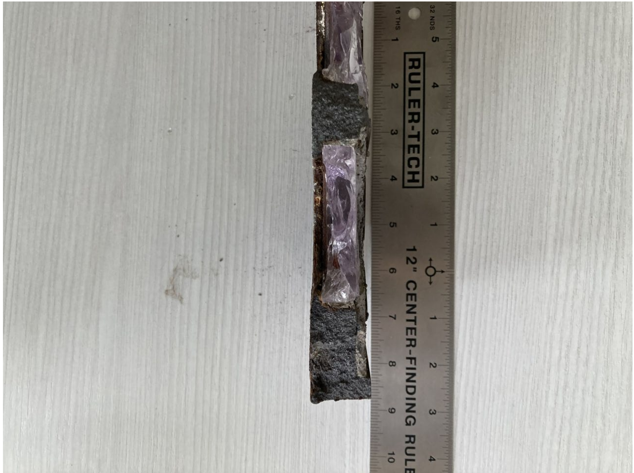
Photo 12: Close up of cross section of a fragment of cast-iron panel
