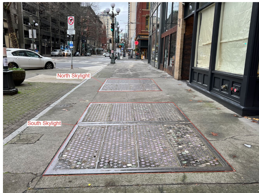
Figure 1: 4 frames, with 4 panels in each frame photo pre-accident condition
