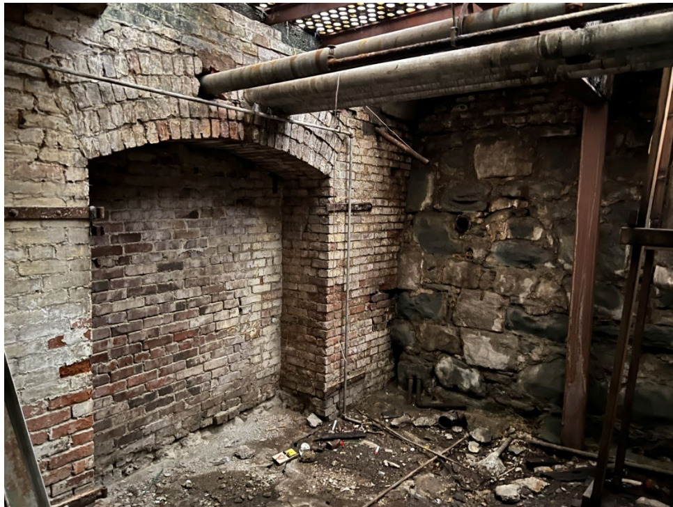
Photo 19: Looking at south end of inside areaway, pre-accident
