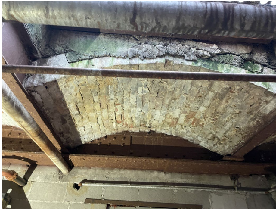
Photo 5: Masonry barrel ceiling looking towards building, post-accident
