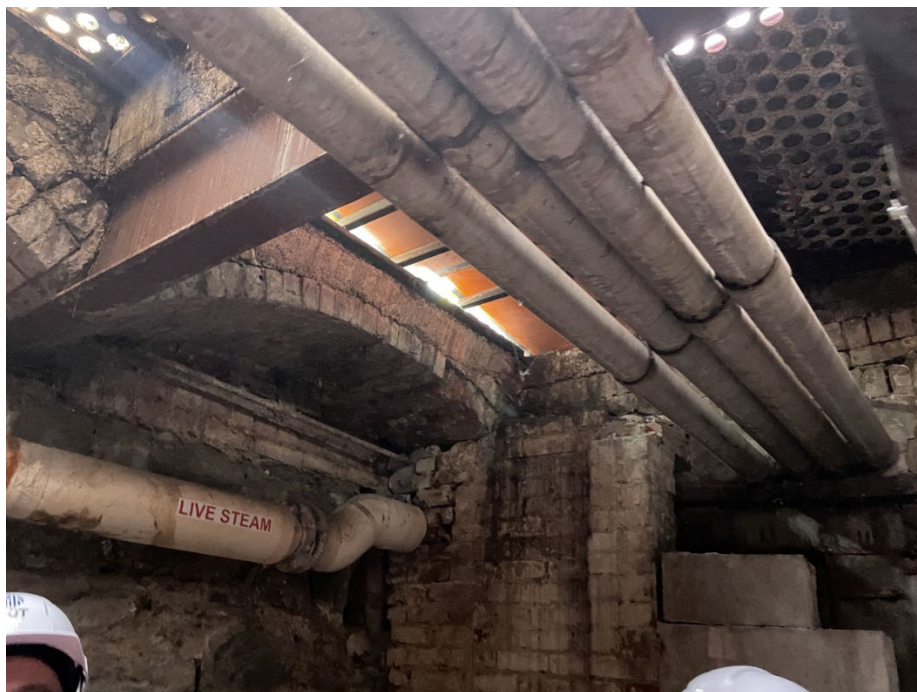
Photo 5: Masonry barrel ceiling looking towards building, post-accident
