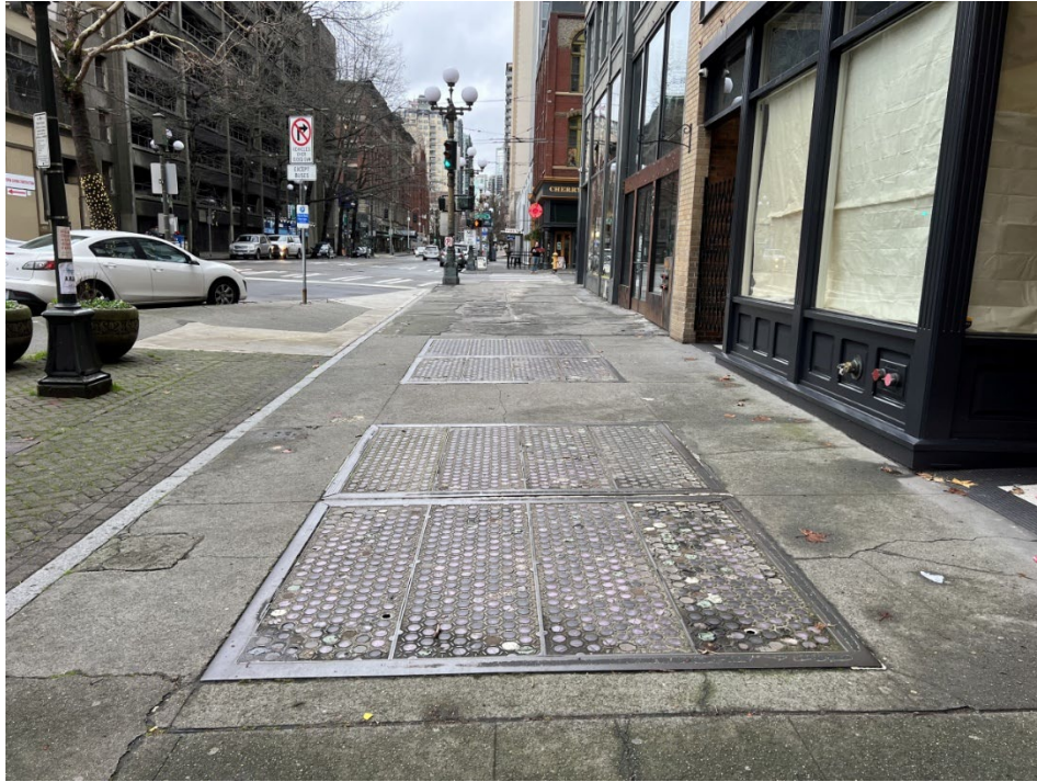
Photo 18: Looking north, top of frame and panel pre-accident
