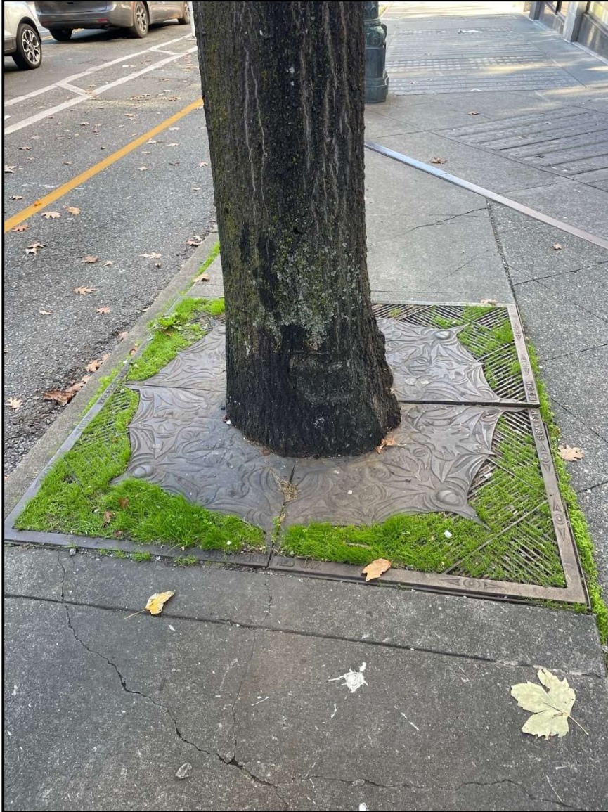
Photo 11. Street tree near Prefontaine Place. Tree is being girdled by tree grate and requires management as soon as possible.
