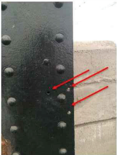
Figure 1. Typ. example of holes to be patched (photo of C B1)
