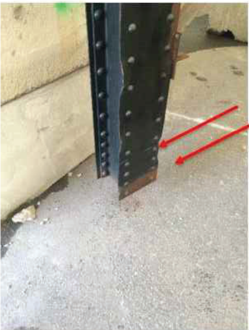
Figure 3: Typ. example of warped Column Base (photo of C B1)
