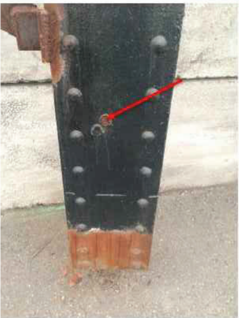
Figure 2: Typ. example of raised rust patches to be repaired (photo of C B2)
