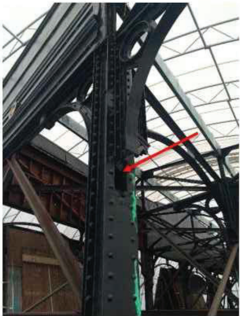
Figure 3: Typ. example of missing corbel (photo of C B8)
