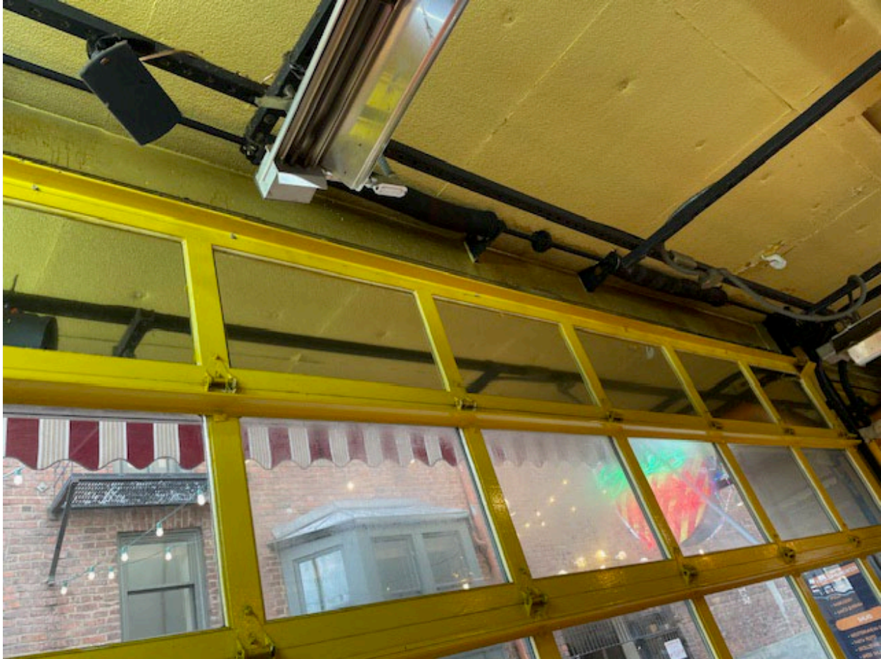
Existing roll up door track close up west facing right side
