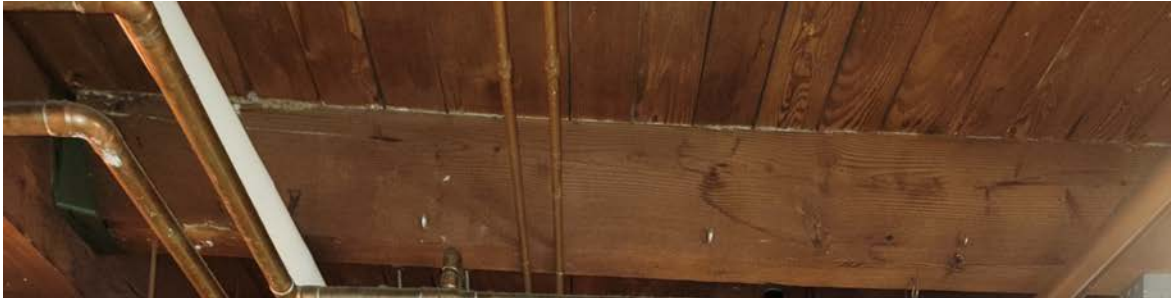
Eyehooks installed in beam
