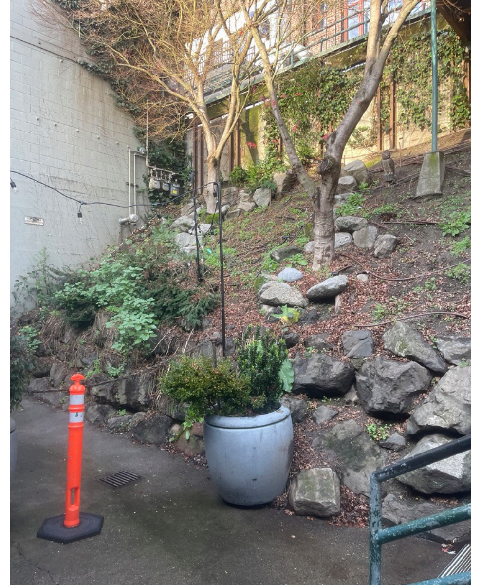
Courtyard: View of East Slope
