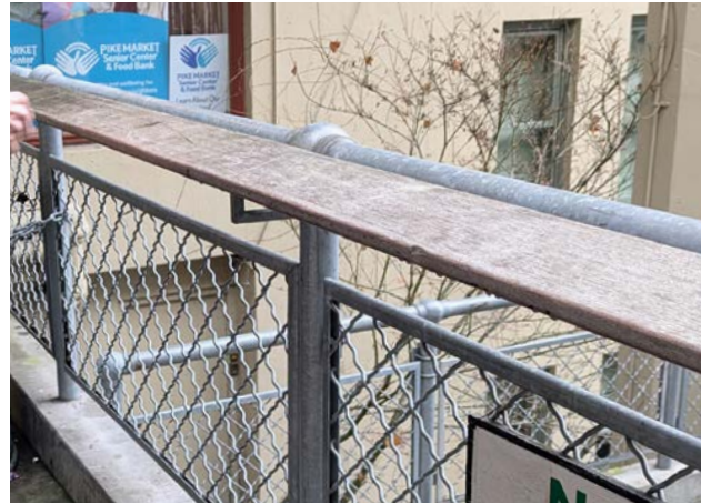
Existing lean rail at Hillclimb.
