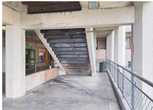
Existing condition under stairs.
