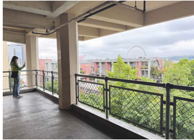
Existing condition at railings.
